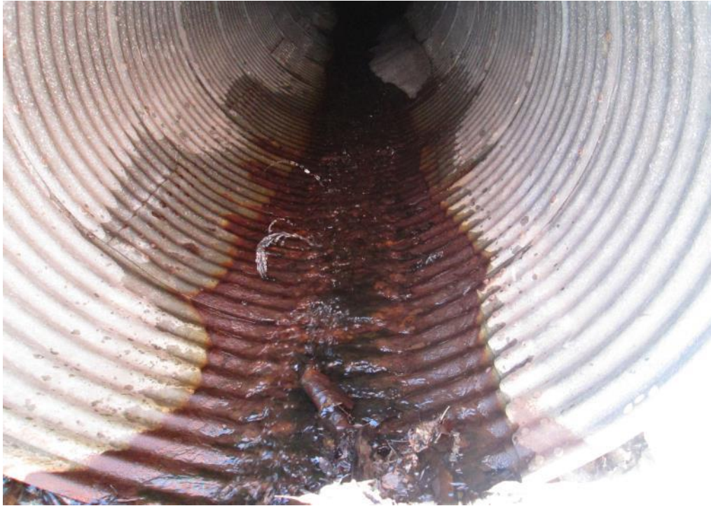
Photo 11: Deterioration of culvert at inlet
