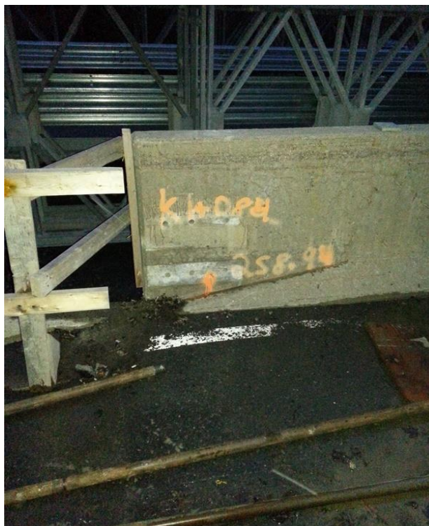
Photo 8: Temporary benchmark on concrete barrier
