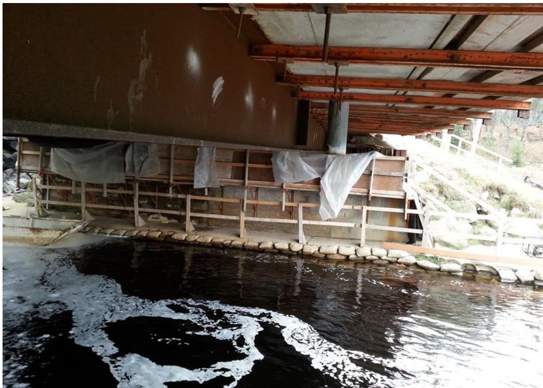
Photo 6: Temporary support under bridge
