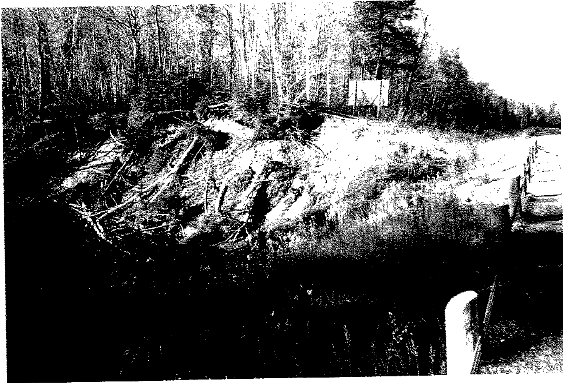
PICTURE 1 Showing Erosion of Road Bank and adjacent hill - looking North-west.
