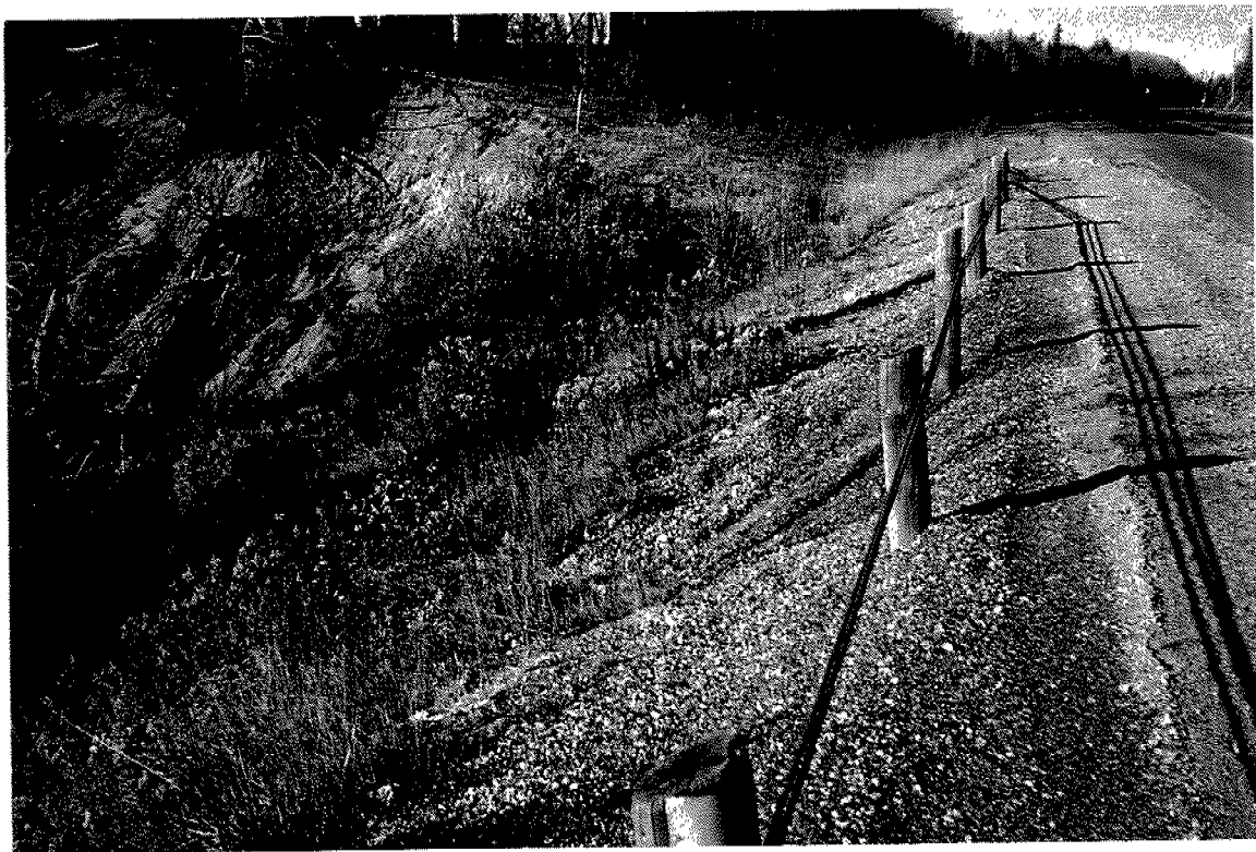
PICTURE 2 Showing Erosion of bank at the north-west corner of site - looking North-west
