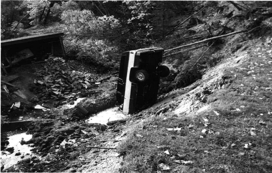
Photo 5 – Note Groundwater and effluent at base of slump.
