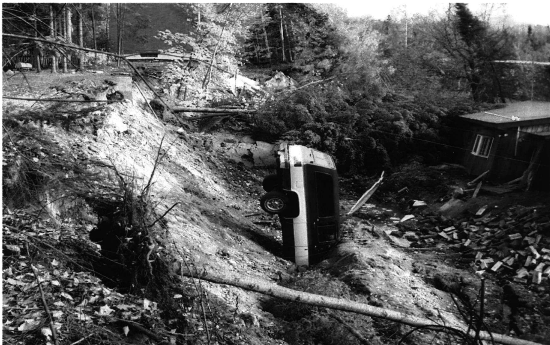
Photo 2 – Sectional View of Main Scarp. Note house on right within slump area.
