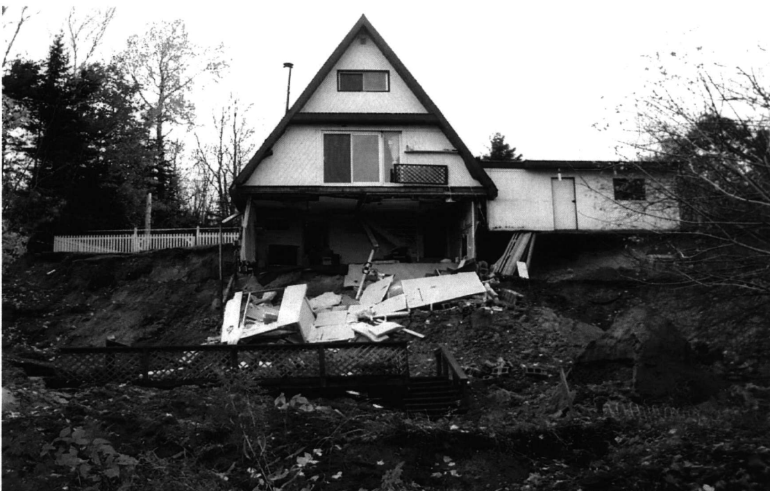
Photo 4 – Home severally undermined and on verge of tumbling into slump area.
