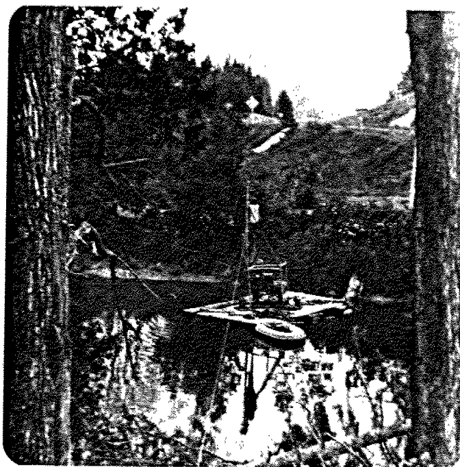
Figure 4 East Bank of River Drilling Rig on Borehole 6
