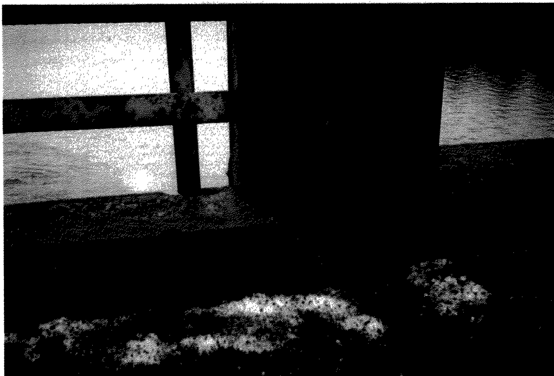
PHOTOGRAPH 10 Note deck settlement on east side of bridge above Pier 2.
