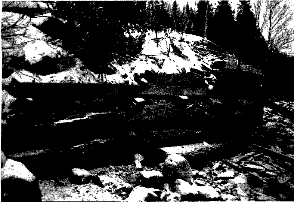
TIMBER CRIB, EAST APPROACH FILL
