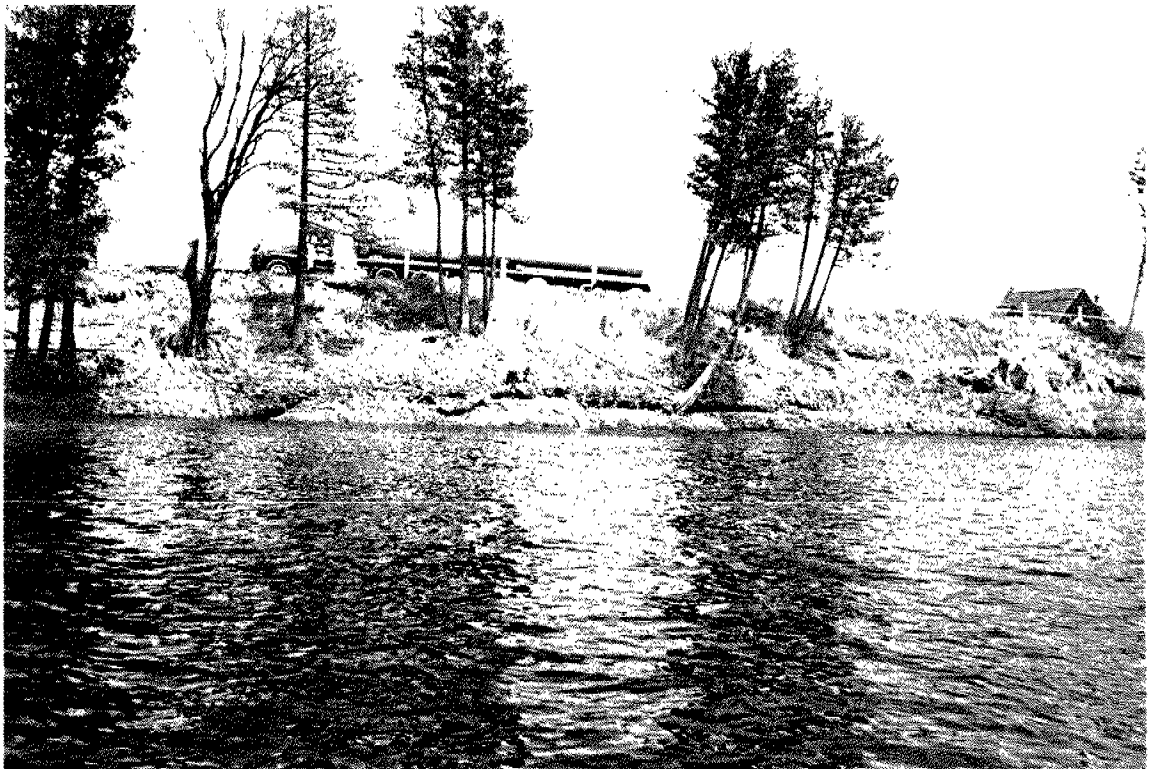
PLATE I SHOWING TOE EROSION AND FORMATION OF BACK SCARPS
