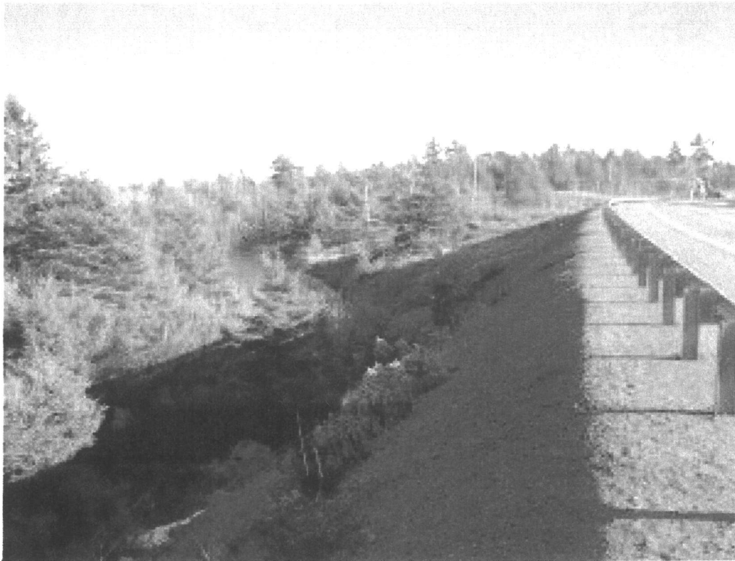
PHOTOGRAPH 7: View looking south Sta. 15+450 from east shoulder Highway 69. Rockfill embankment across east end of Ink Lake. Bedrock exposed, south side of lake and rock cut east side of Highway 69 to south.
