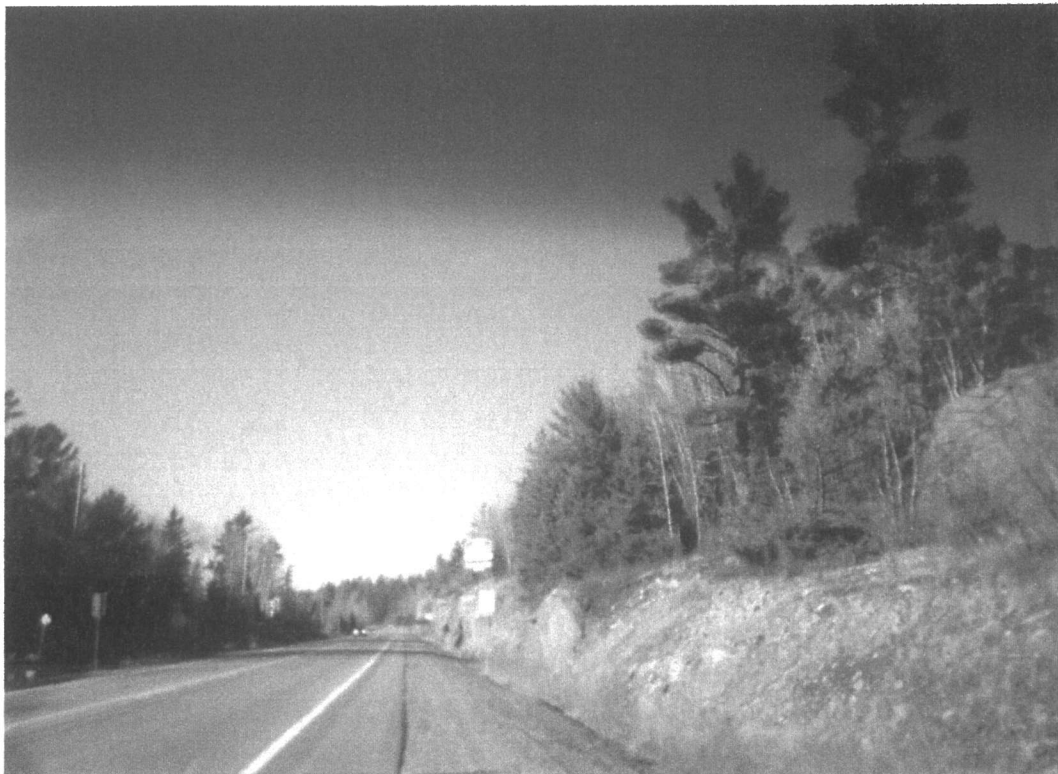
PHOTOGRAPH 15: View looking north at Sta. 17+900 from east shoulder of Highway 69. Till cover over bedrock on steep right (east) slope. Bedrock cut right side in distance.
