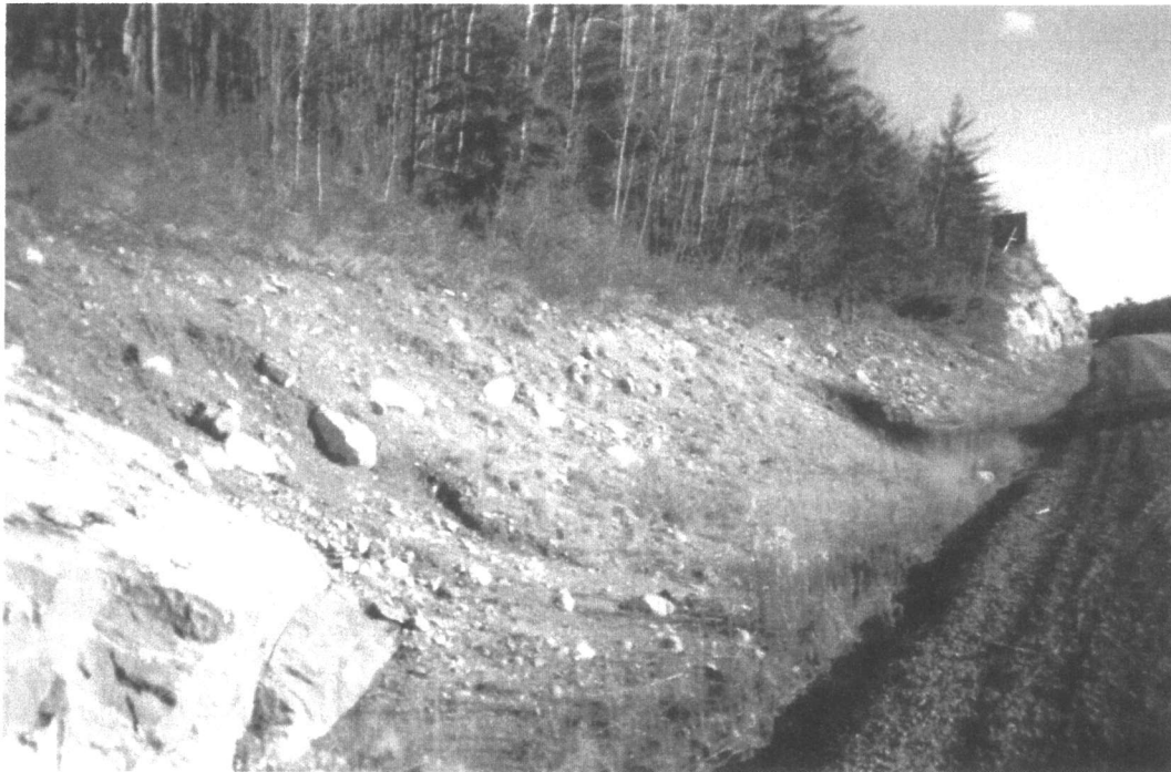
PHOTOGRAPH 17: View looking south at Sta. 19+250 from east shoulder of Highway 69 (at west edge of corridor). Bedrock cut left (east) foreground, then till cover over bedrock. Rock cut (5 – 6 m) at Sta. 19+000 in distance.
