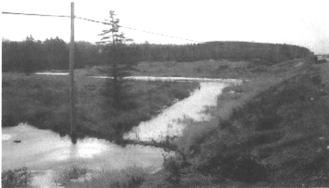
PHOTOGRAPH 29: View looking south Sta. 27+750, from east shoulder of Highway 69 along east side of corridor. Water course at toe of fill with beaver dam in foreground. Outwash plain (glaciofluvial) with bedrock knob outcrop at tree-line.
