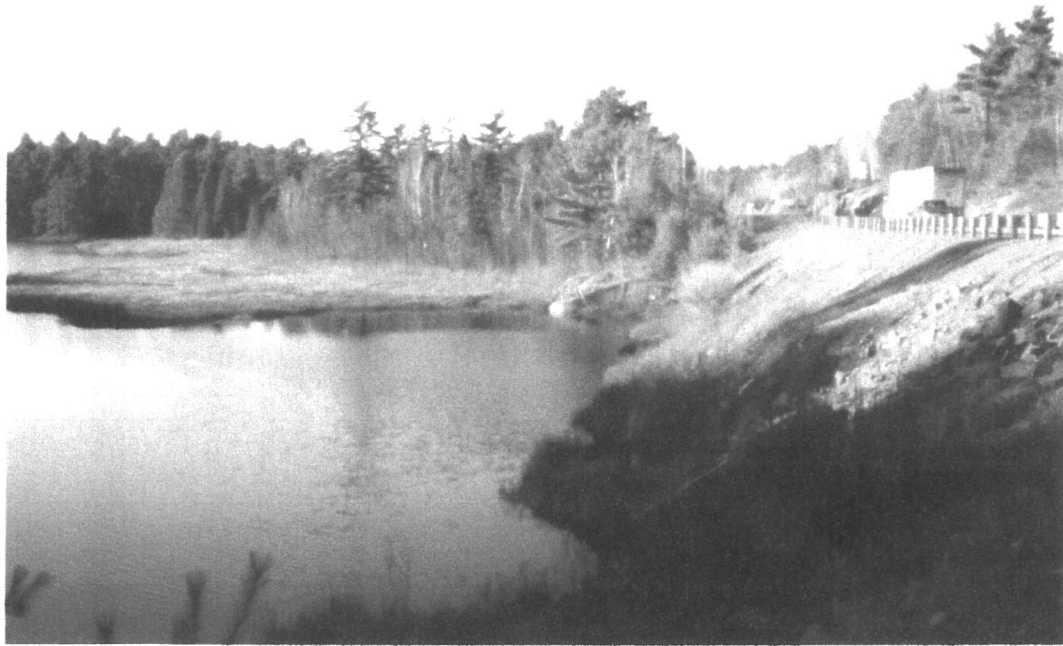
PHOTOGRAPH 11: View looking north Sta. 17+550 from west side of Highway 69 rockfill embankment crossing Murdock River. Bedrock outcrops south bank and swamp north side.
