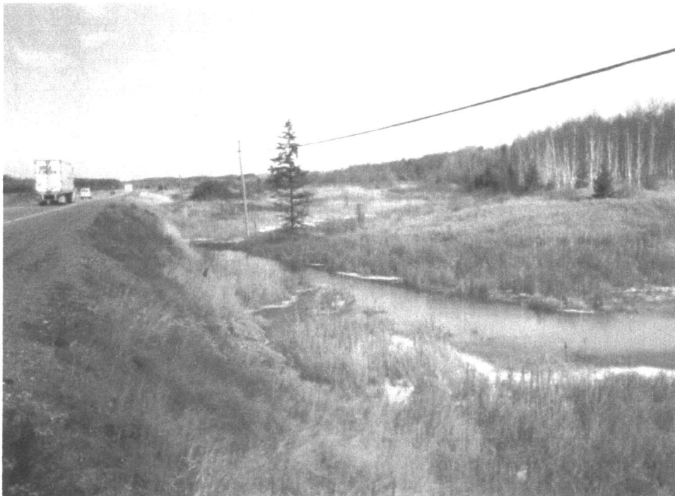
PHOTOGRAPH 28: View looking north Sta. 27+650 from east shoulder of Highway 69 along east side of corridor (outwash plain-glaciofluvial). Water course on east half of corridor. Signs of embankment movement. Gabion baskets at timber culvert. Beaver dam visible at hydro pole.
