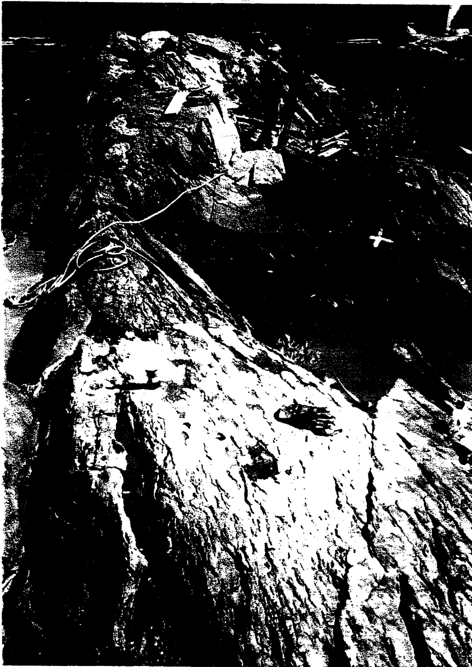
Plate 10: Looking east at new bridge centre pier location. Note jagged character of exposed rock surface.
