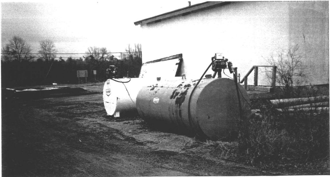
Plate 5: AST diesel tanks adjacent the salt shed.
