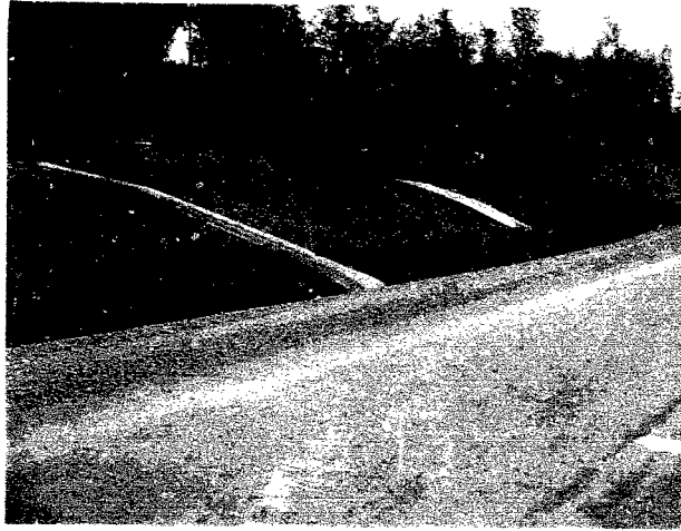
-Water flowing from concrete drain as it did in April 1968. No water in concrete drain in background which has cracked due to removal of soil support beneath it by erosion of springs.
