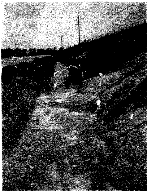
-Water in roadside ditch; evidence of springs in slope.
