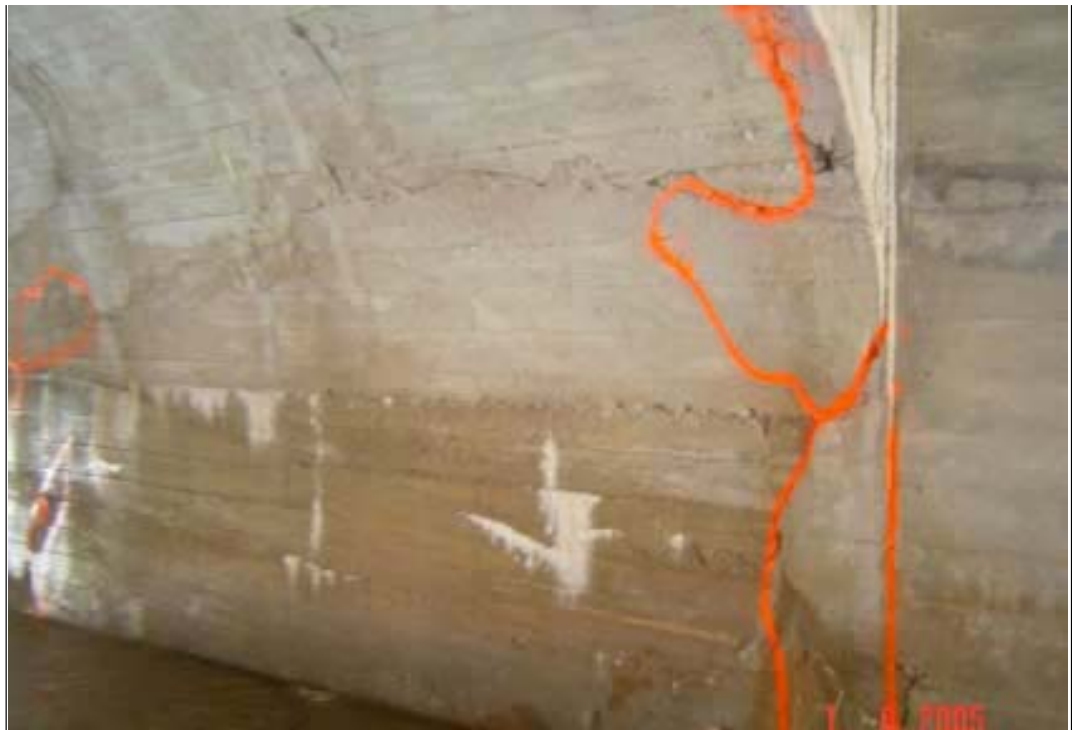
Photo 13: Delaminations and cracks in arch, east wall.
