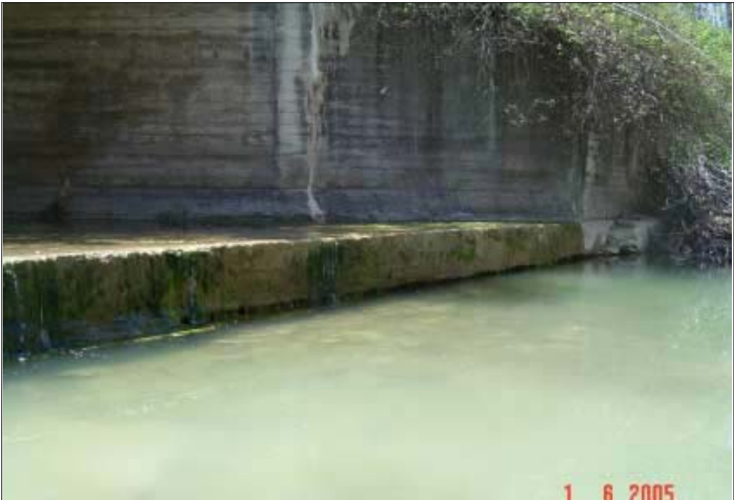
Photo 7: Undermining at outlet.
