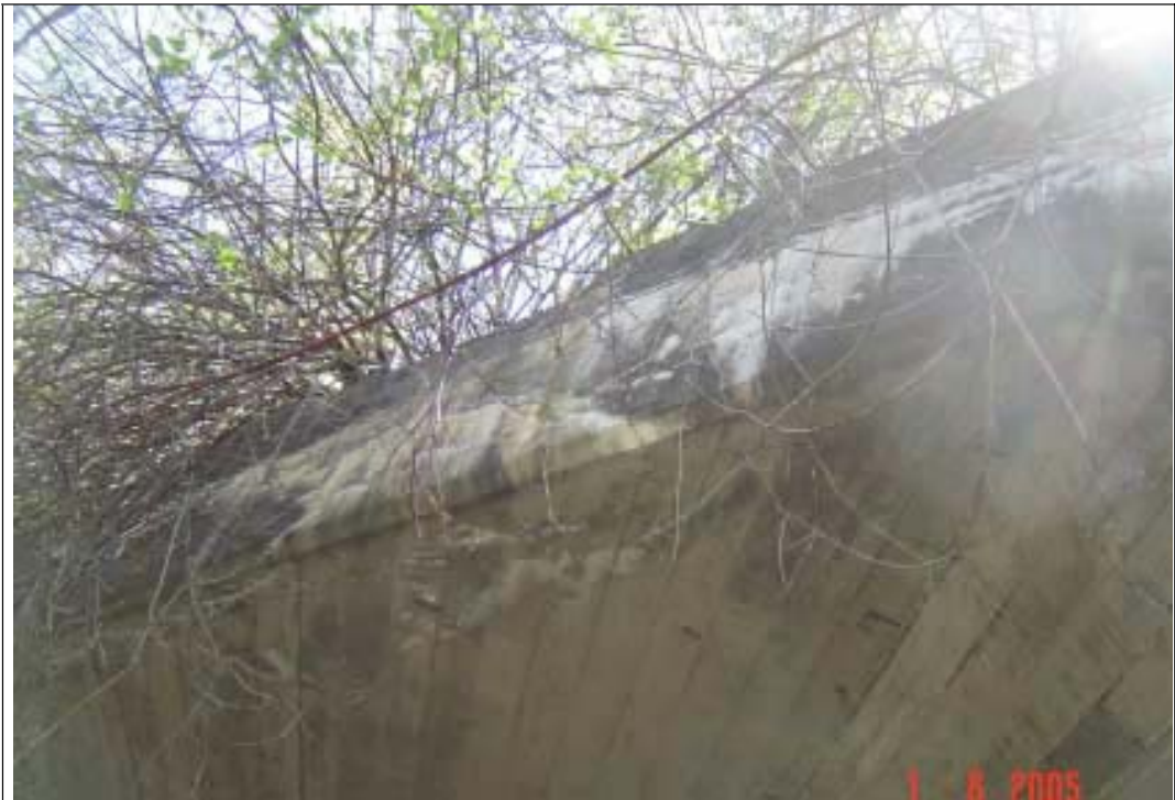
Photo 8: Cracking and leaching at north headwall.
