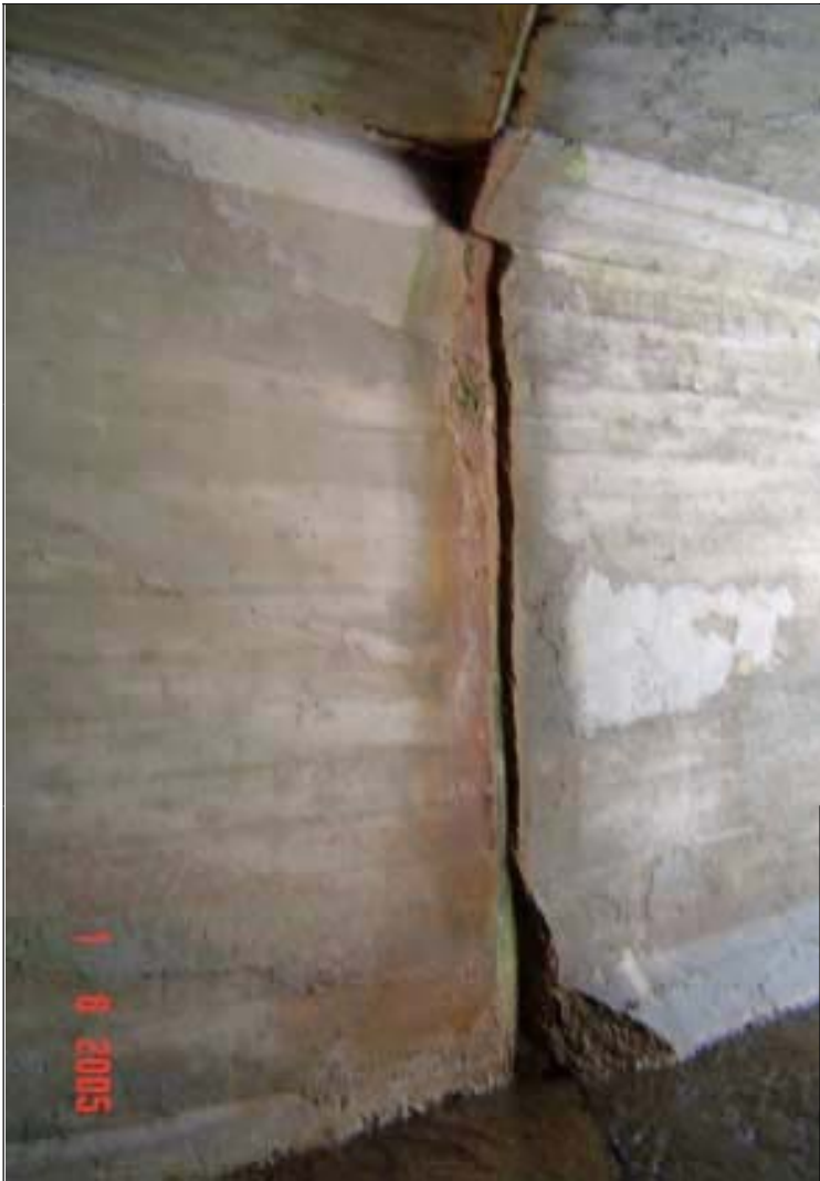
Photo 9: Typical construction joint at south extension.
