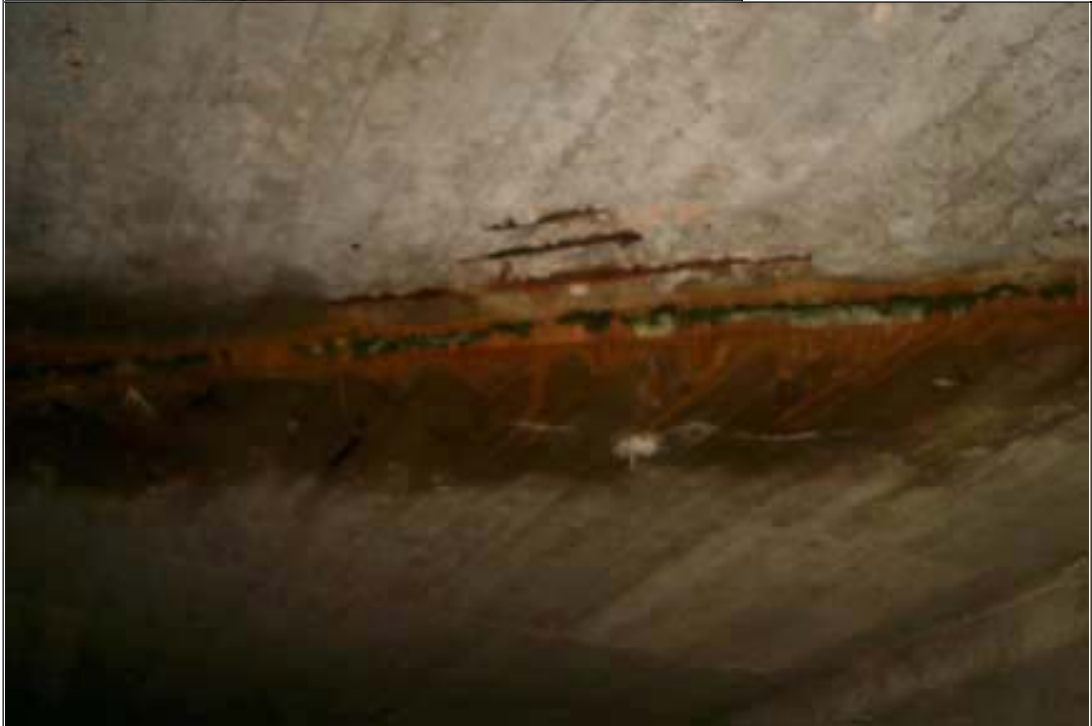
Photo 10: Delamination and wetness at soffit construction joint (south extension).
