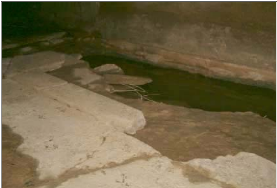
Photo 14: Floor slab failure at arch, looking southwest.
