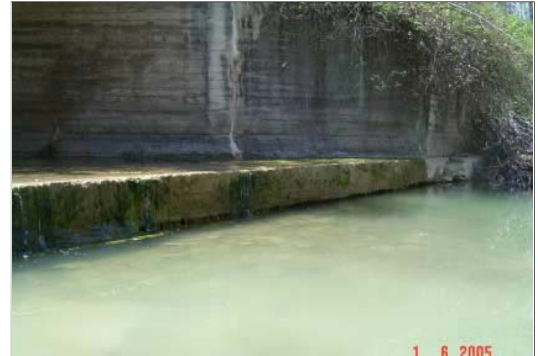
Photo 7: Undermining at outlet.
