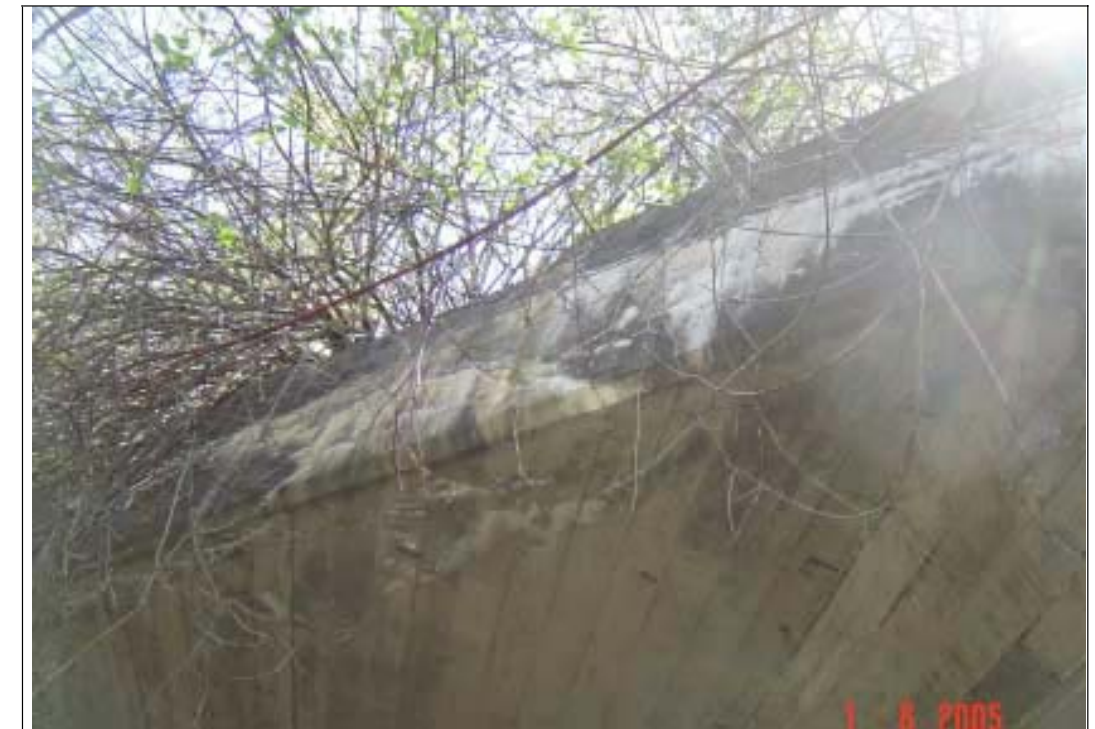
Photo 8: Cracking and leaching at north headwall.
