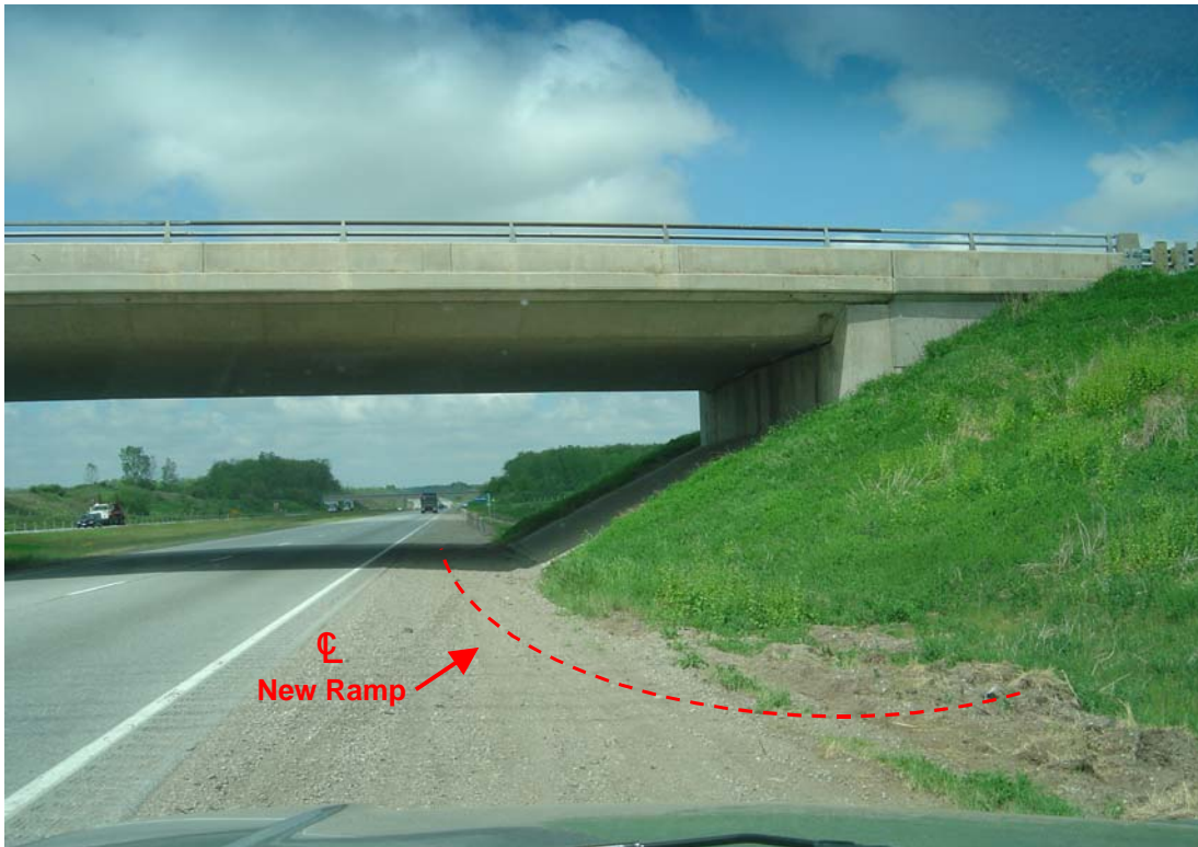
Photograph 1: Looking west along Highway 403 at north abutment of Oak Park Road structure. Abutment foreslope will be removed to allow construction of new on-ramp under structure.
