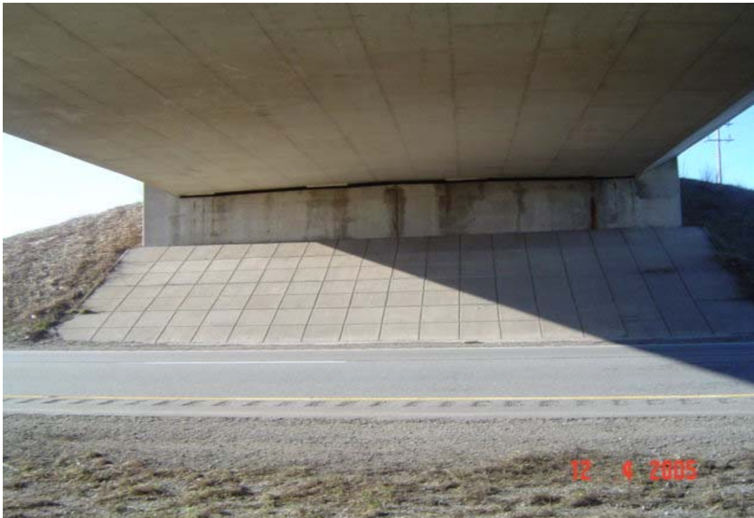
Photograph 3: Looking north from median of Highway 403 at foreslope of Oak Park Road north abutment. Note slope protection with concrete slabs and water seepage below deck on vertical abutment wall.
