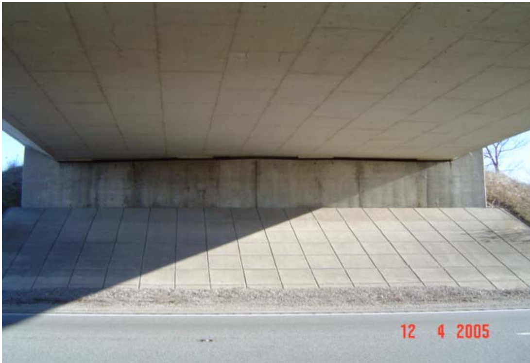
Photograph 4: Looking south from median of Highway 403 at foreslope of Oak Park Road south abutment. Note slope protection with concrete slabs.
