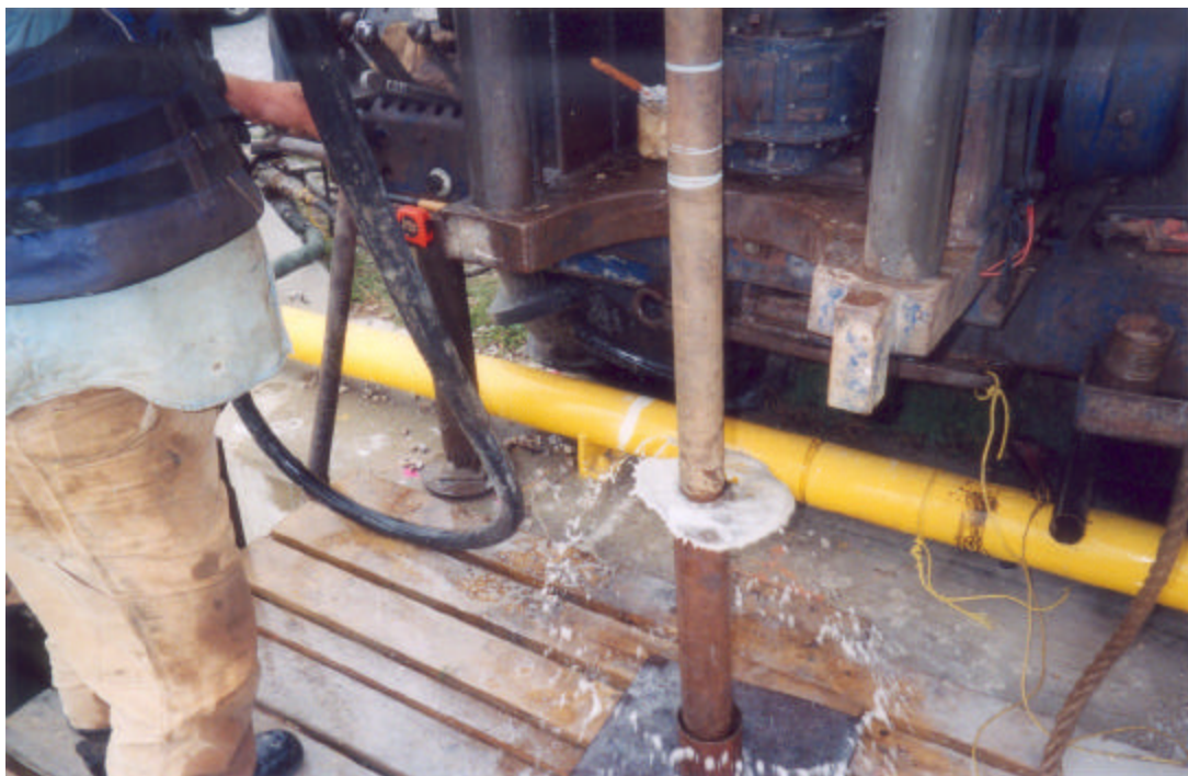
Photo 2: Washboring through drill casing.
