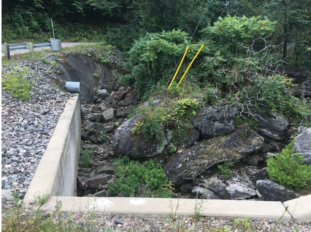
Photo 1. Looking upstream from culvert inlet, note erosion at north wingwall
