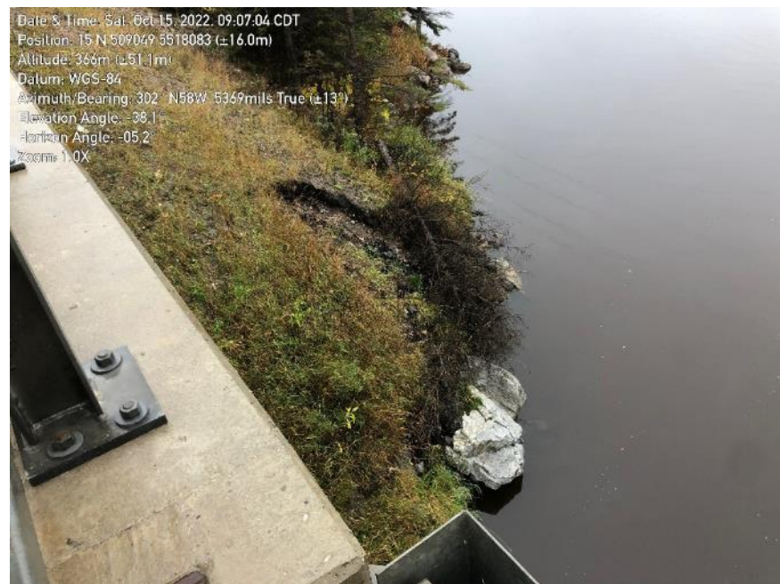
Photo 6: Looking down at toe erosion at northwest corner of bridge (October 2022)
