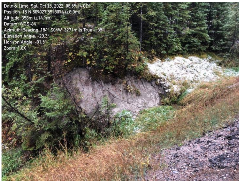
Photo 8: Looking south towards slide beyond ditch at southwest corner of bridge (October 2022)
