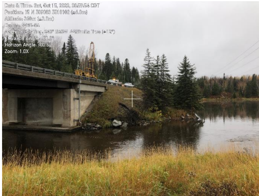
Photo 5: Looking southwest at northwest corner of bridge (embankment toe erosion) (October 2022)
