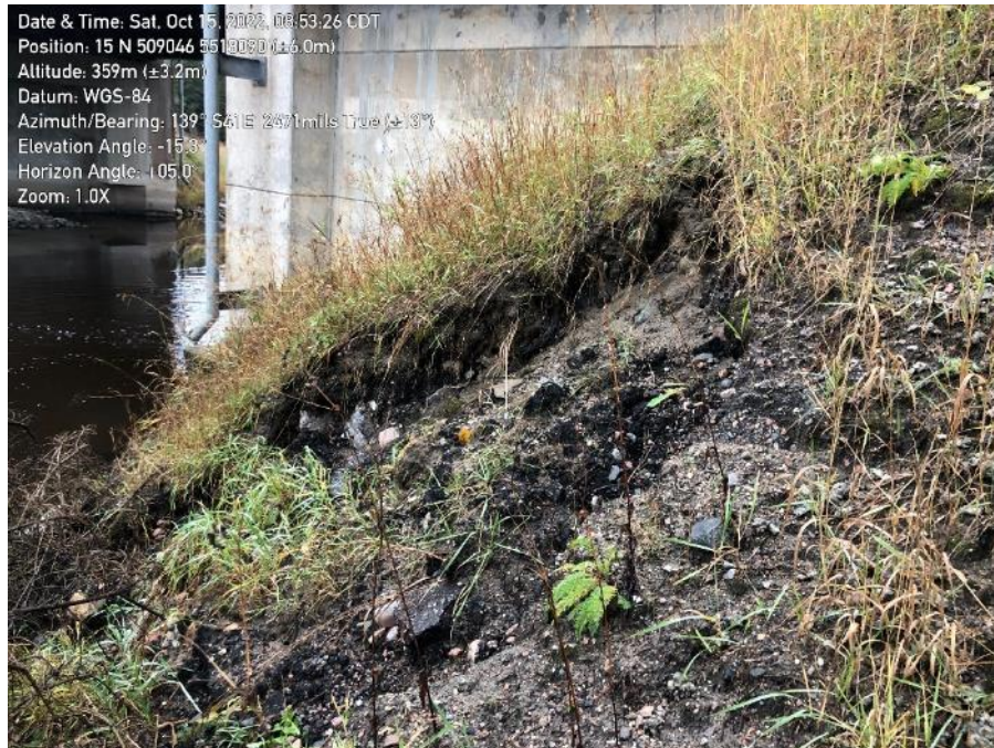
Photo 7: Looking southeast at toe erosion at northwest corner of bridge (October 2022)
