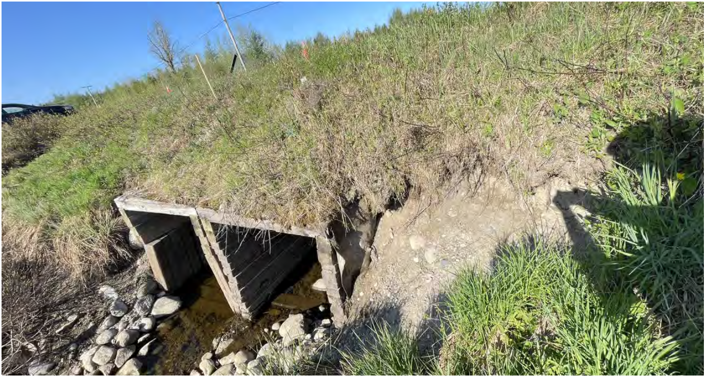
Photograph #13 – Localized erosion at the north edge of the culvert outlet at the east embankment toe. (May 2023)
