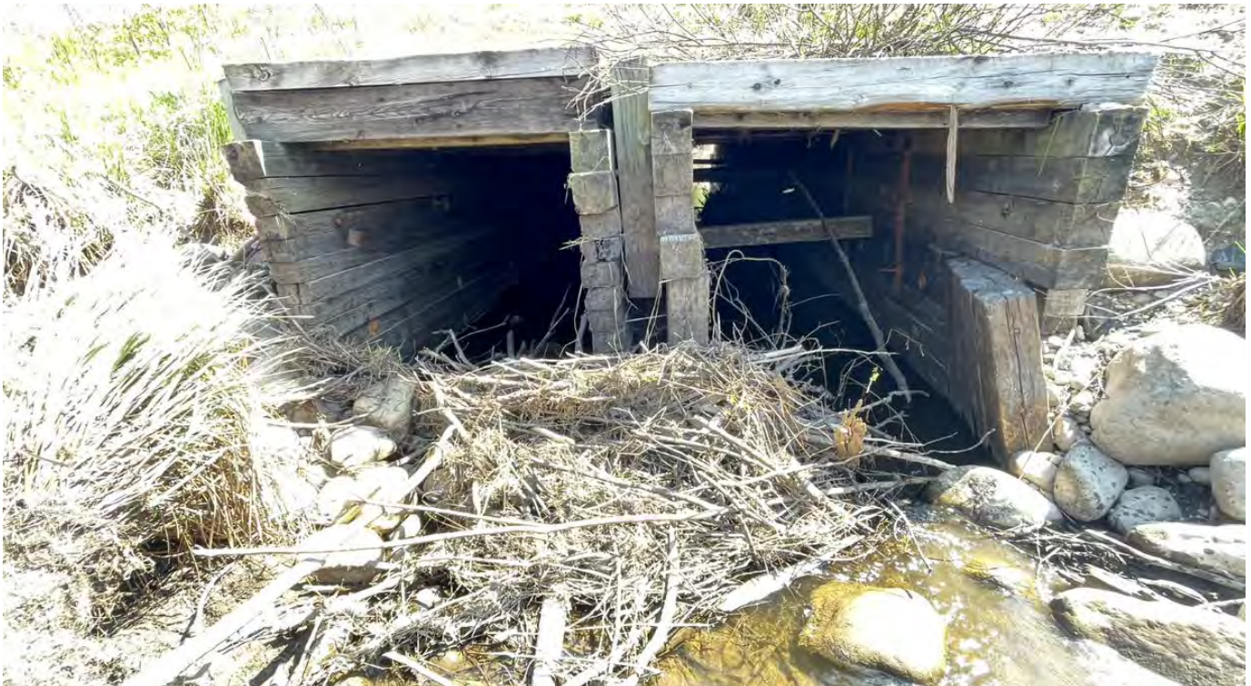
Photograph #2 – Highway 579 culvert inlet with debris at the west embankment toe. (May 2023)
