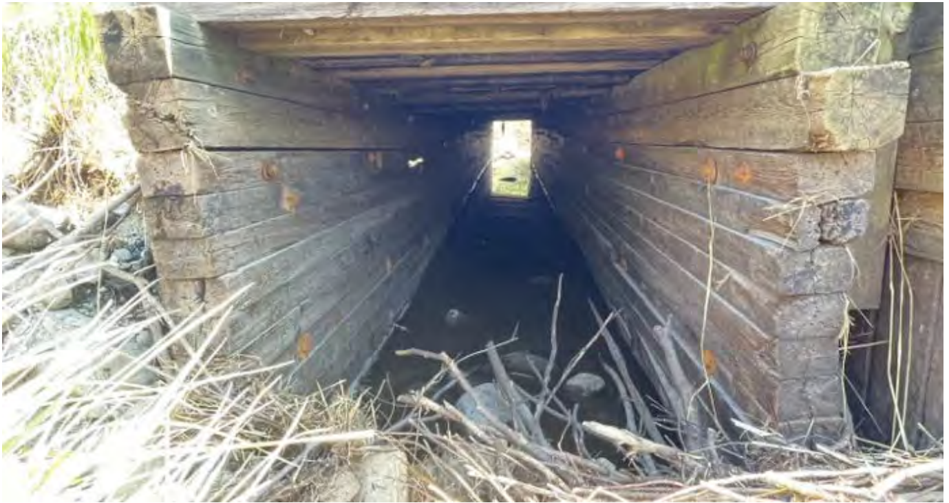
Photograph #5 – Highway 579 culvert inlet at the west embankment toe, north cell. (May 2023)
