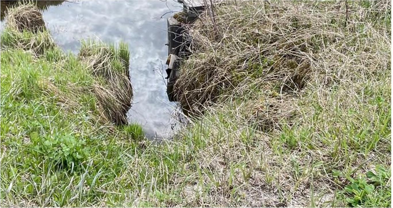
**Photograph #7** – Erosion along the north edge of the culvert near the inlet, facing east. (May 2023)
