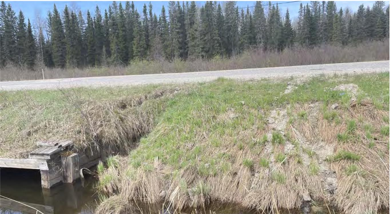
**Photograph #8** – Erosion along the north edge of the culvert near the inlet, facing west. (May 2023)
