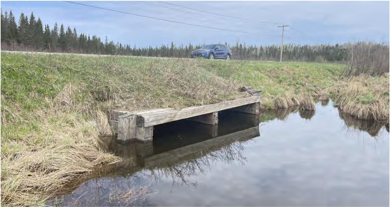
**Photograph #1** – Culvert inlet at the east embankment toe, surrounded by a ponded water, facing west. (May 2023)
