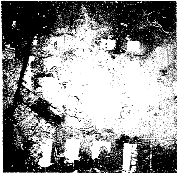
Boiling at base of excavation
