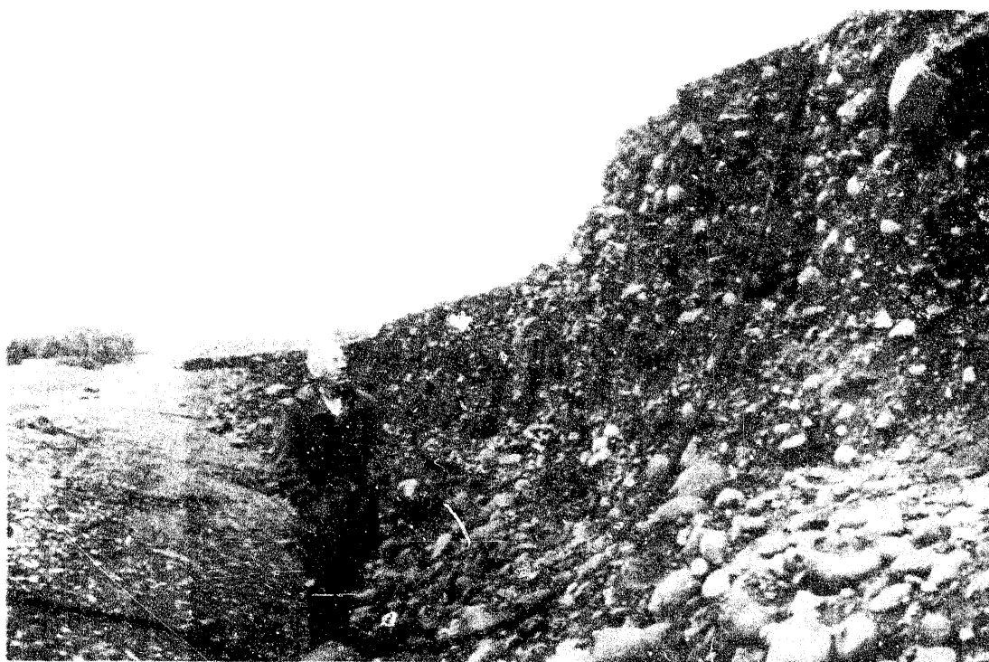
FIG. 4: VIEW OF EXPOSED PORTION OF EMBANKMENT AFTER FAILURE
