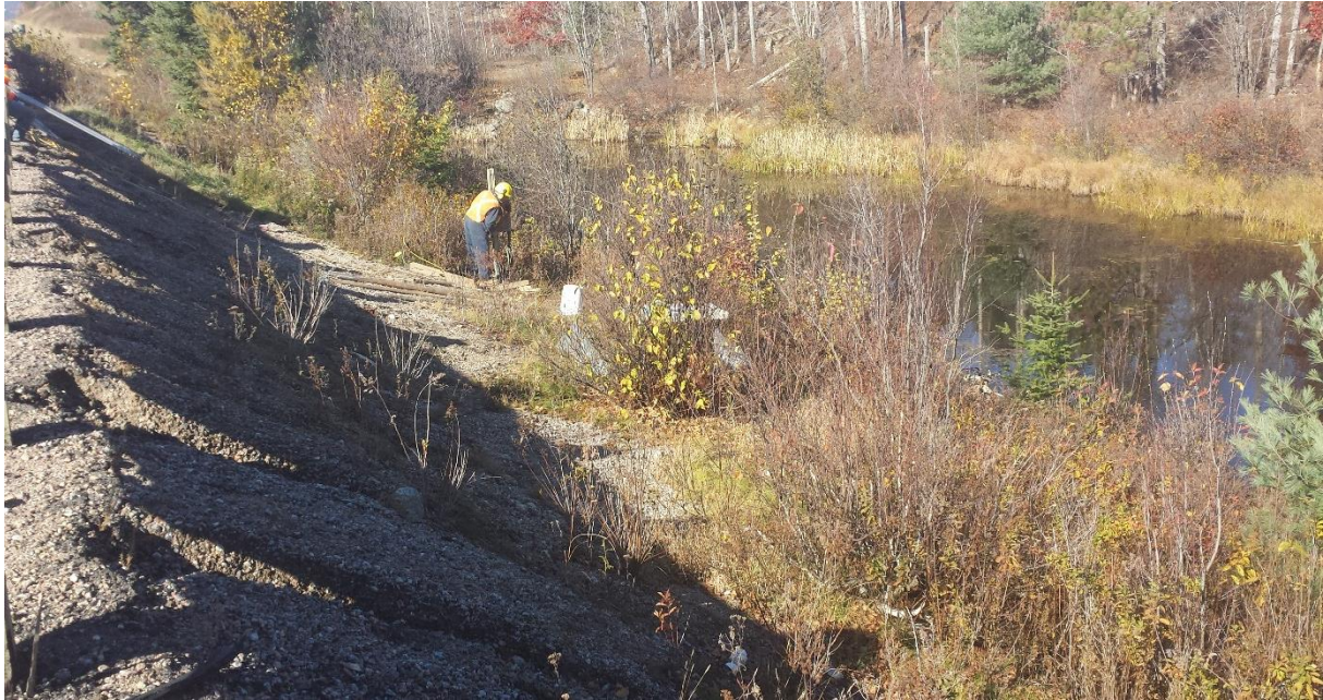
Figure 7: Erosion of north embankment granular cover
