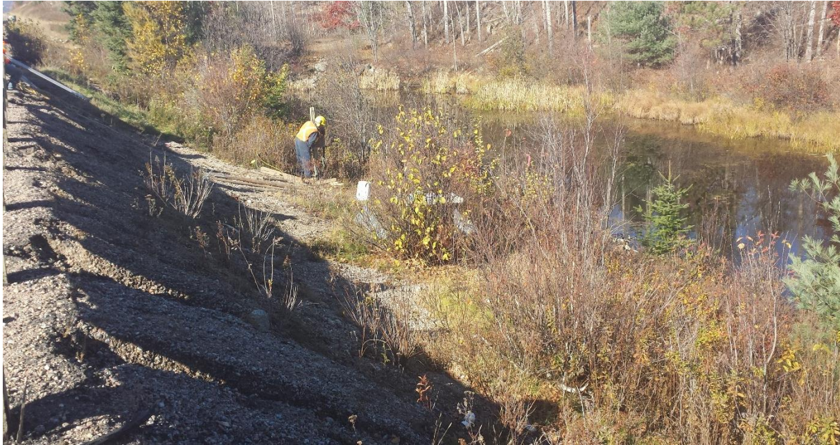
Figure 7: Erosion of north embankment granular cover
