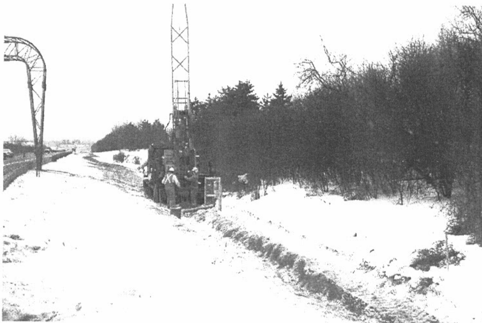
Photo No. 2: Drilling BH10-1.
