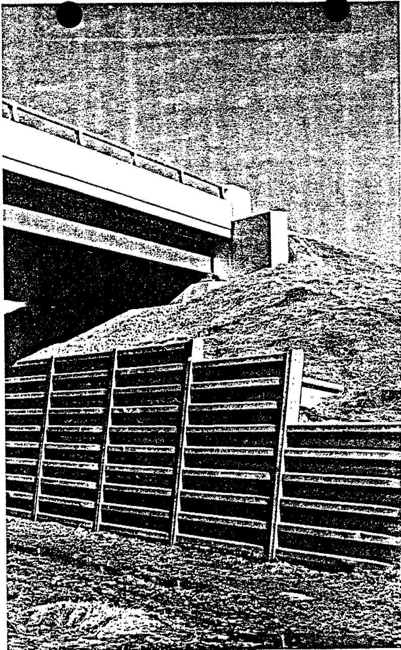
Figure 1 Bin-type Steel Retaining Wall
