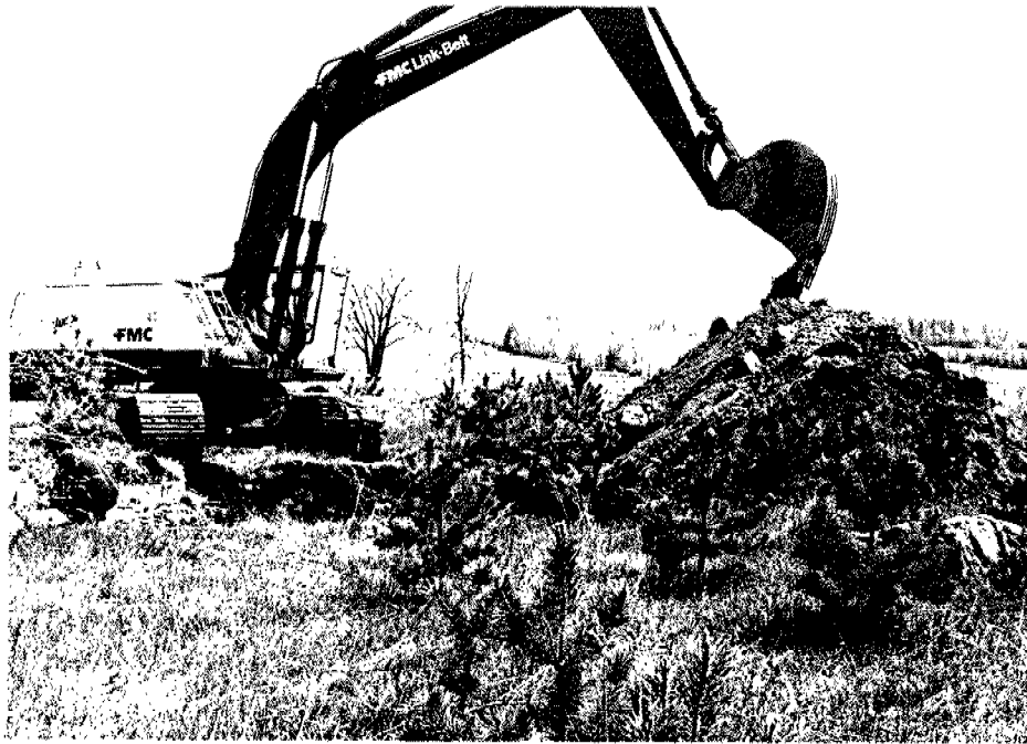
PHOTO 1 - Stockpile of soil consisting of a heterogeneous mixture of silt, sand, gravel, cobbles and boulders (glacial till) excavated at test pit #1
