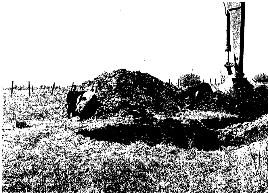
PHOTO 4 - Enormous boulder sizes are not uncommon in the till deposit. The photo illustrates a 1.5 m boulder.
