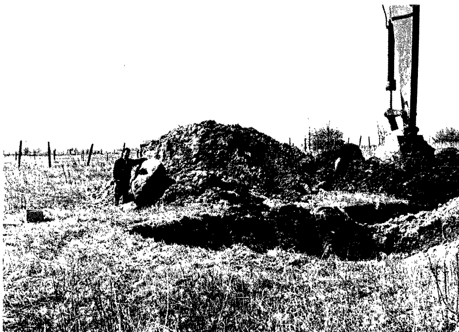
PHOTO 4 - Enormous boulder sizes are not uncommon in the till deposit. The photo illustrates a 1.5 m boulder.
