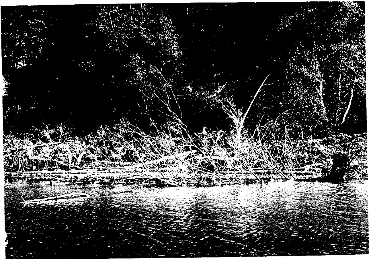
PLATE No. 11 TOE FAILURE AT STATION 271
