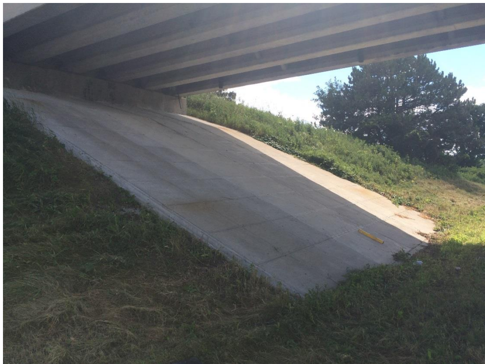
Figure 10: South abutment foreslope slope pavers
