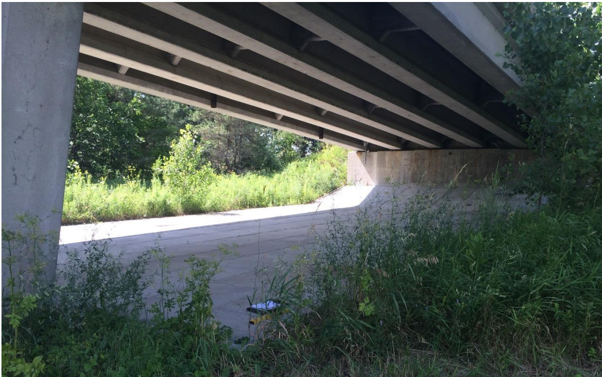
Figure 6: North abutment foreslope slope pavers
