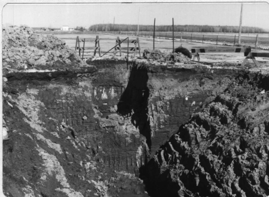
PHOTOGRAPH 1 VIEW OF TEST TRENCH LOOKING EAST SHORTLY AFTER EXCAVATION ON MARCH 12, 1974. DEPTH OF VERTICAL SIDED SECTION - APPROX. 11 FT. DEPTH OF SLOPING SIDED SECTION - APPROX. 16 FT.
