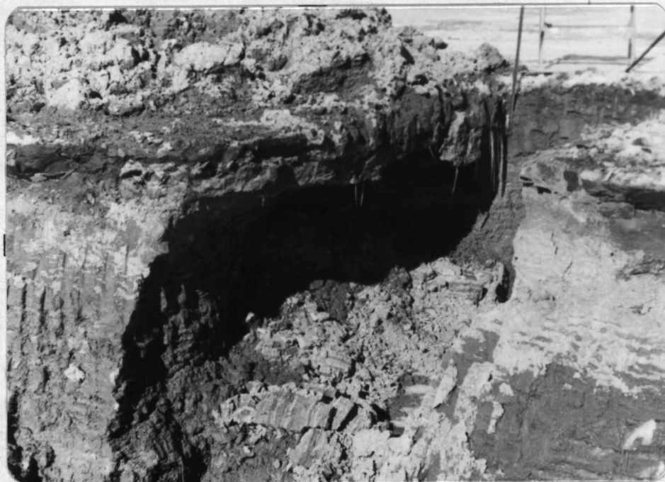
PHOTOGRAPH 4 DETAIL OF FAILURE ON THE NORTH VERTICAL WALL, MARCH 15, 1974.
