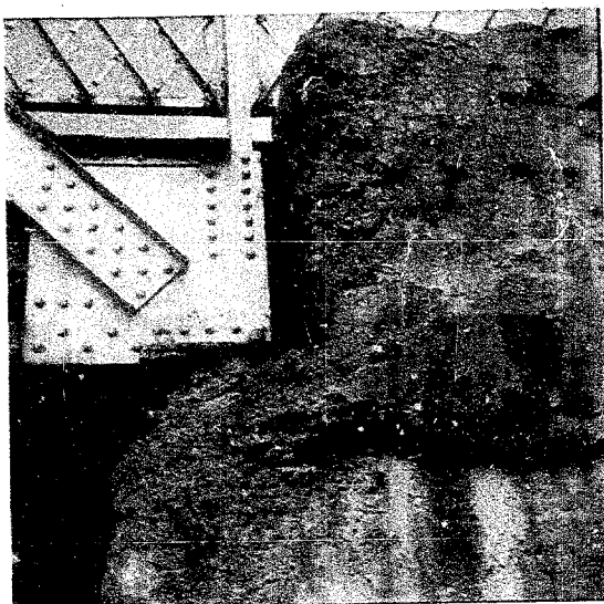
Photo of left corner of existing south abutment showing deterioration of concrete around bearing plate and anchor bolts.
