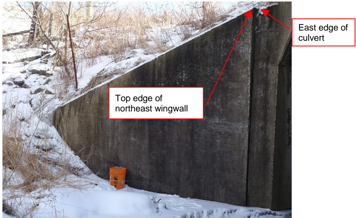
Photograph 5: Rotation of northeast wingwall (2017/01/17)
