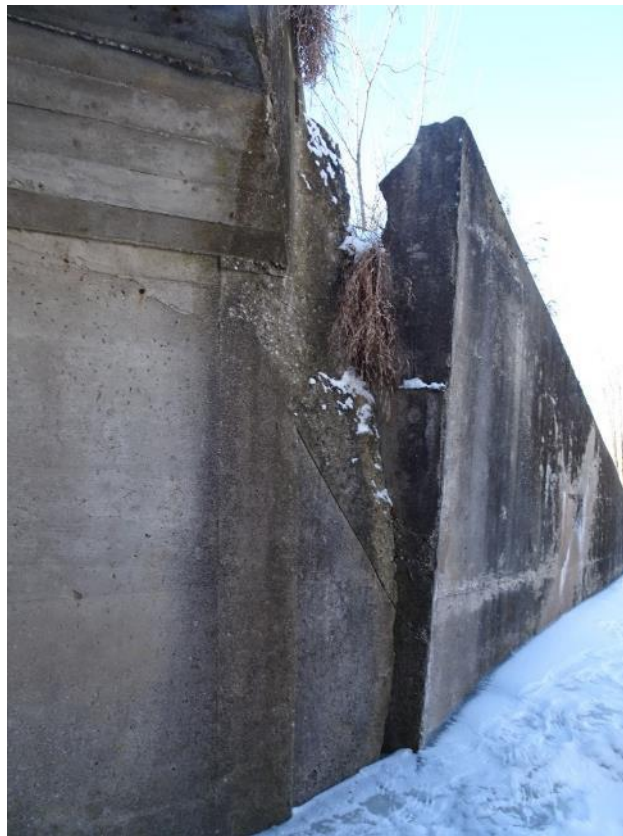
Photograph 4: Rotation of northwest wingwall (2018/02/16)
