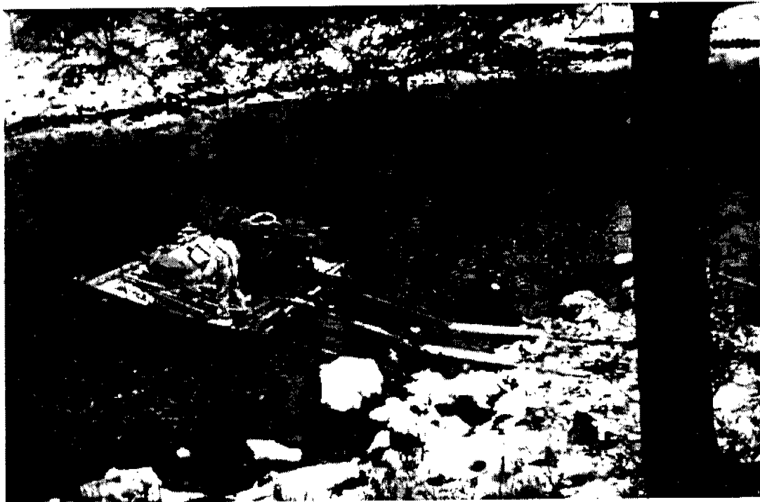
PHOTOGRAPH 4 Raft and drill rig (D-25) used to advance boreholes for piers.
