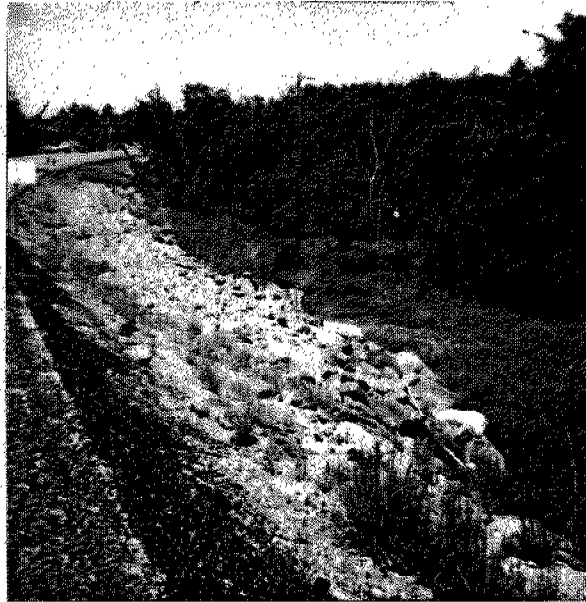
Site 2 - looking South at east side - rockfill berm added.
