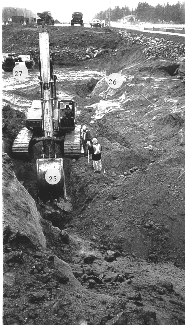
Photo 8: November 11, 1998. View of backhoe digging to expose bedrock ledge at east end of abutment area for northbound structure looking north from shoulder area showing:
