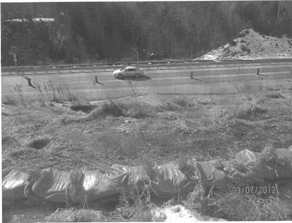
Figure 5: Sand bags placed after the instability took place.
