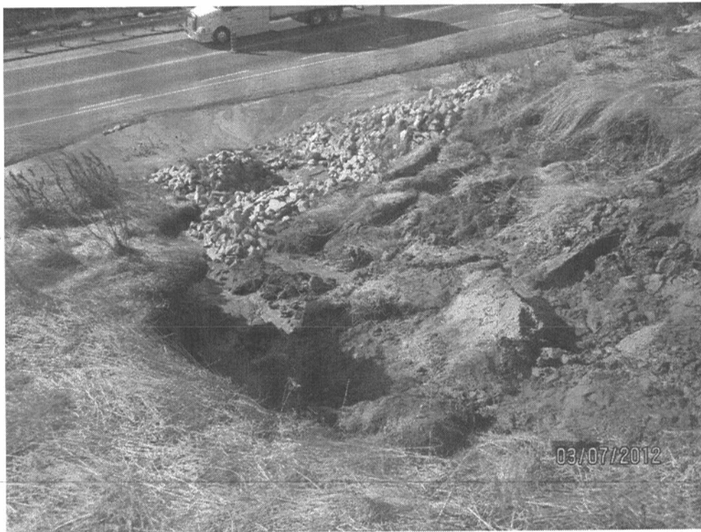
Figure 2: Slope Instability from the crest, towards south.
