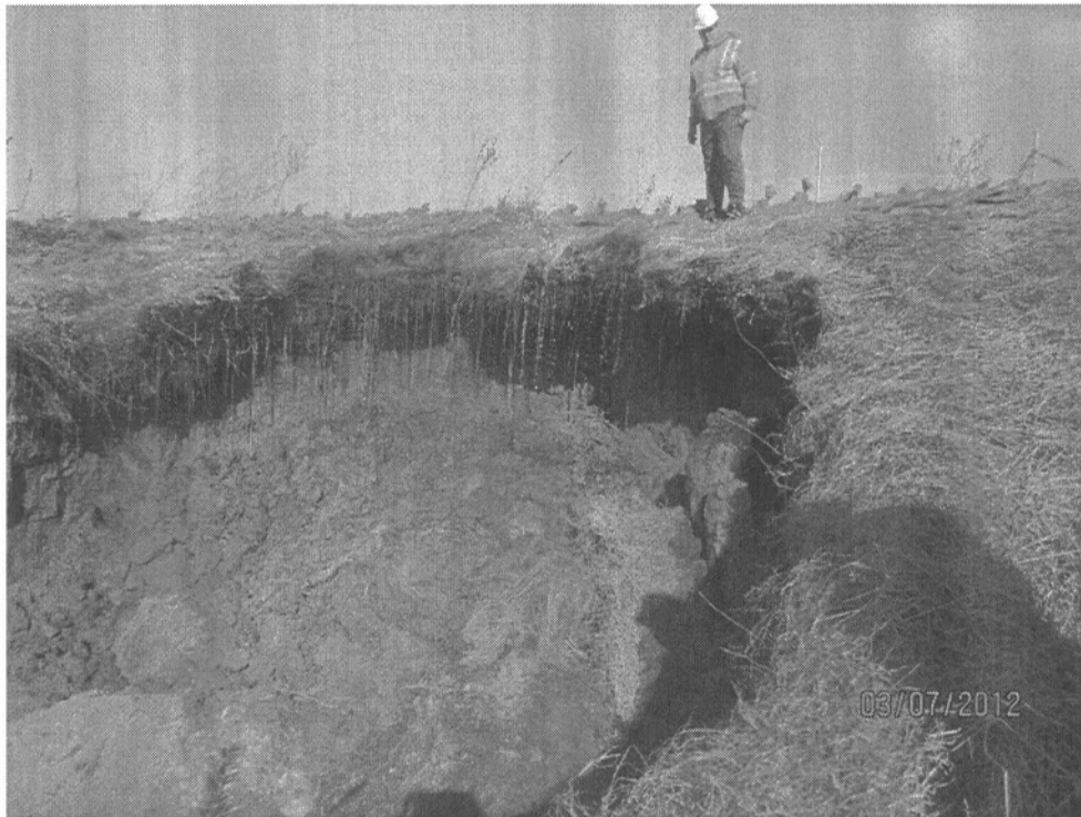
Figure 3: Slope Instability from the mid-height berm, towards north.
