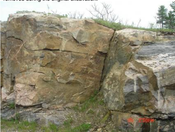
D) Highway 400 North Bound – Looking East at a saw-toothed wedge assumed to have either fallen out or was pulled out and removed during the original excavation.
