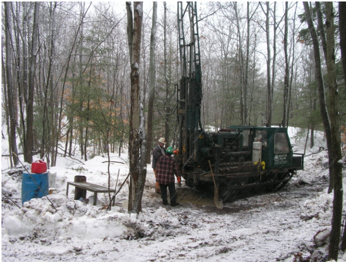
Photograph #13 View of drilling/coring for Well EBW12. Photo taken facing northeast.
