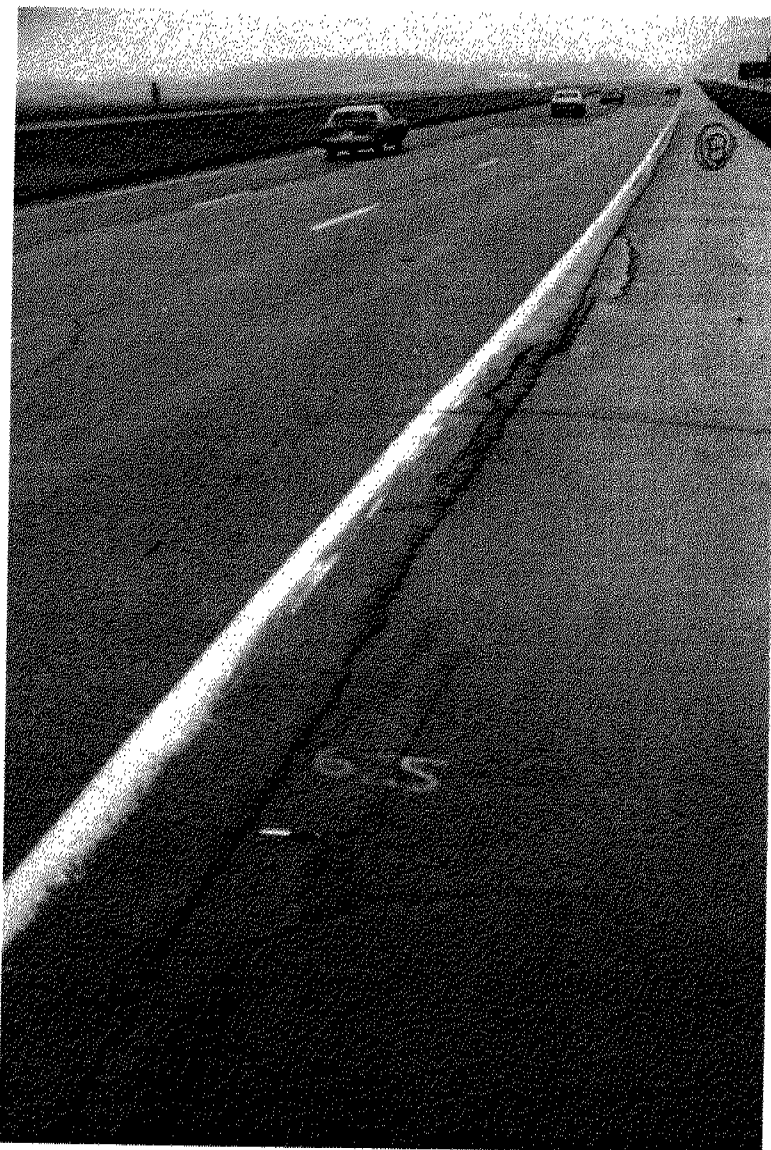
Severe stepping along outside edge of recently patched pavement section Sta. 10+665 N.B.L
