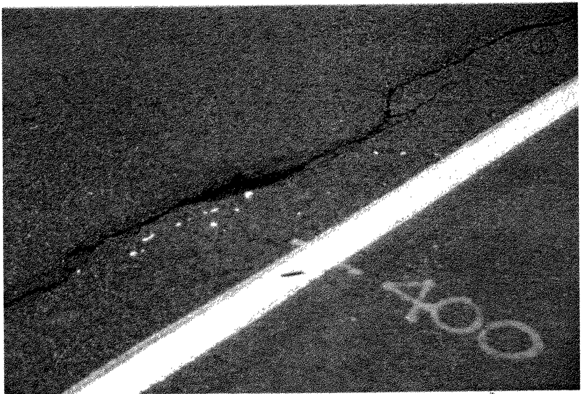
Very Severe Single Longitudinal Meandering Outer Wheel Track Crack Sta 10+400 N.B.L
