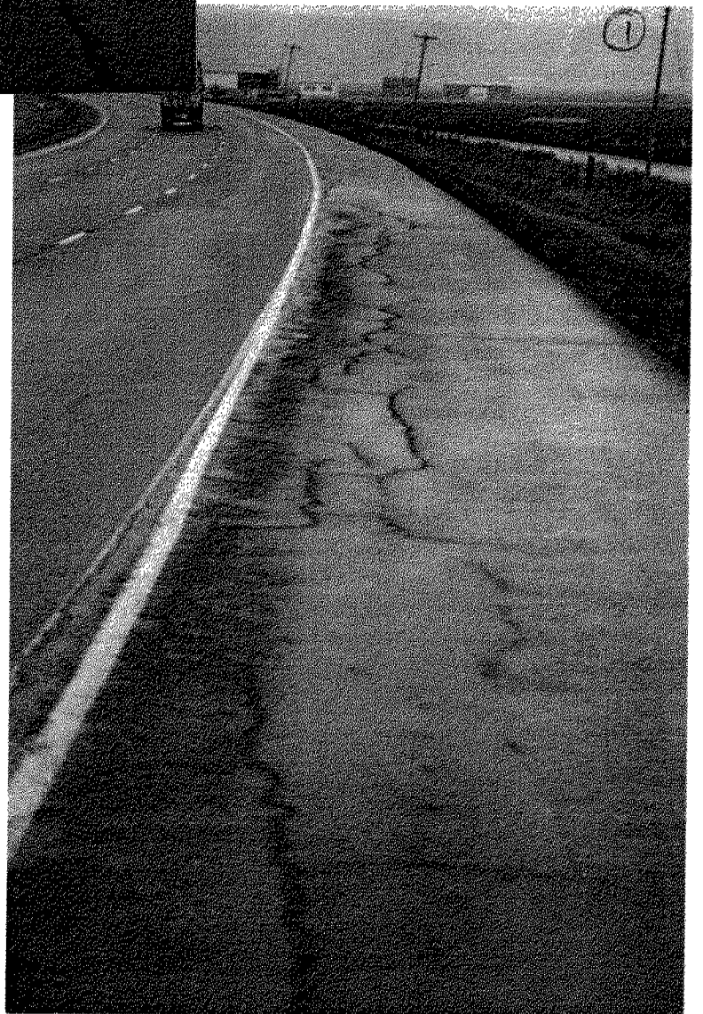
Severe to very severe multiple meandering cracks along shoulder Sta 10+700 N.B.L. looking north
