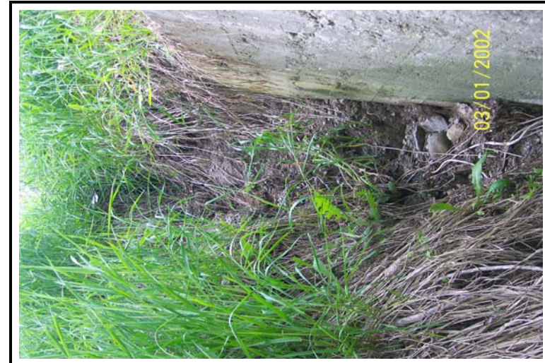
C28 Photo 4 Embankment Erosion at Northwest Corner
