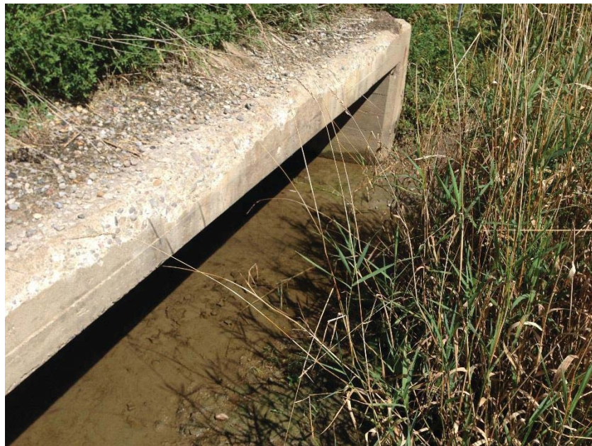
Photo 2: South end – existing culvert outlet.
