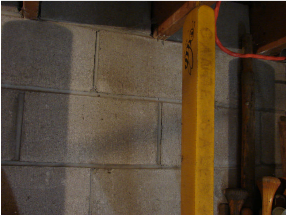
Photograph 33: Residence basement level east wall – concrete block step cracking, typical.
