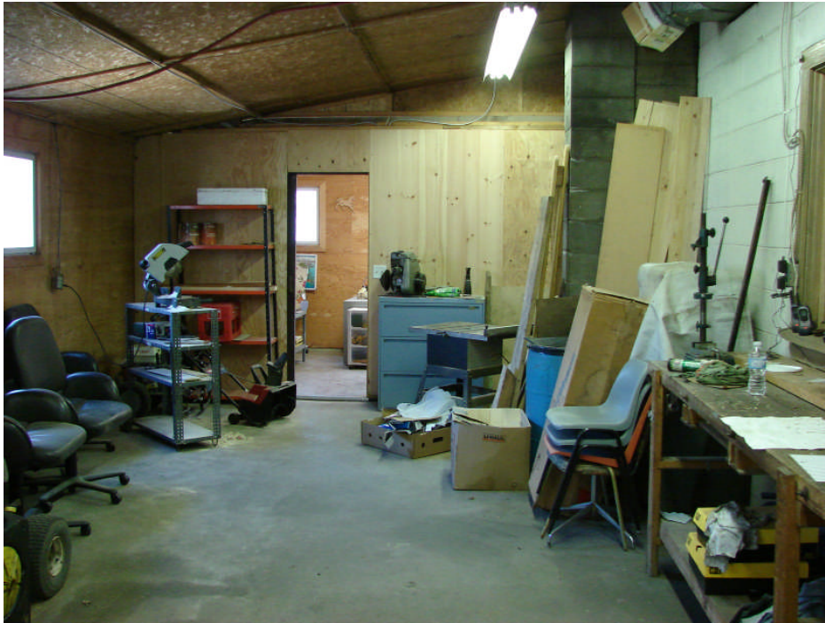
Photograph 55: Garage Building rear workshop – plywood wall cladding conceals the main structure.
