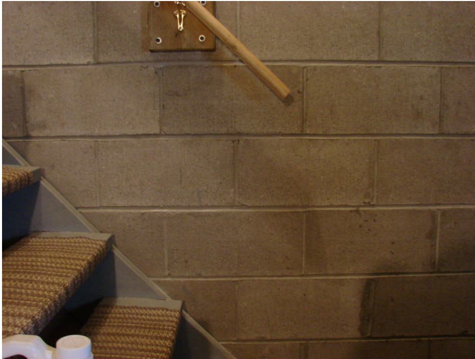
Photograph 41: Residence basement level west wall – concrete block wall step cracking near north end, typical.
