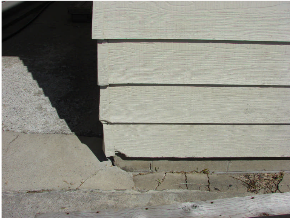
Photograph 3: Residence south elevation – impact damaged to siding and cracking slab-on-grade concrete at west end.
