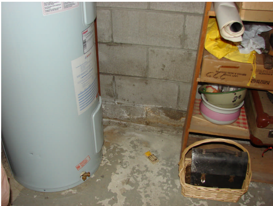
Photograph 40: Residence basement level west wall – moisture staining and efflorescence adjacent water heater, typical.
