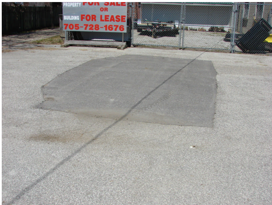
Photograph 27: Site Works – small asphalt patch/repair in southeast of the garage building.
