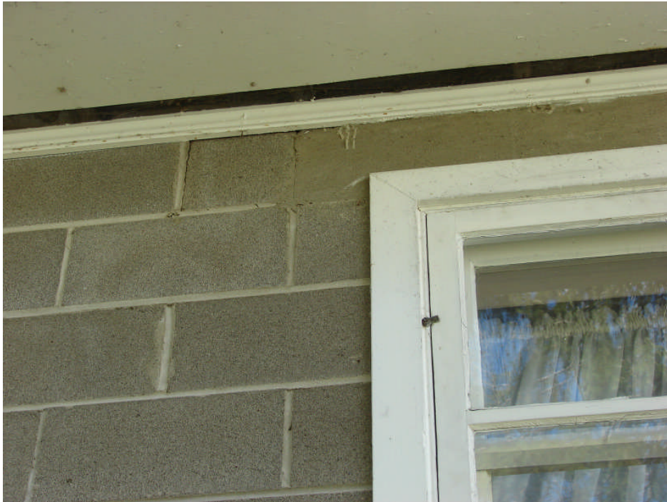
Photograph 19: Residence north elevation – cracked concrete block at soffit.
