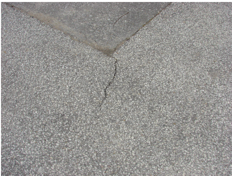
Photograph 24: Site Works – cracking of asphalt pavement adjacent the large asphalt patch/repair.
