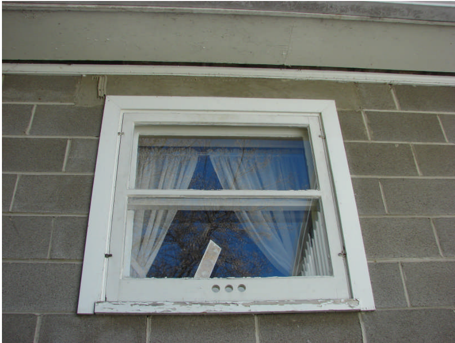
Photograph 15: Residence north elevation – soffit paint peeling, repaired window lintels, typical.
