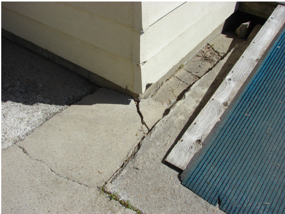
Photograph 10: Residence West elevation – severely deteriorated slab-on-grade concrete with extensive cracking, typical.
