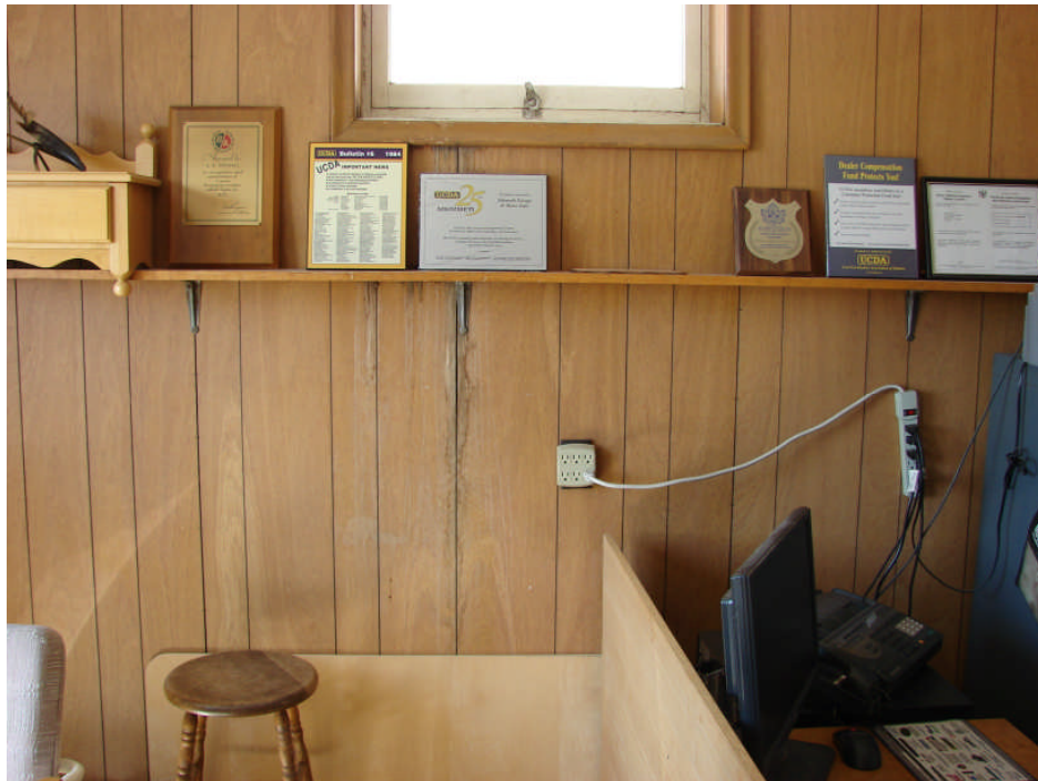
Photograph 55: Residence main floor level – moisture staining of wood panelling below west window at office.
