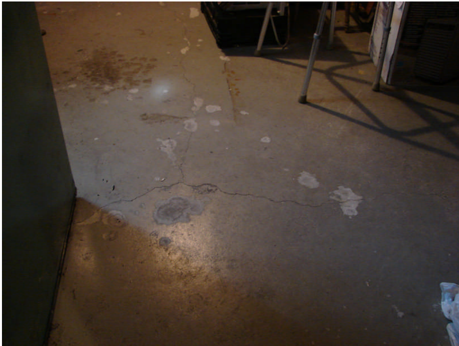
Photograph 44: Residence basement level – painted concrete slab-on-grade cracks, typical.
