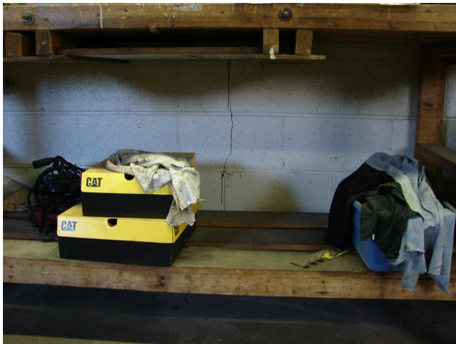
Photograph 57: Garage Building rear workshop south wall – wall step cracking below wall openings, typical.
