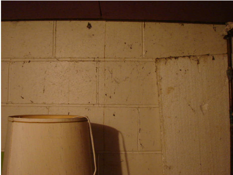
Photograph 37: Residence basement level south wall – concrete block wall step cracking near east end, typical.
