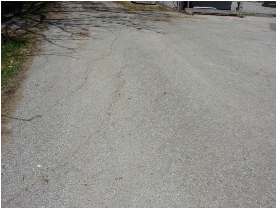
Photograph 30: Site Works – extensive cracking and some alligator cracking of asphalt pavement at the west end.
