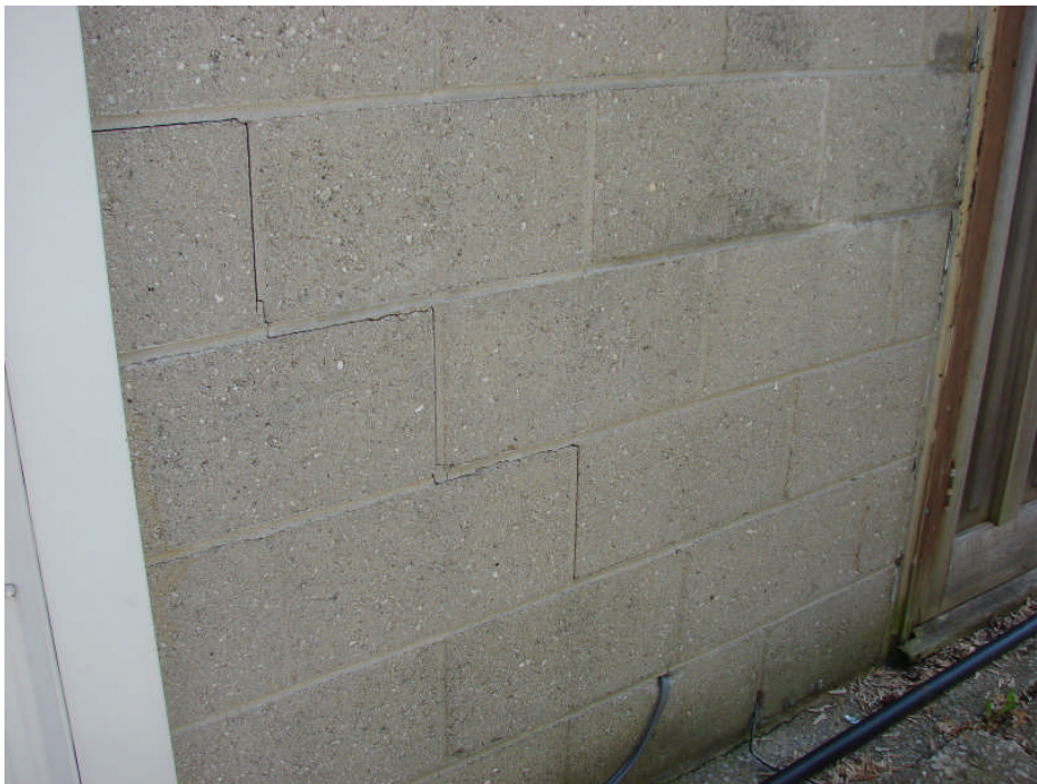
Photograph 16: Garage Building west elevation – concrete block wall step cracking between door and north gate, typical.
