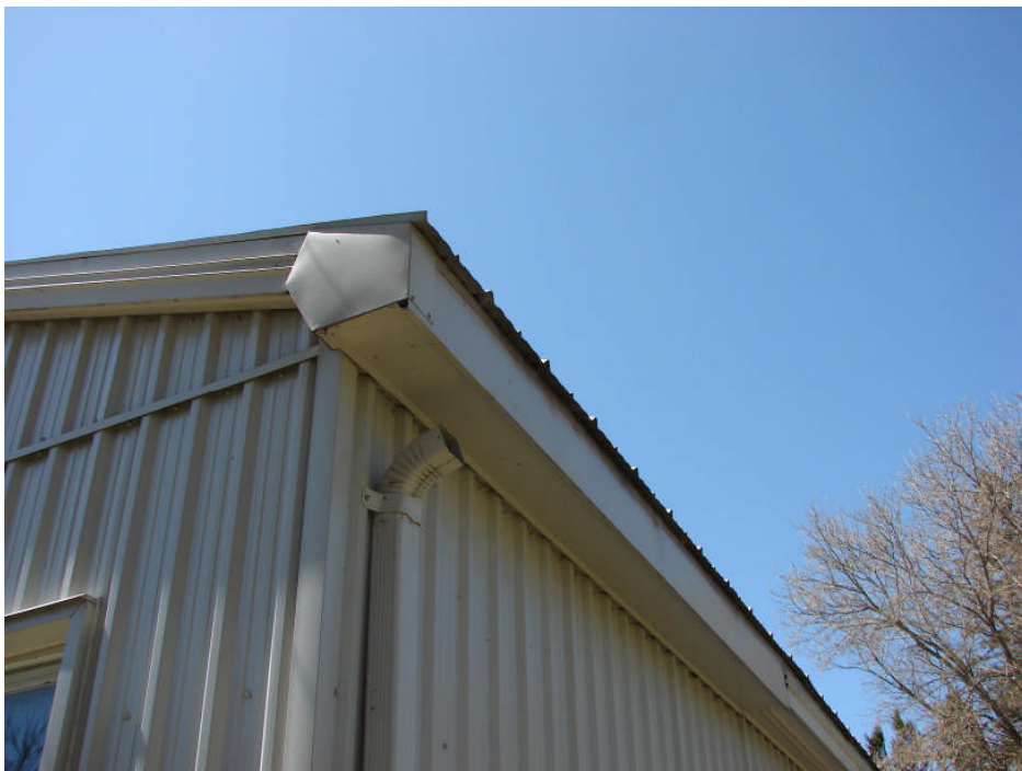
Photograph 24: Garage Building north elevation – missing rainwater gutter.
