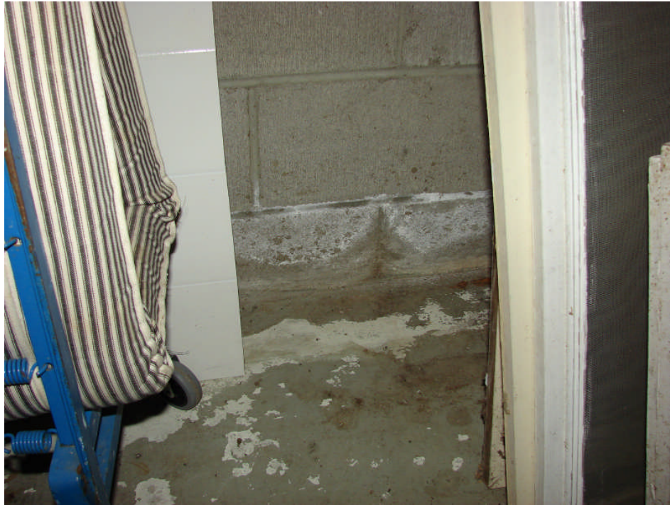
Photograph 27: Residence basement level north wall – moisture staining and efflorescence at the concrete block wall near west corner.
