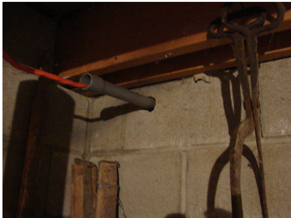
Photograph 30: Residence basement level east wall – unsealed wall penetration through concrete block.
