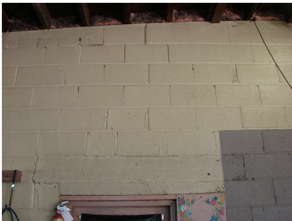
Photograph 46: Garage Building east wall – concrete block wall step cracking above exterior door, typical.
