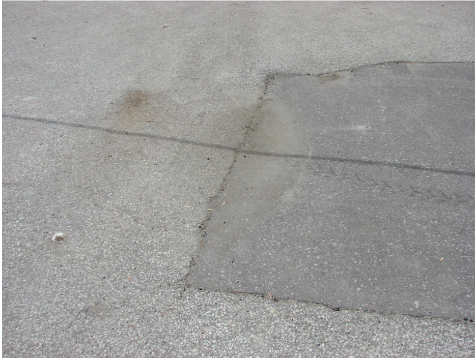
Photograph 29: Site Works – minor settlement and water ponding staining on the south side of the small asphalt patch/repair.
