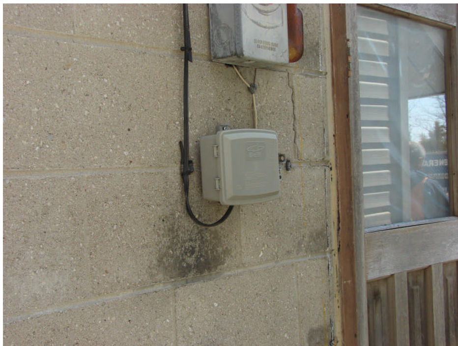
Photograph 17: Garage Building west elevation – concrete block wall step cracking near door on north side, typical.
