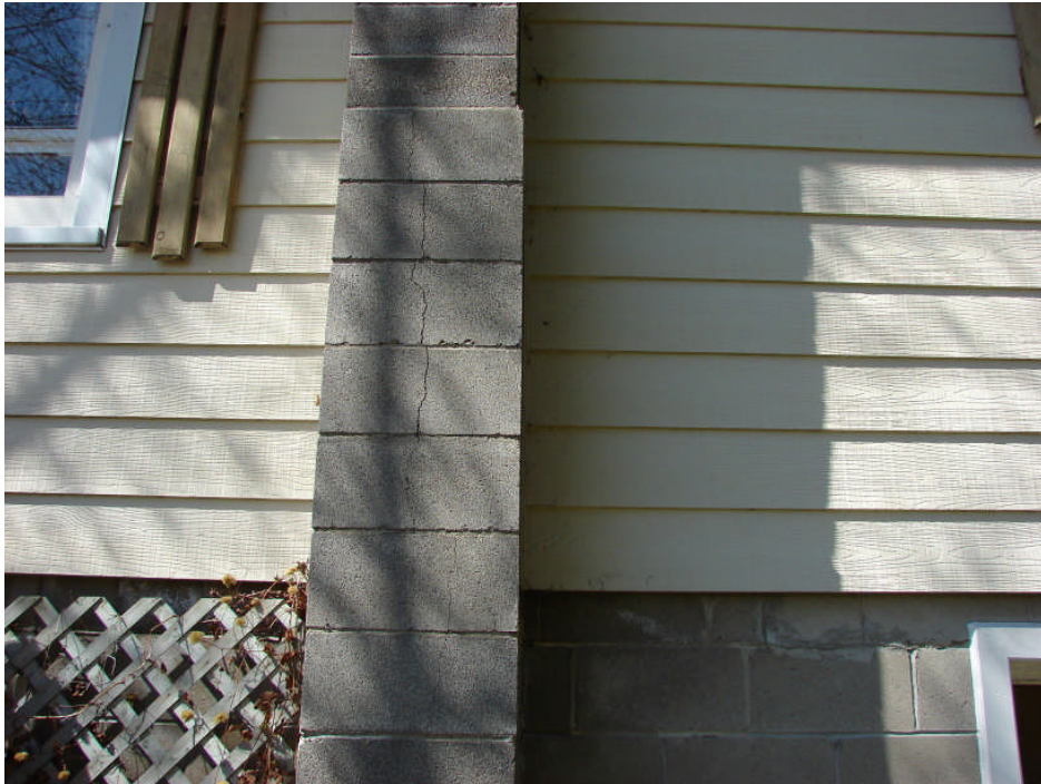
Photograph 23: Residence East elevation – concrete block cracks along east face of chimney.
