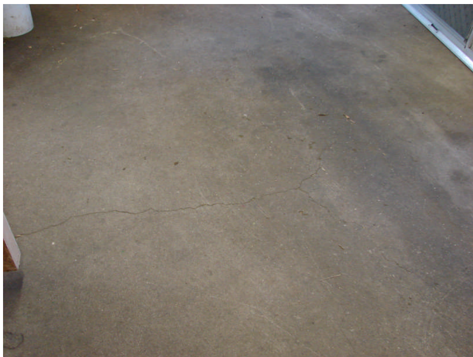
Photograph 58: Garage Building rear workshop - unpainted concrete slab-on-grade with minor cracks, typical.
