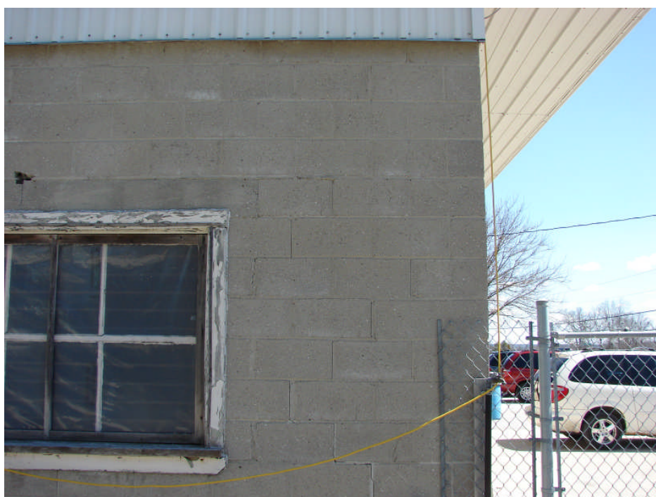
Photograph 12: Garage Building west elevation – concrete block wall step cracking above south window at south end, typical.
