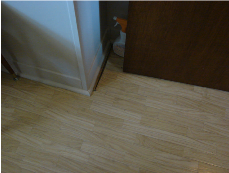
Photograph 51: Residence main floor level – vinyl sheet flooring / open seam along baseboard at centre bedroom on north side, typical.
