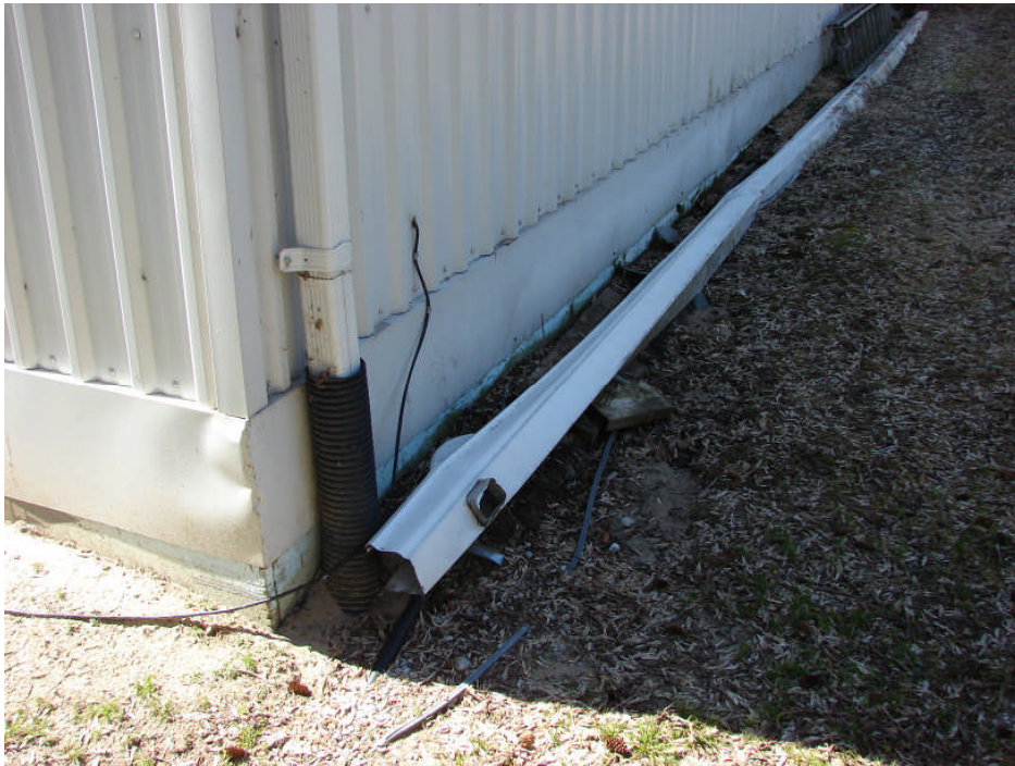
Photograph 23: Garage Building north elevation – damaged eavestrough resting on ground.
