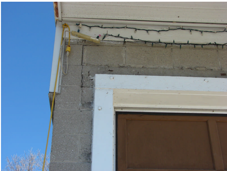
Photograph 3: Garage Building south elevation – concrete block wall step cracking at west end adjacent overhead door, typical.
