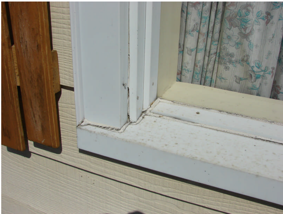
Photograph 4: Residence south elevation – Aged and deteriorated windows caulking, typical.
