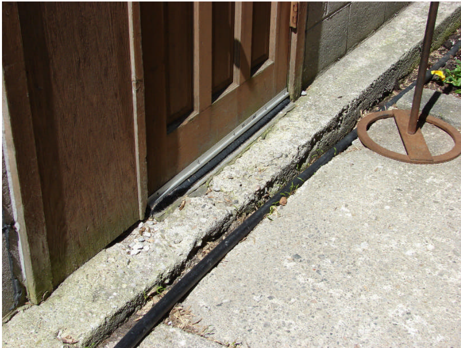
Photograph 31: Garage Building east elevation (south part) – severely deteriorated and breaking concrete door threshold, typical.
