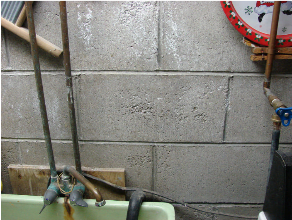
Photograph 39: Residence basement level south wall – extensive efflorescence and wall pitting of concrete block, typical.
