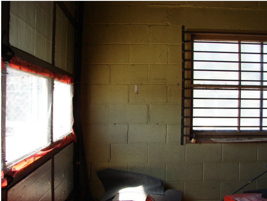
Photograph 49: Garage Building west wall – concrete block wall step cracking at south end, typical.
