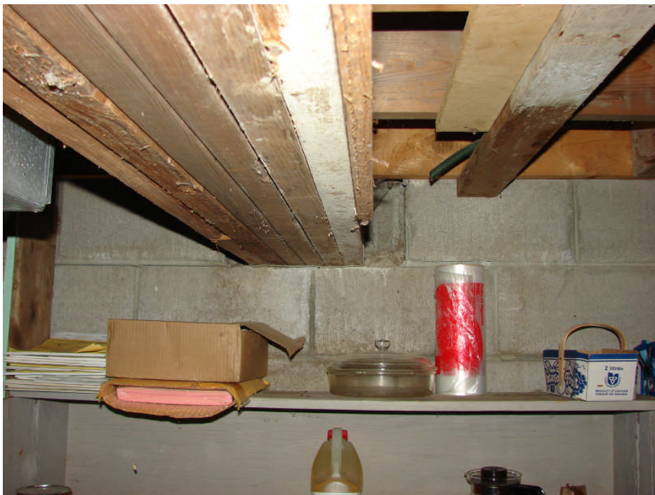
Photograph 42: Residence basement level west wall – concrete block wall joint cracking at beam pocket.
