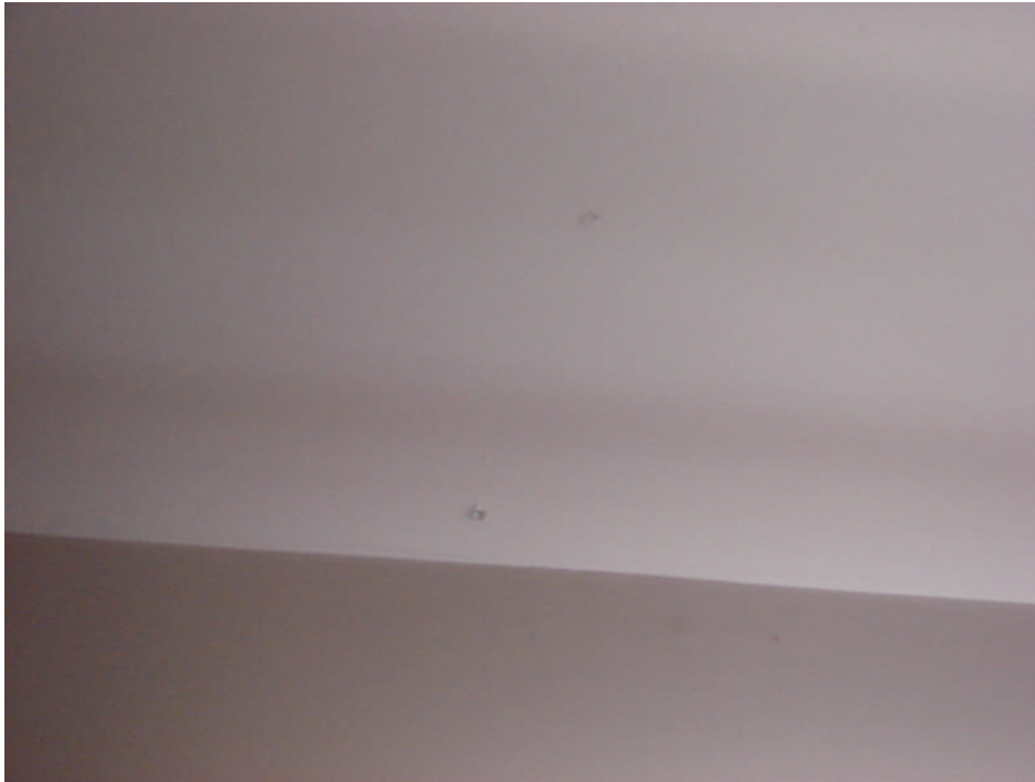
Photograph 47: Residence main floor level – ceiling drywall popped nails at north end of northwest bedroom.
