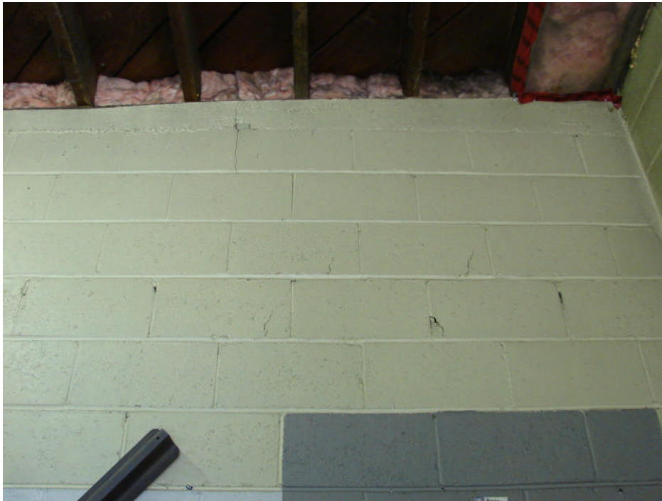
Photograph 47: Garage Building east wall – concrete block wall step cracking at south end, typical.
