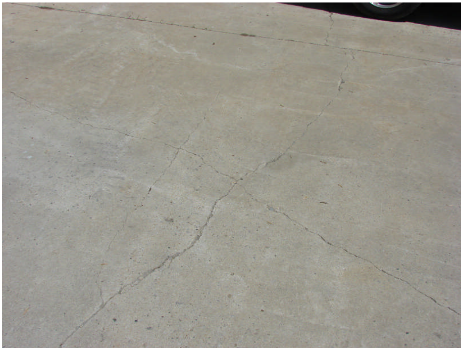
Photograph 35: Site Works – cracking of concrete slab-on-grade pad south of the east overhead door to the garage building, typical.
