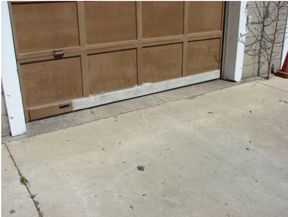
Photograph 5: Garage Building south elevation – concrete slab-on-grade cracking at east overhead door, typical.
