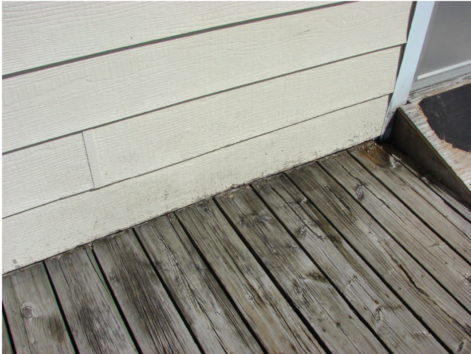
Photograph 5: Residence south elevation – Aged and deteriorated wood porch decking, typical.
