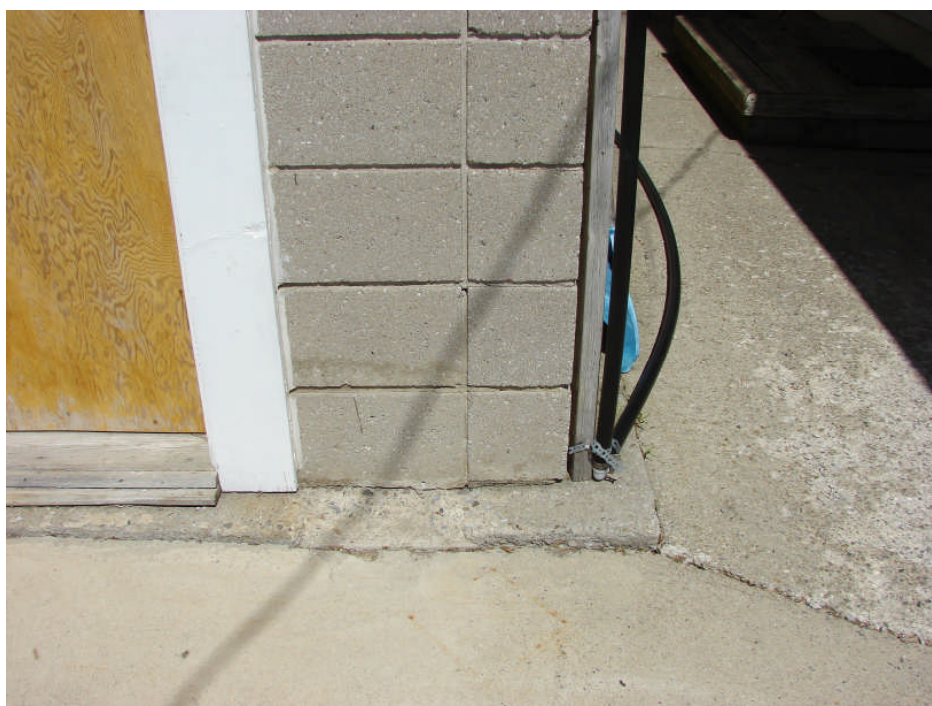
Photograph 8: Garage Building south elevation – concrete block wall step cracking at east end, typical.
