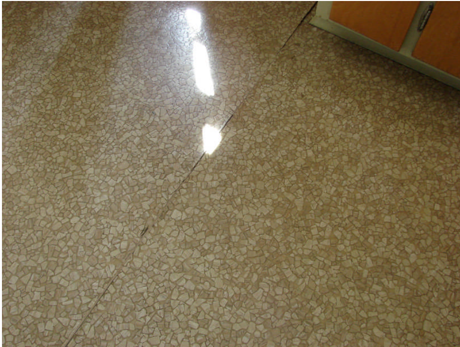
Photograph 49: Residence main floor level– open seam at vinyl sheet flooring at kitchen, typical.
