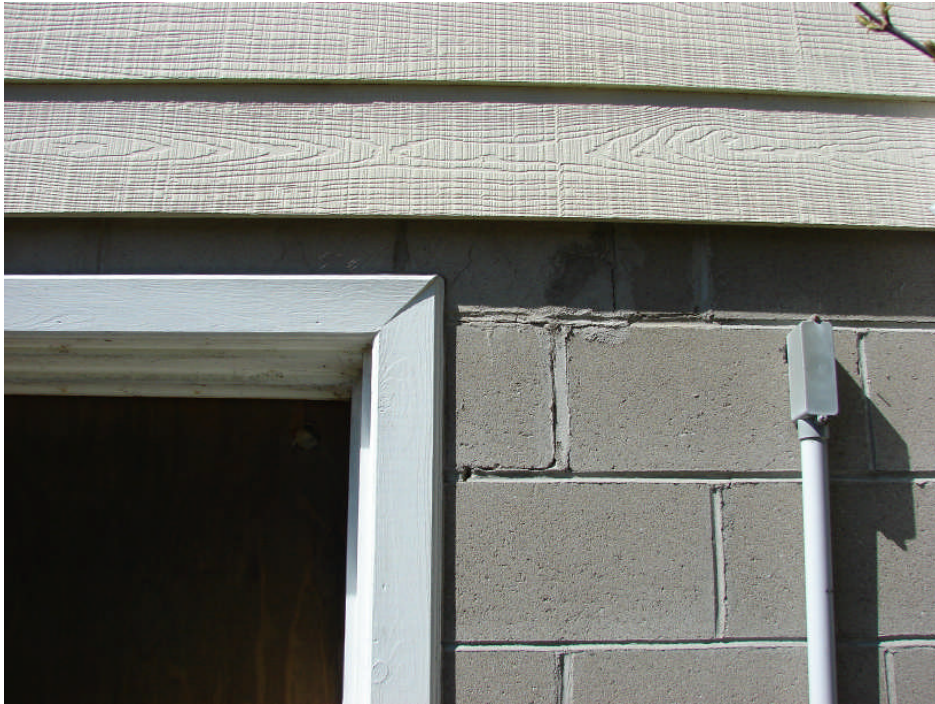
Photograph 21: Residence east elevation – concrete block wall step cracking at north end of basement lintel door frame.
