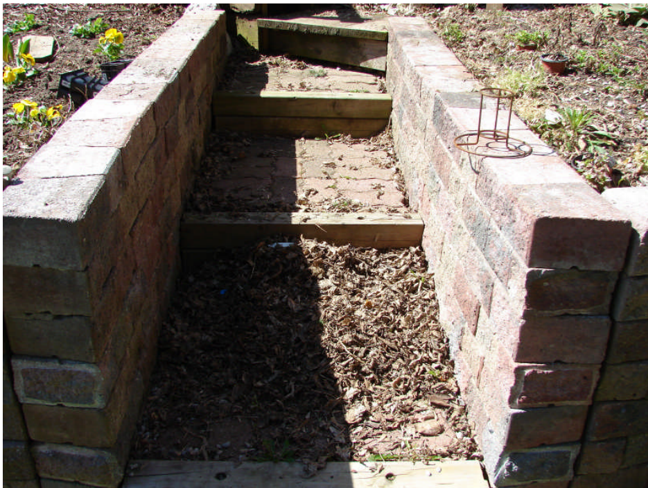
Photograph 24: Residence east elevation – differential settlement of interlocking unit pavers at landscaped areas, typical.
