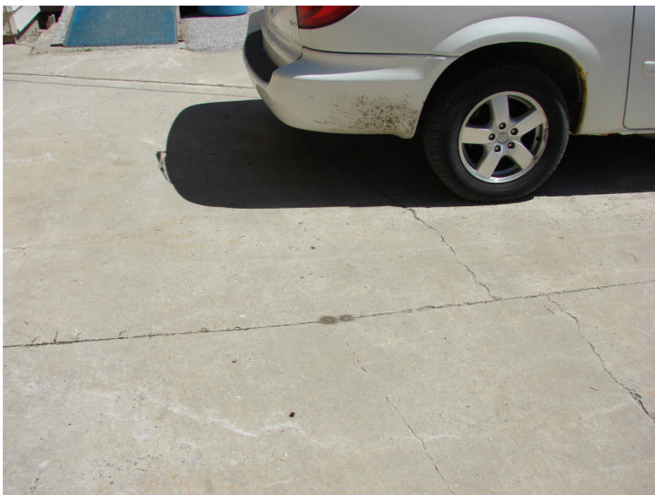
Photograph 36: Site Works – cracking of concrete slab-on-grade pad south of the east overhead door to the garage building, typical.
