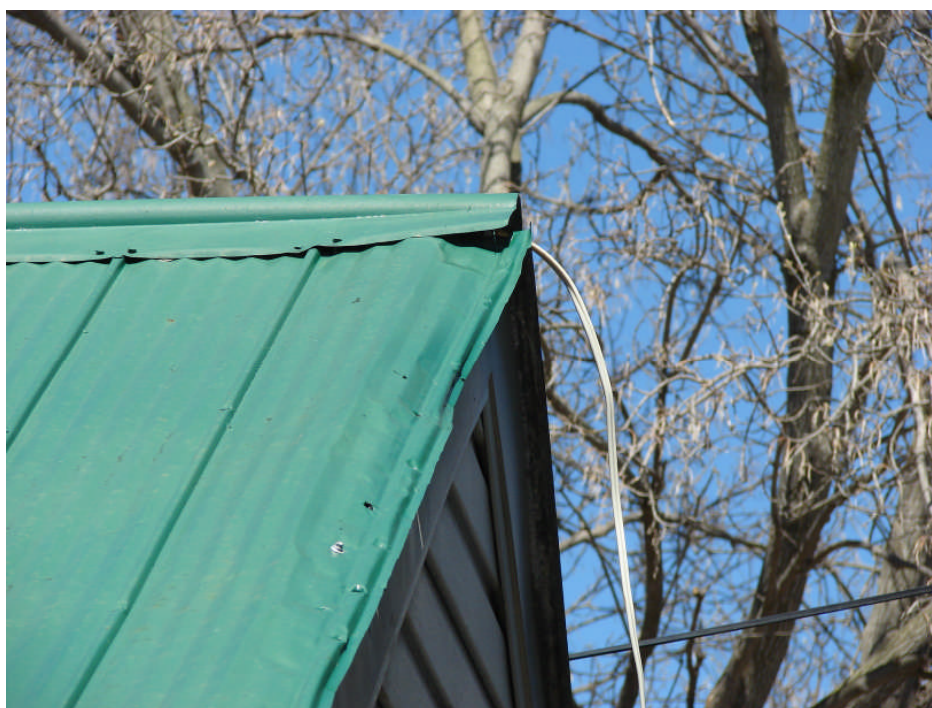
Photograph 8: Other Structures Storage Building - roof ridge missing end cap at east end, typical.
