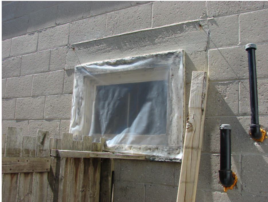
Photograph 27: Garage Building east elevation (north part) – aged and deteriorated window paint with peeling/blistering paint, typical
