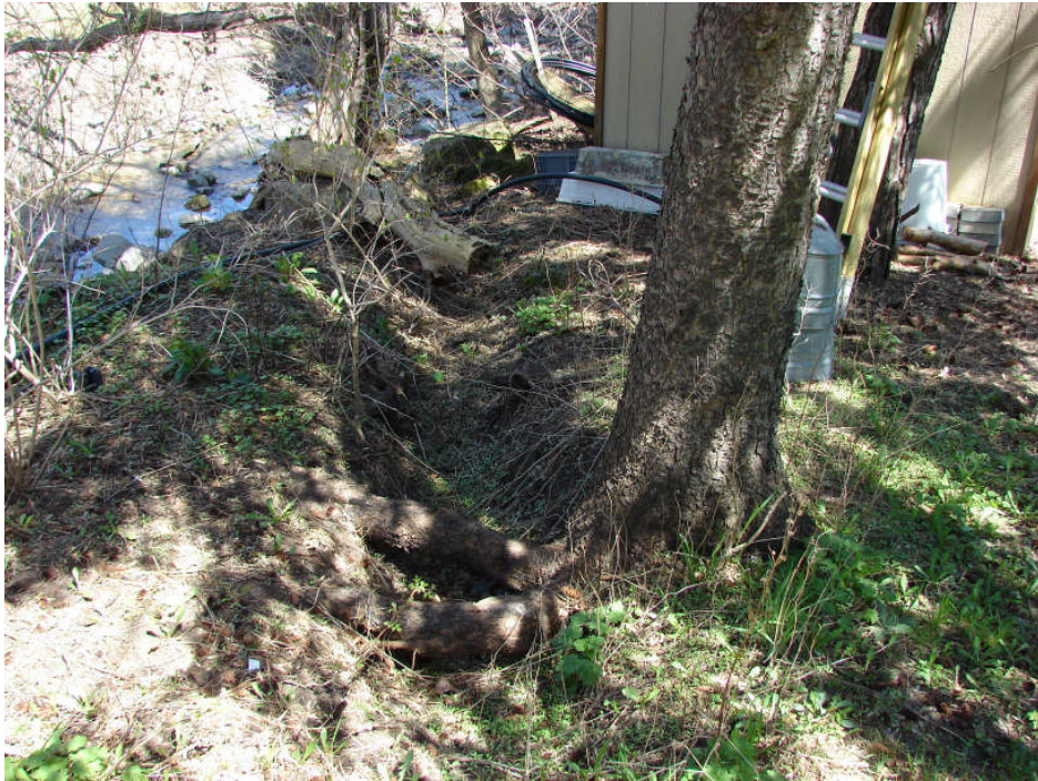
Photograph 13: Site Works – general view along south side of drainage ditch near residence looking east, with extensive soil erosion, typical.
