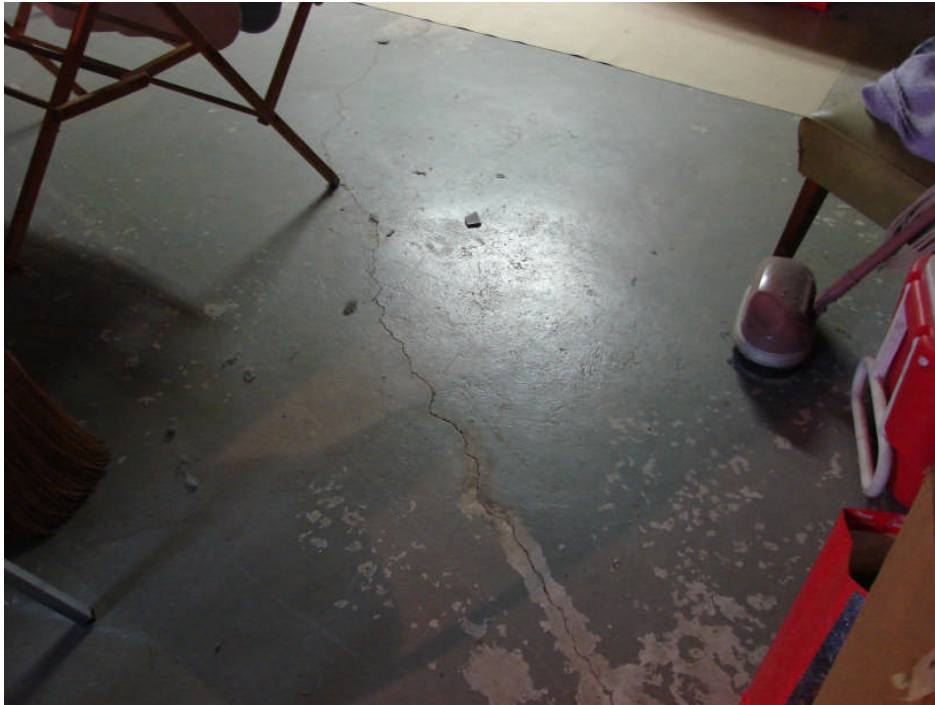
Photograph 43: Residence basement level – painted concrete slab-on-grade cracks, typical.
