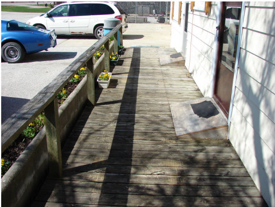
Photograph 8: Residence south elevation – aged and deteriorated pressure treated wood porch decking and guardrail, typical.
