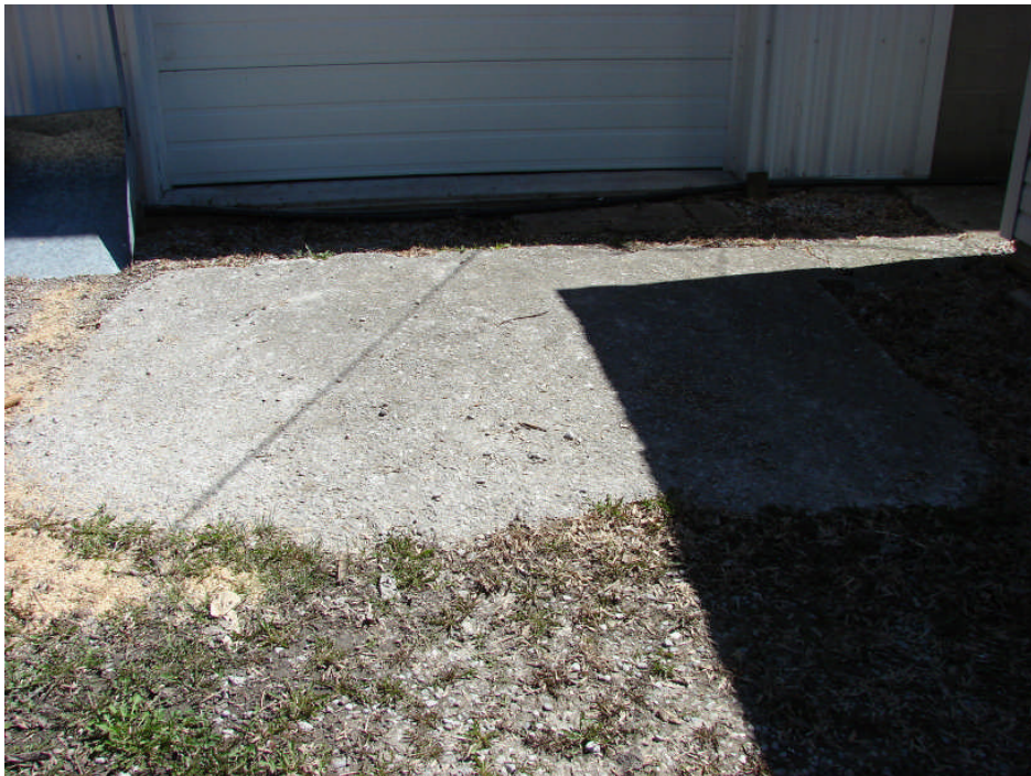
Photograph 20: Garage Building west elevation – extensive deterioration of concrete slab-on-grade with severe surface spalling, typical.
