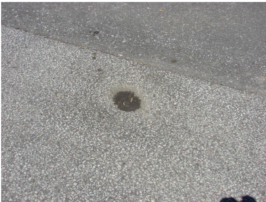
Photograph 23: Site Works – hole in the asphalt pavement near the large asphalt patch/repair.
