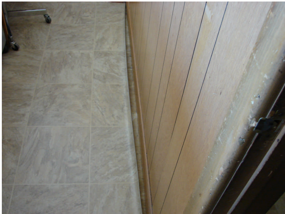
Photograph 56: Residence main floor level – open seam at vinyl sheet flooring along north baseboard.
