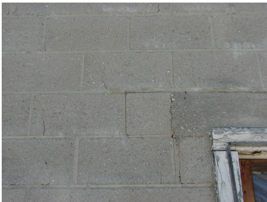
Photograph 14: Garage Building west elevation – concrete block wall step cracking above north end of south window, typical.
