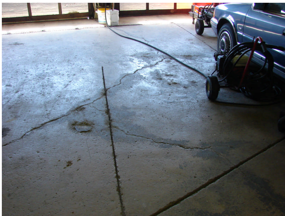
Photograph 53: Garage Building – unpainted concrete slab-on-grade central areas cracks, typical.
