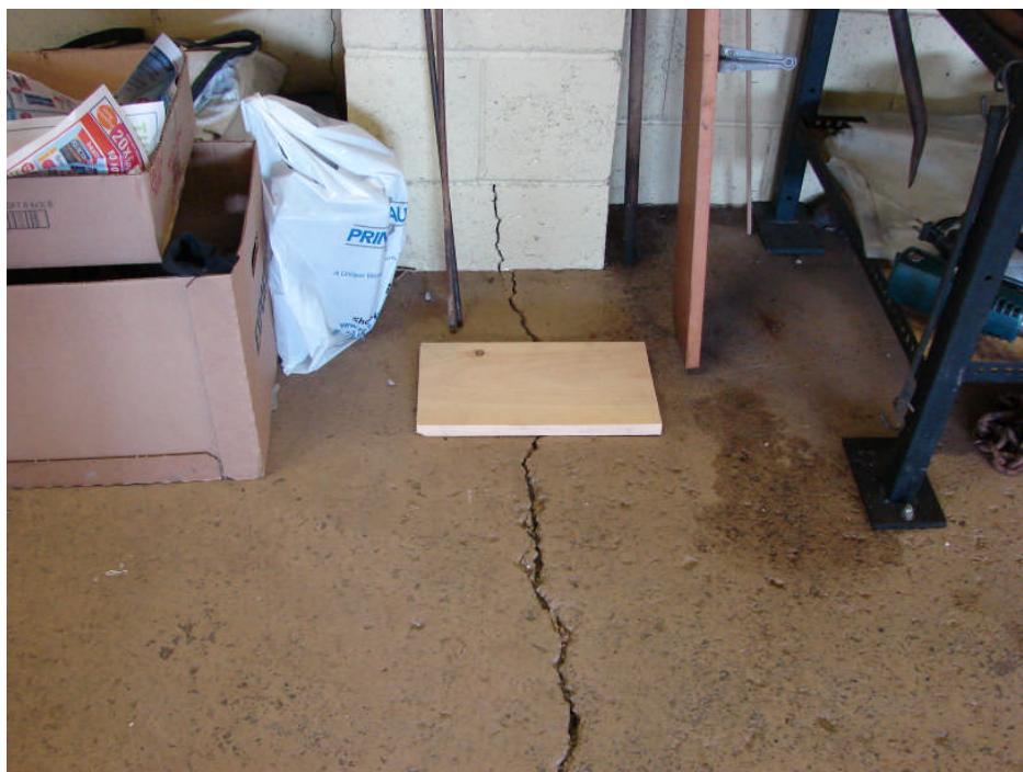
Photograph 40: Garage Building north wall – continued wall and slab cracks at east concrete block pier, typical.
