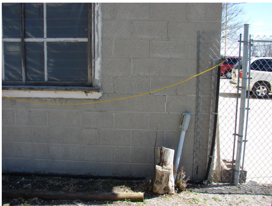
Photograph 11: Garage Building west elevation – concrete block wall step cracking at south end, typical.
