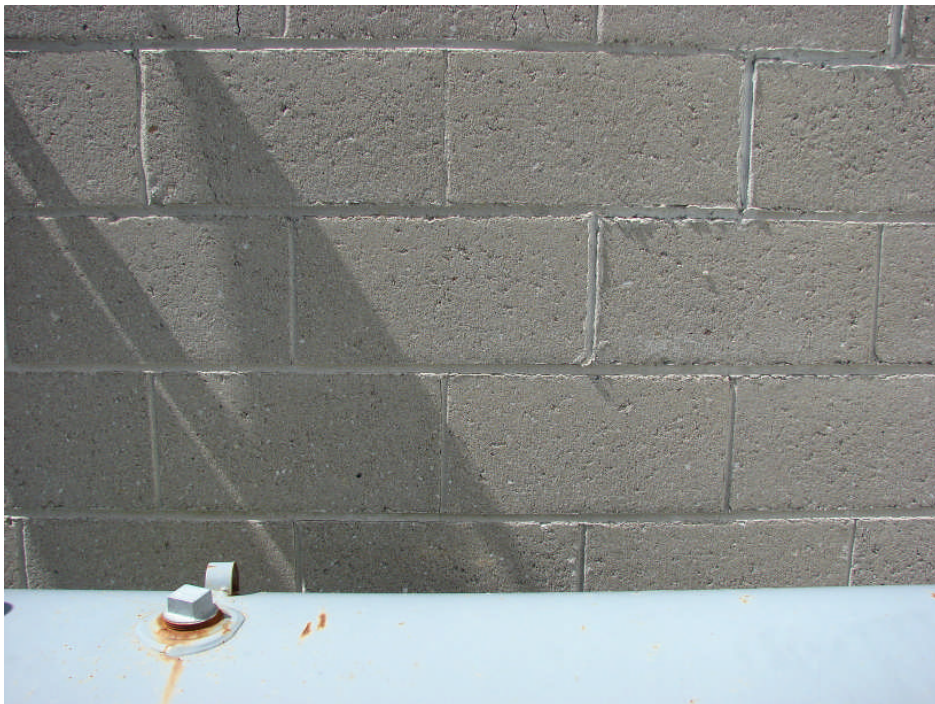
Photograph 26: Garage Building east elevation (north part) – concrete block wall step cracking near oil tank, typical.
