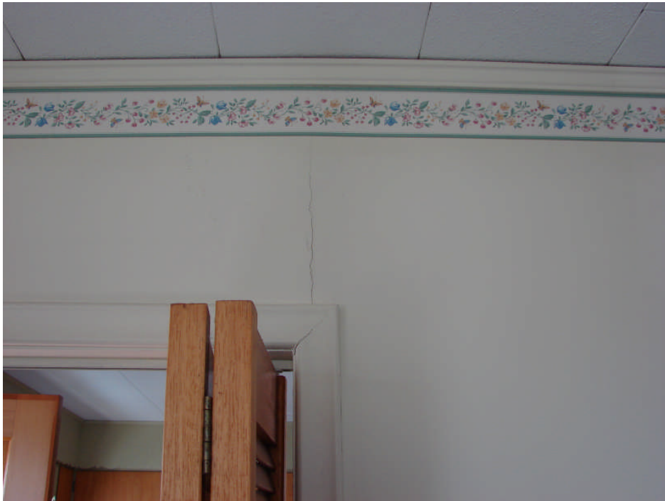
Photograph 50: Residence main floor level – drywall crack above door at family room to entrance vestibule.
