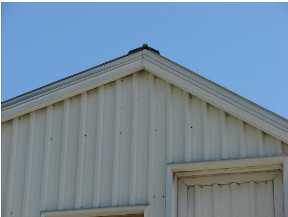
Photograph 10: Garage Building west elevation – missing ridge end cover at west side of metal roof, typical.
