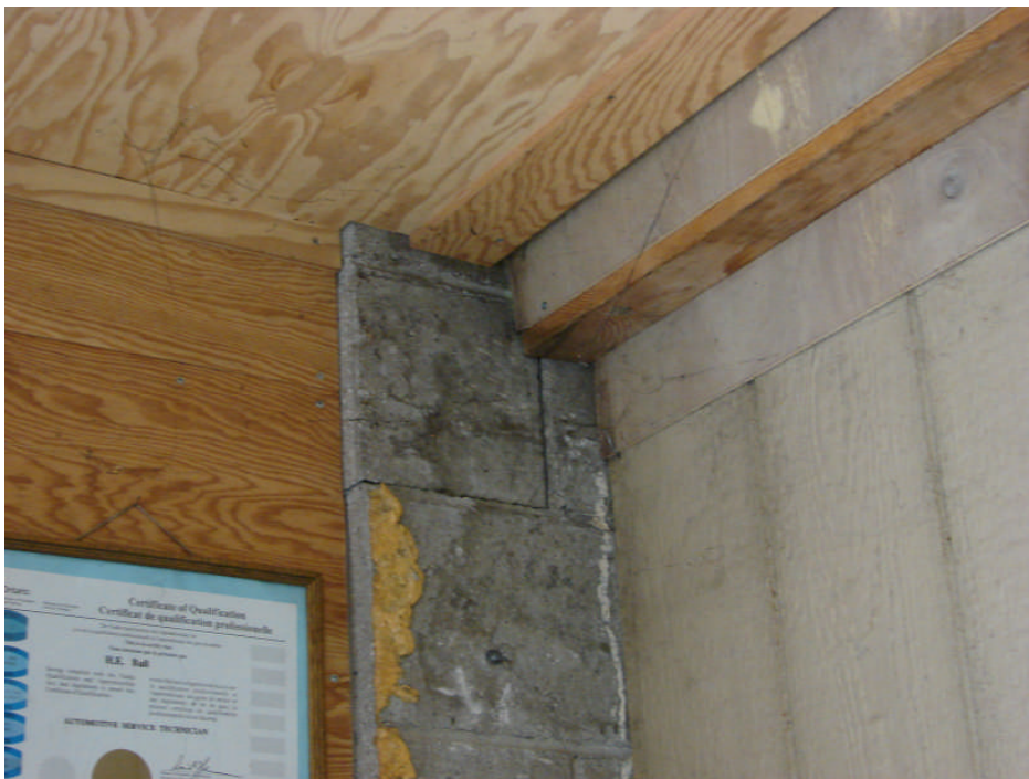
Photograph 56: Garage Building rear workshop – office southwest corner wall cracks.
