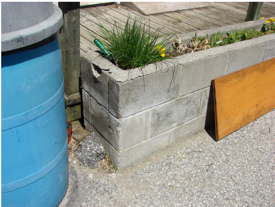
Photograph 40: Site Works – concrete block joint cracking at planter box including loose and cracking grout coping along south building elevation, typical.
