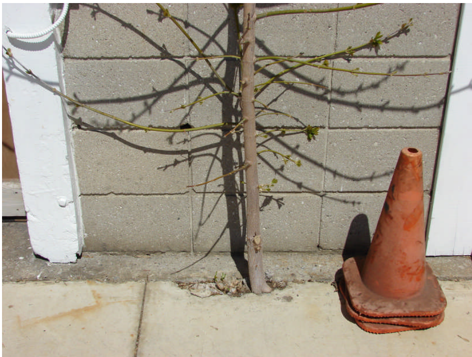
Photograph 6: Garage Building south elevation – vegetation growth through concrete slab-on-grade at east overhead door.
