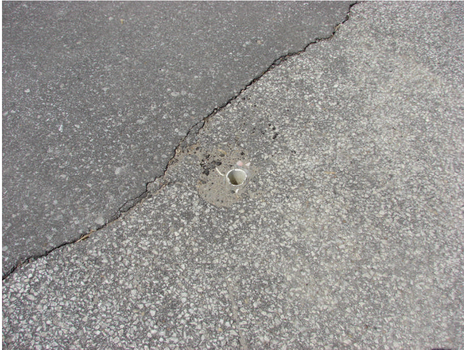
Photograph 25: Site Works – hole in the asphalt pavement near the large asphalt patch/repair.
