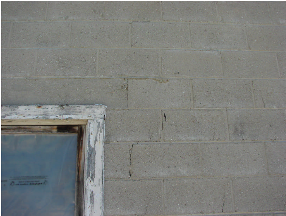
Photograph 15: Garage Building west elevation – concrete block wall step cracking above south end of south window, typical.
