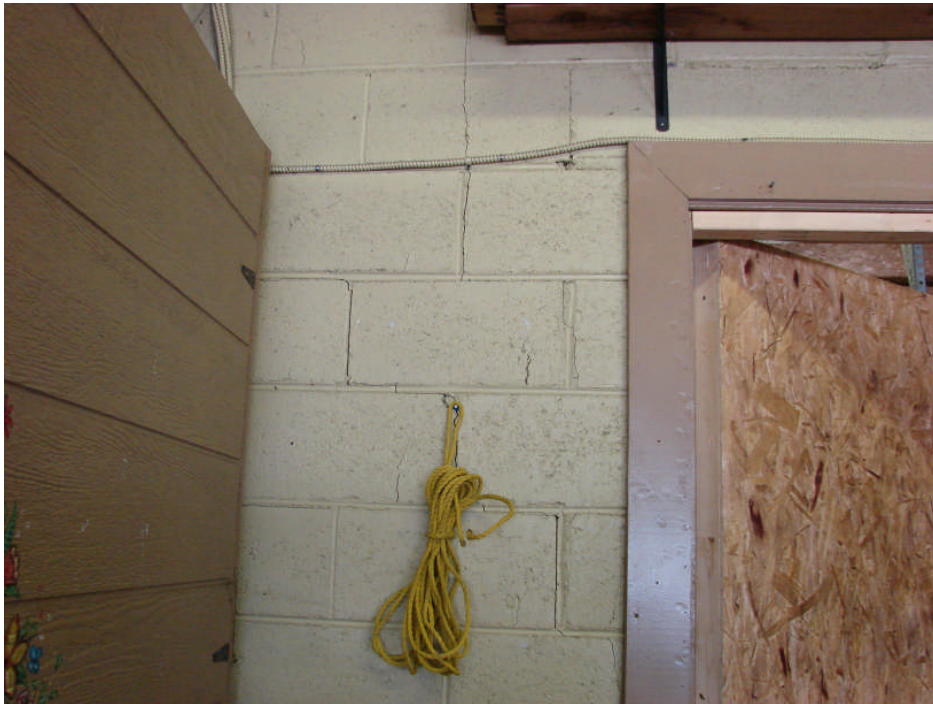
Photograph 37: Garage Building north wall – concrete block wall step cracking near west end, typical.
