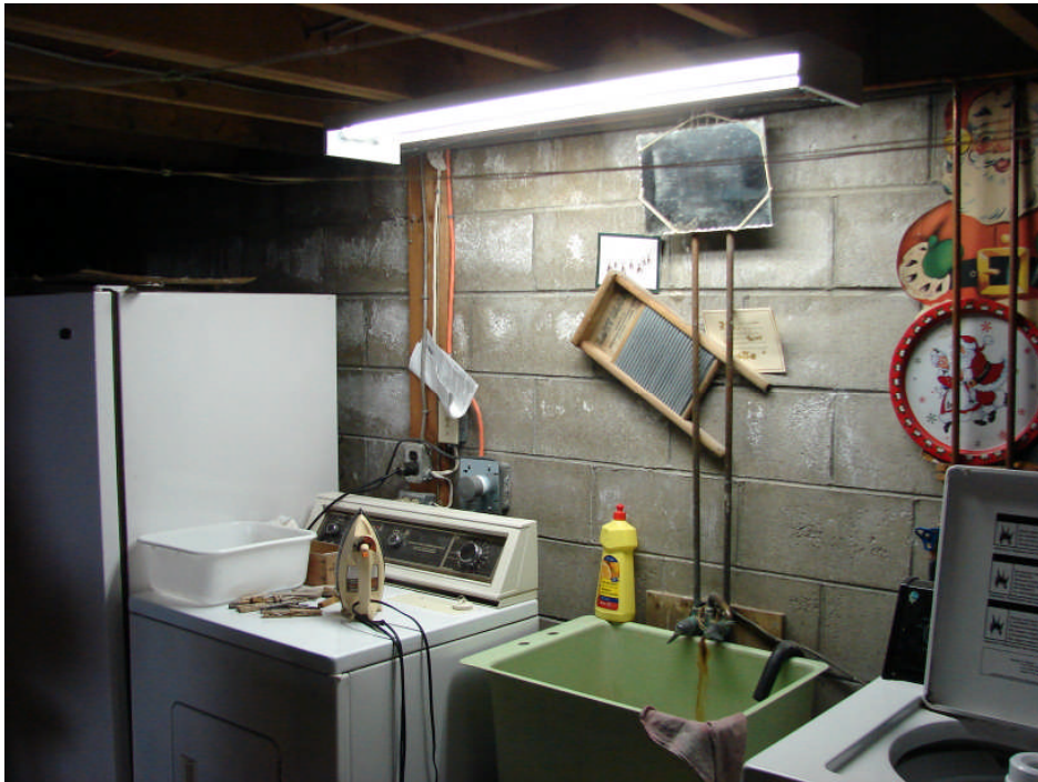
Photograph 38: Residence basement level south wall – extensive efflorescence and wall pitting of concrete block, typical.
