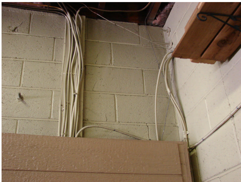
Photograph 52: Garage Building west wall – concrete block wall step cracking above electrical panel at north end, typical.
