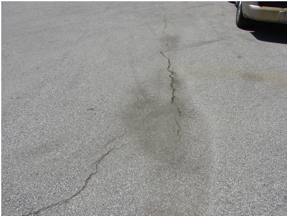
Photograph 22: Site Works – cracking of asphalt pavement along Highway 26 near entrance, typical.
