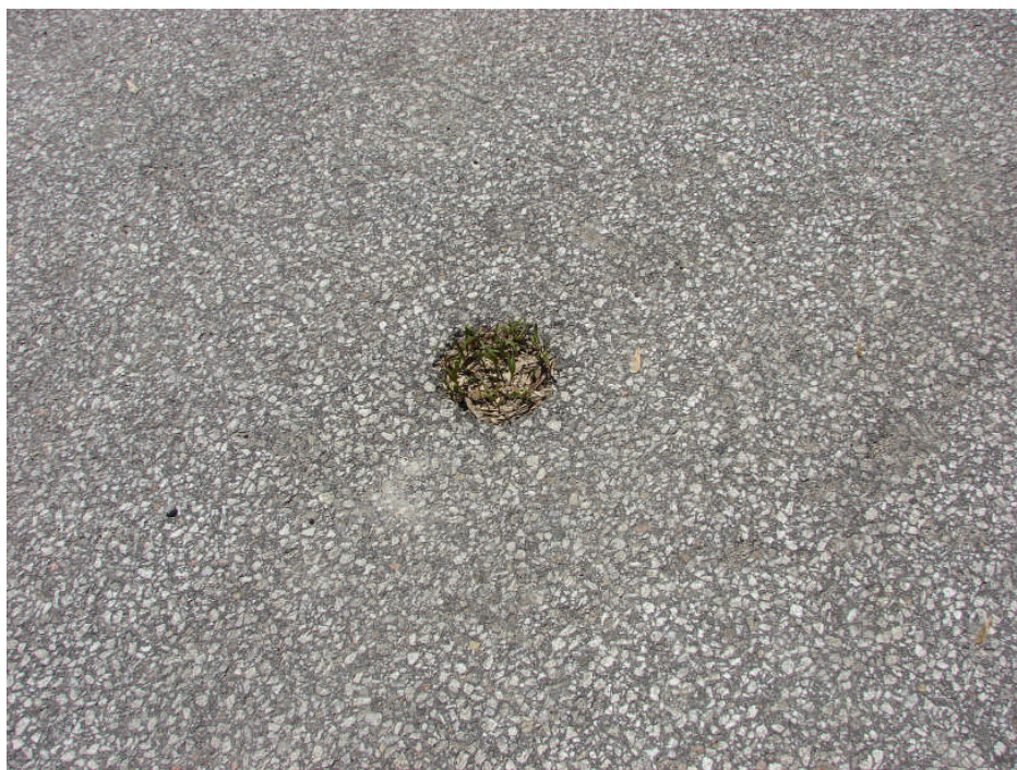
Photograph 28: Site Works – hole in the asphalt pavement near the small asphalt patch/repair.
