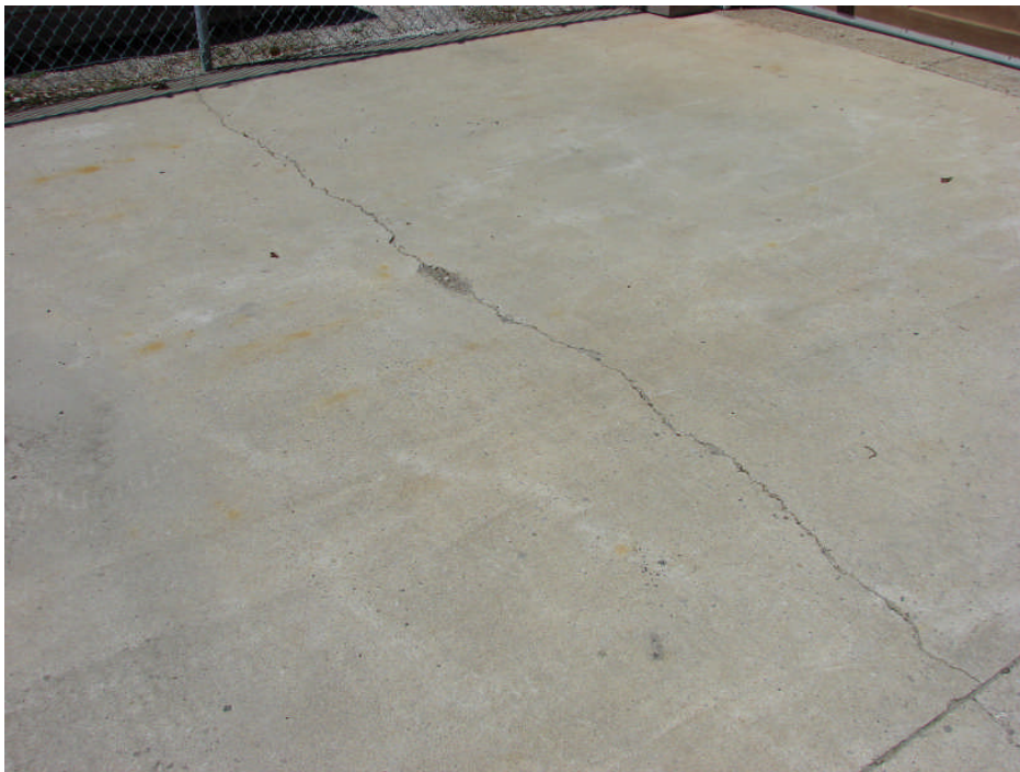
Photograph 34: Site Works – cracking of concrete slab-on-grade pad south of the west overhead door to the garage building, typical.
