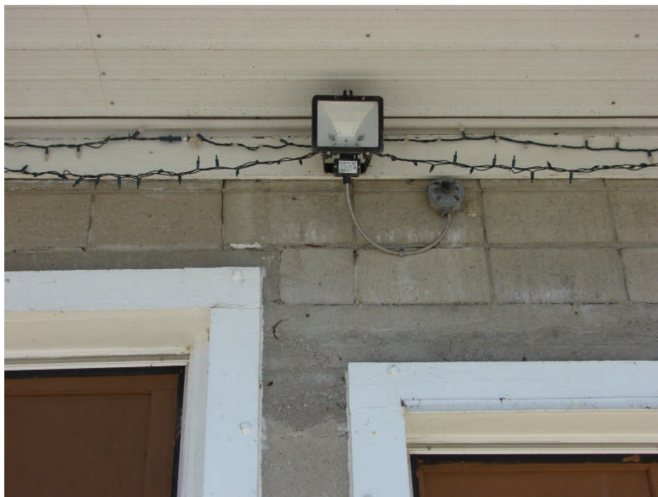
Photograph 7: Garage Building south elevation –concrete block wall step cracking between overhead doors, typical.
