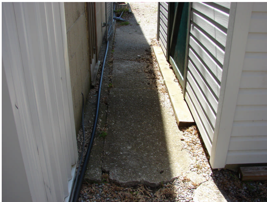
Photograph 21: Garage Building west elevation – deterioration of concrete slab-on-grade with surface spalling and differential settlement, typical.
