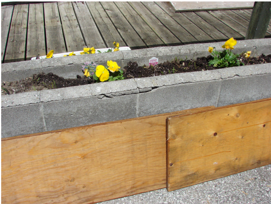
Photograph 42: Site Works – concrete block joint cracking at planter box including loose and cracking grout coping along south building elevation, typical.
