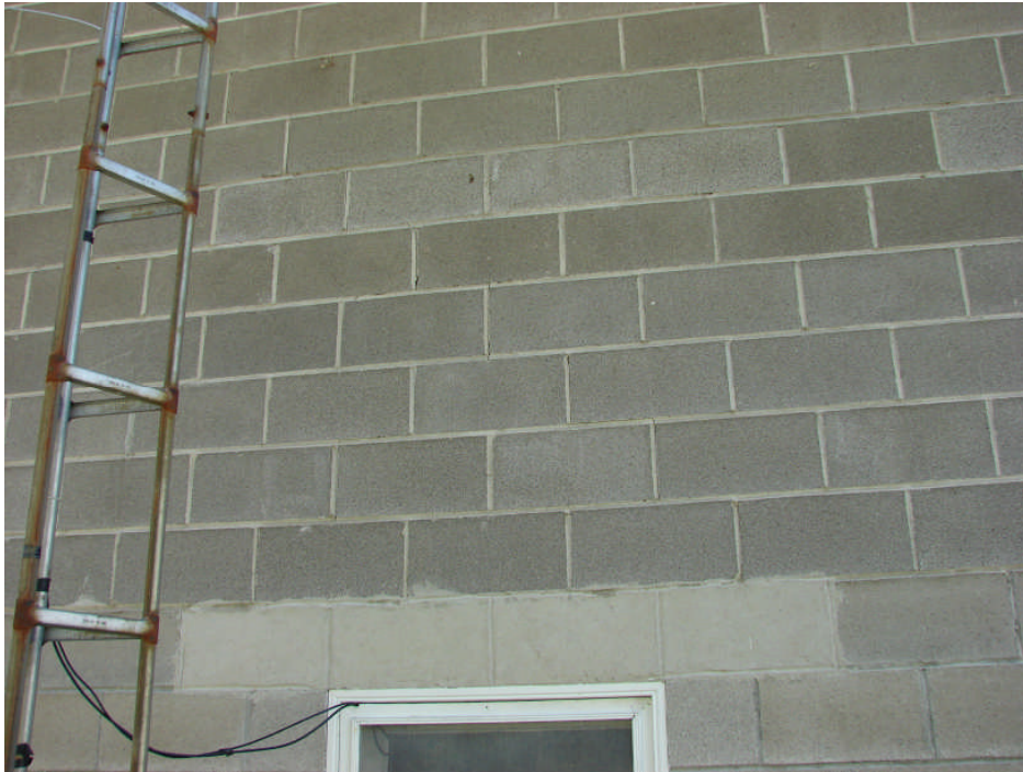
Photograph 17: Residence north elevation – Basement and main floor concrete block step cracking near east end, typical.
