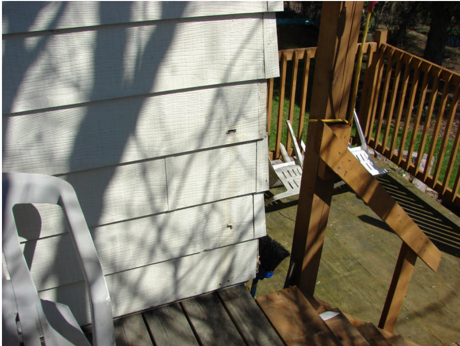
Photograph 7: Residence south elevation – nail holes on siding at east end.
