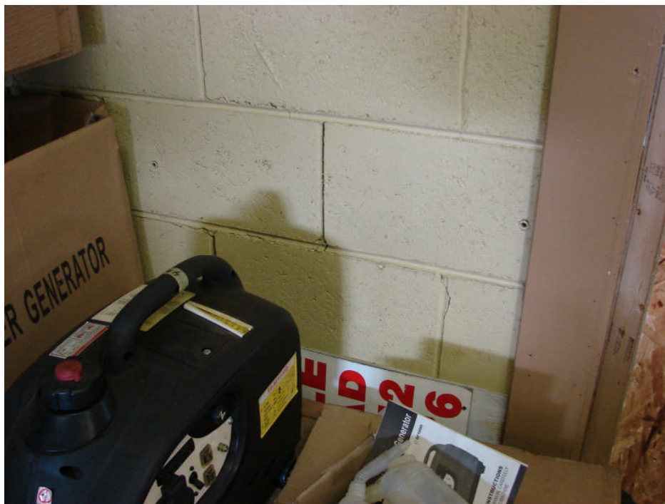
Photograph 36: Garage Building north wall – concrete block wall step cracking near west end, typical.
