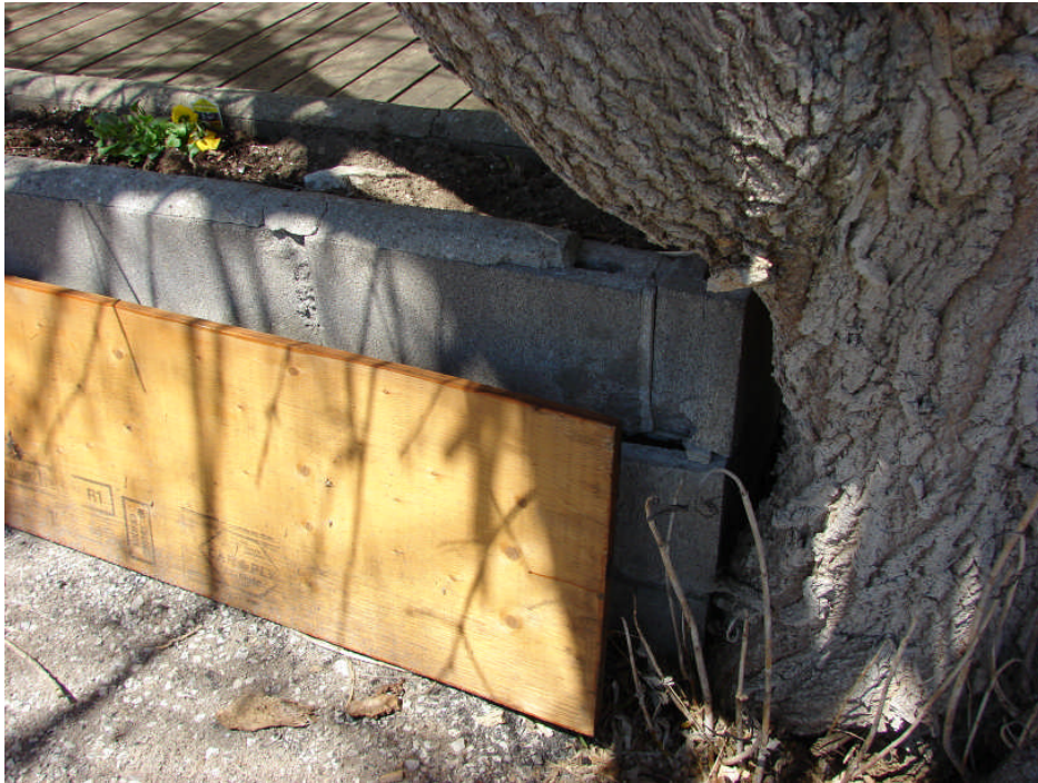
Photograph 41: Site Works – concrete block joint cracking at planter box including loose and cracking grout coping along south building elevation, typical.
