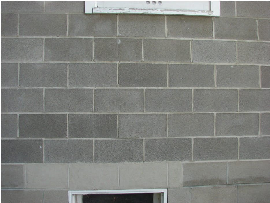
Photograph 14: Residence north elevation – Basement and main floor concrete block step cracking, typical.
