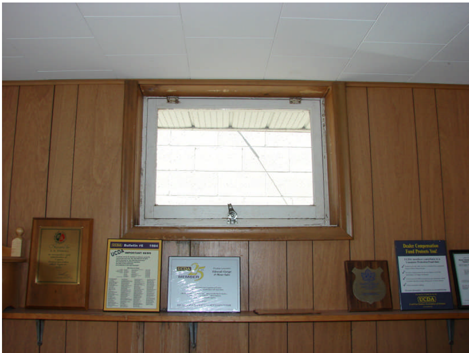
Photograph 54: Residence main floor level – moisture staining at window at west wall at office.
