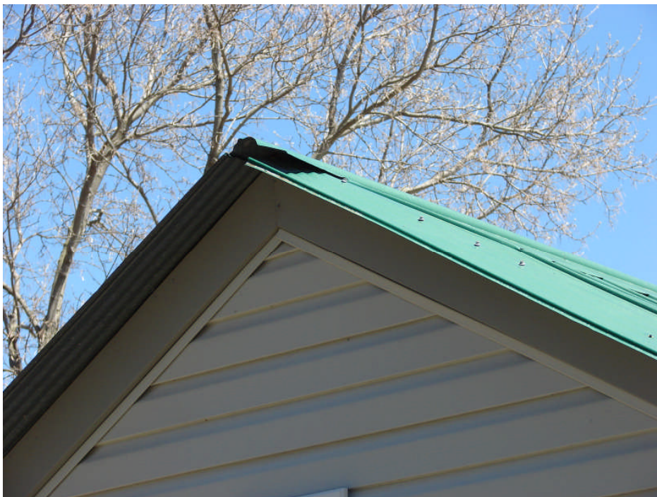
Photograph 4: Other Structures Storage Building - roof ridge missing end cap at west end, typical.
