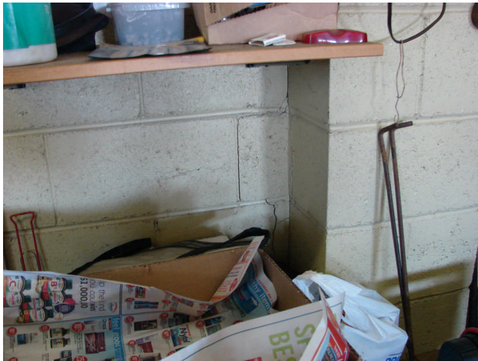
Photograph 39: Garage Building north wall – concrete block wall step cracking near west concrete block pier, typical.
