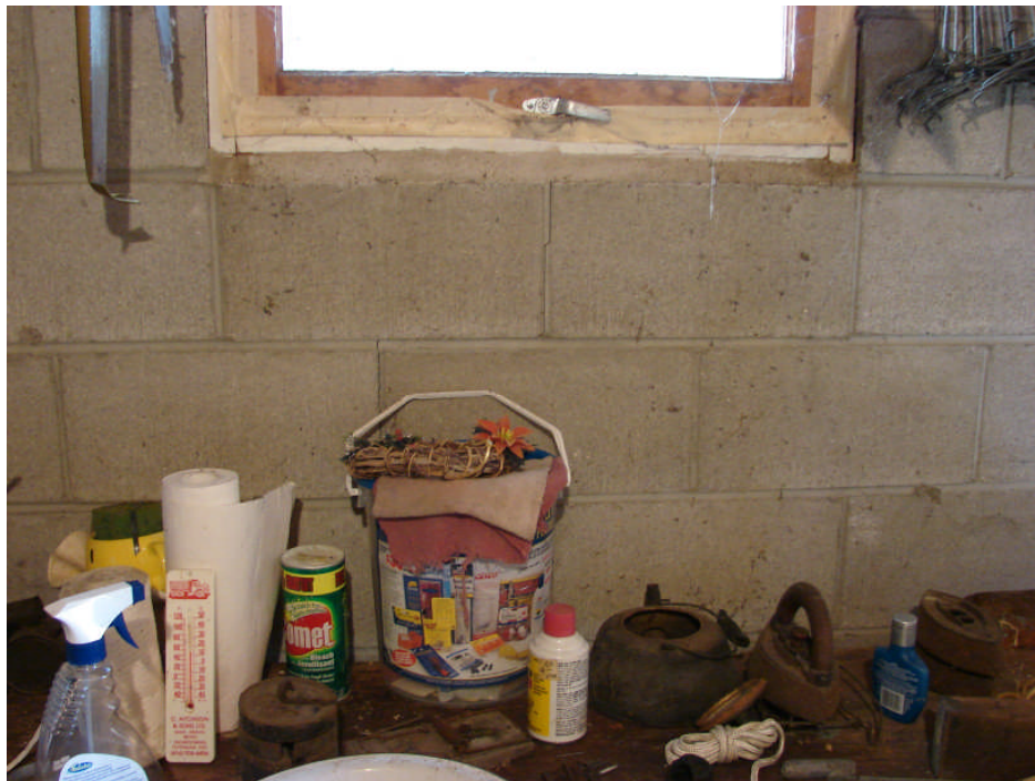
Photograph 28: Residence basement level north wall – concrete block step cracking and taped window perimeter, typical.
