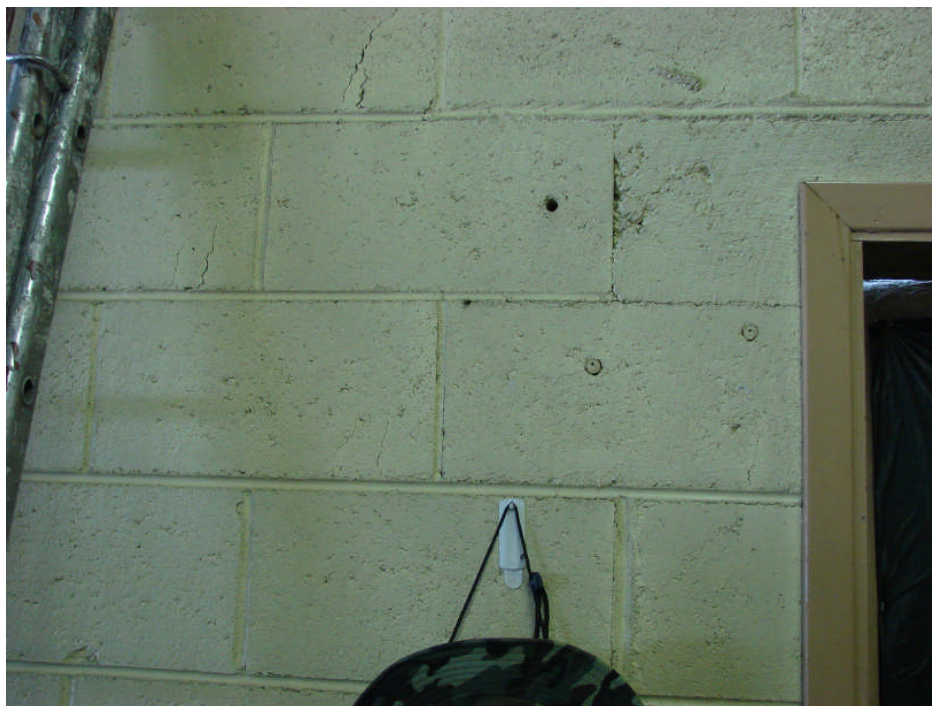
Photograph 51: Garage Building west wall – concrete block wall step cracking at door near north end, typical.
