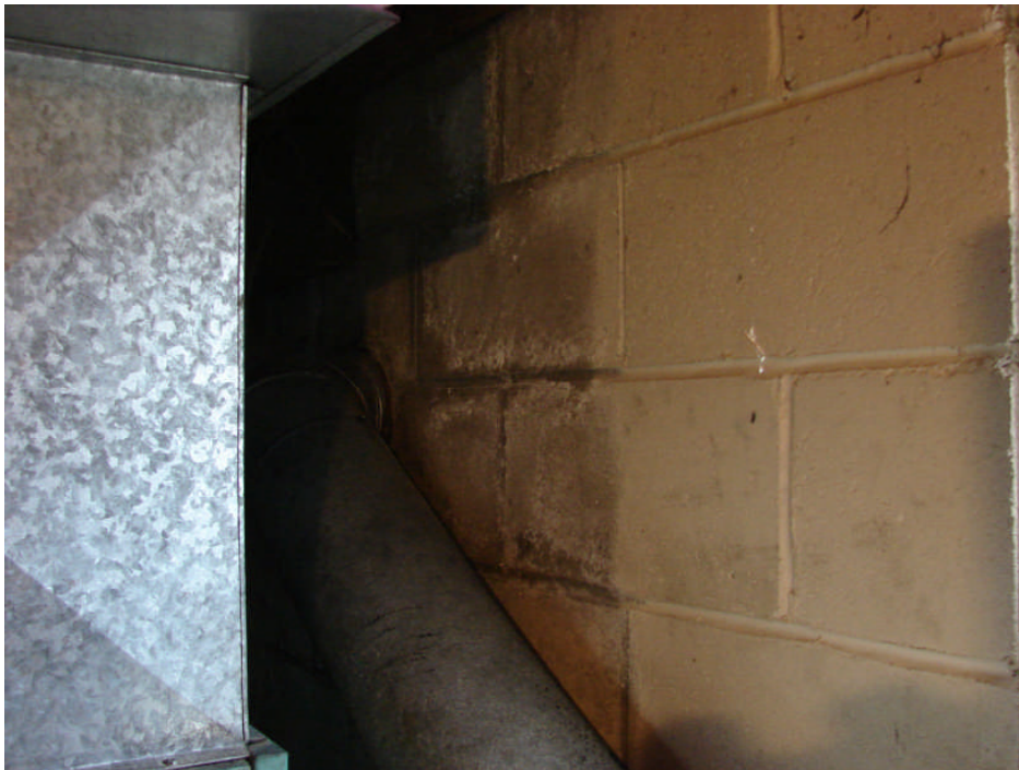
Photograph 34: Residence basement level east wall – moisture staining and efflorescence behind heating system.
