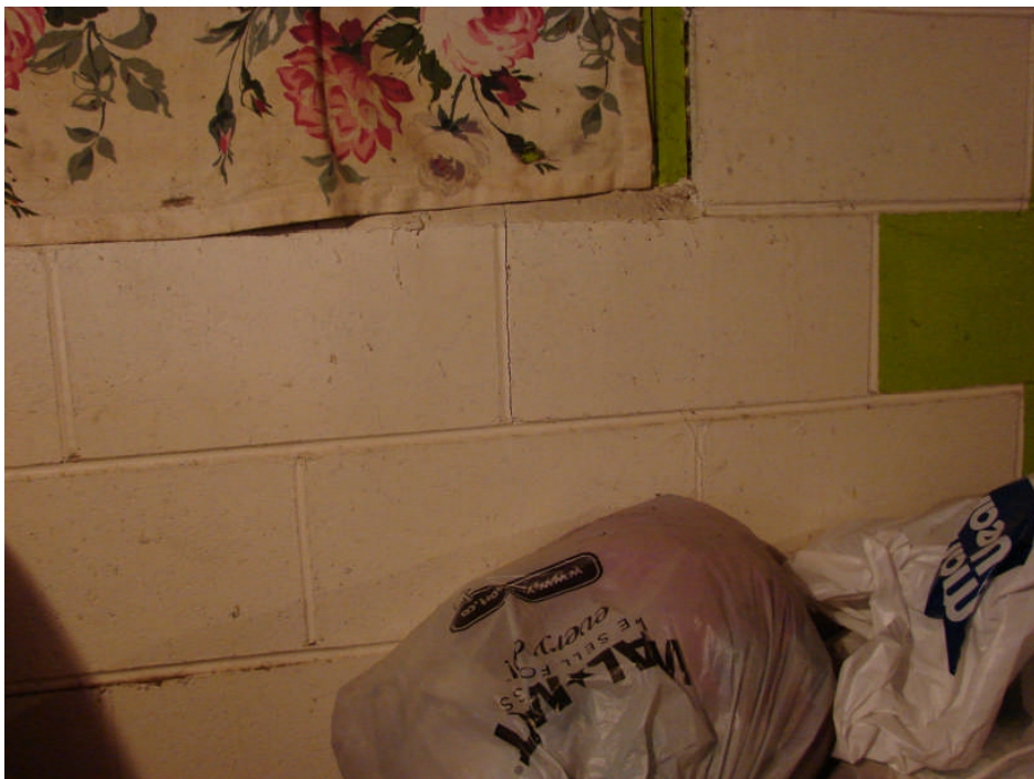
Photograph 36: Residence basement level east wall – concrete block wall step cracking under south window, typical.
