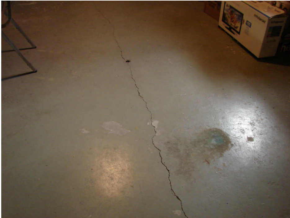
Photograph 45: Residence basement level – painted concrete slab-on-grade cracks, typical.
