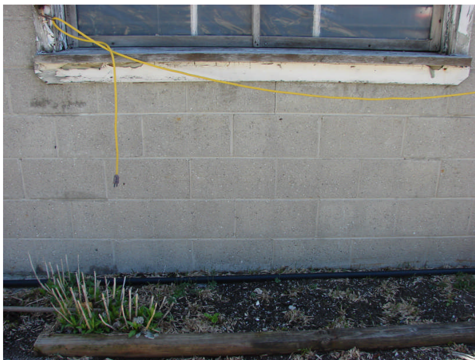
Photograph 13: Garage Building west elevation – concrete block wall step cracking below south window, typical.
