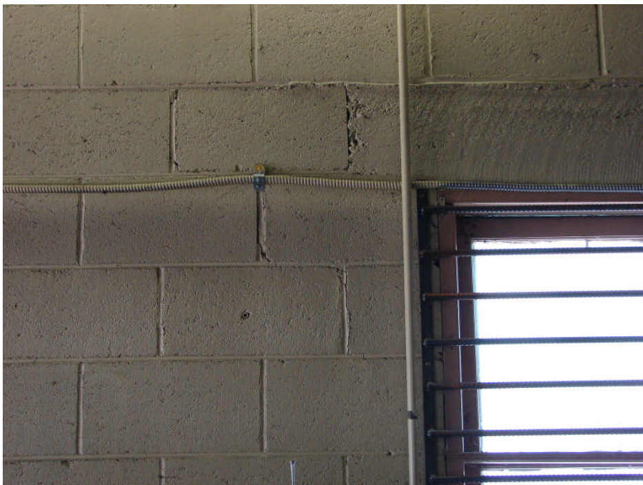
Photograph 50: Garage Building west wall – concrete block wall step cracking at south end of north window, typical.
