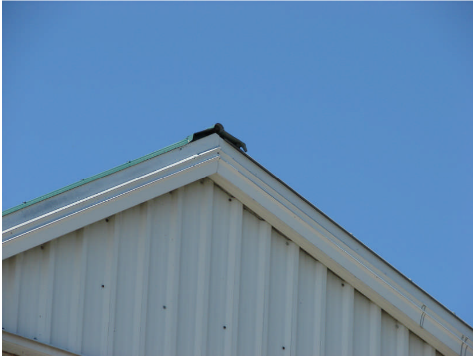
Photograph 29: Garage Building west elevation – missing ridge end cover at east side of metal roof, typical.
