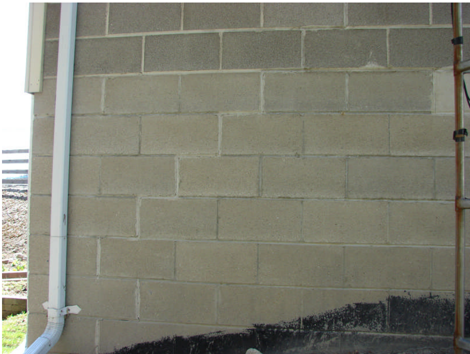
Photograph 18: Residence north elevation – repaired wall step cracks at east end.
