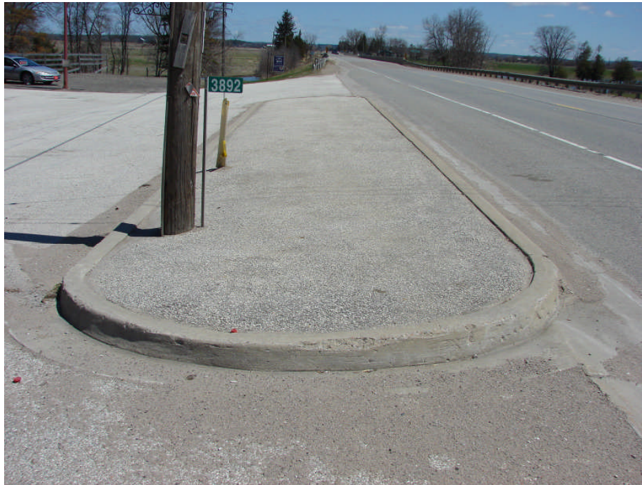
Photograph 31: Site Works – cracking of concrete curb including scuff marks and impact damage at boulevard island, typical.
