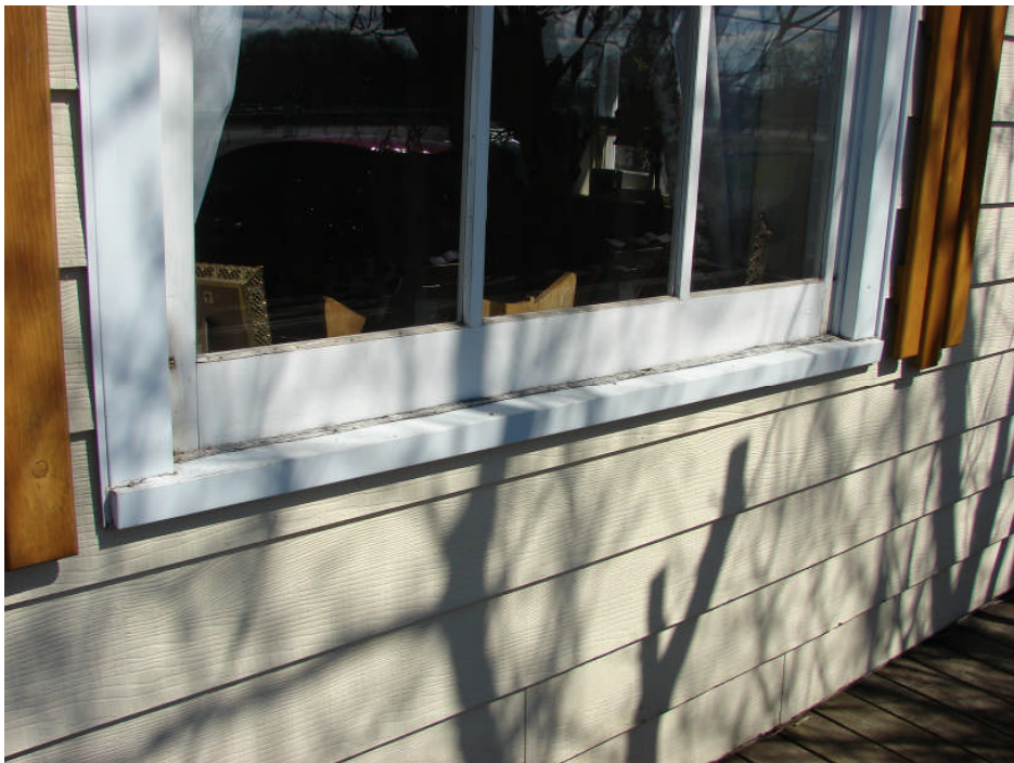
Photograph 6: Residence south elevation – Aged and weather worn paint with peeling/blistering at wooden windows, typical.
