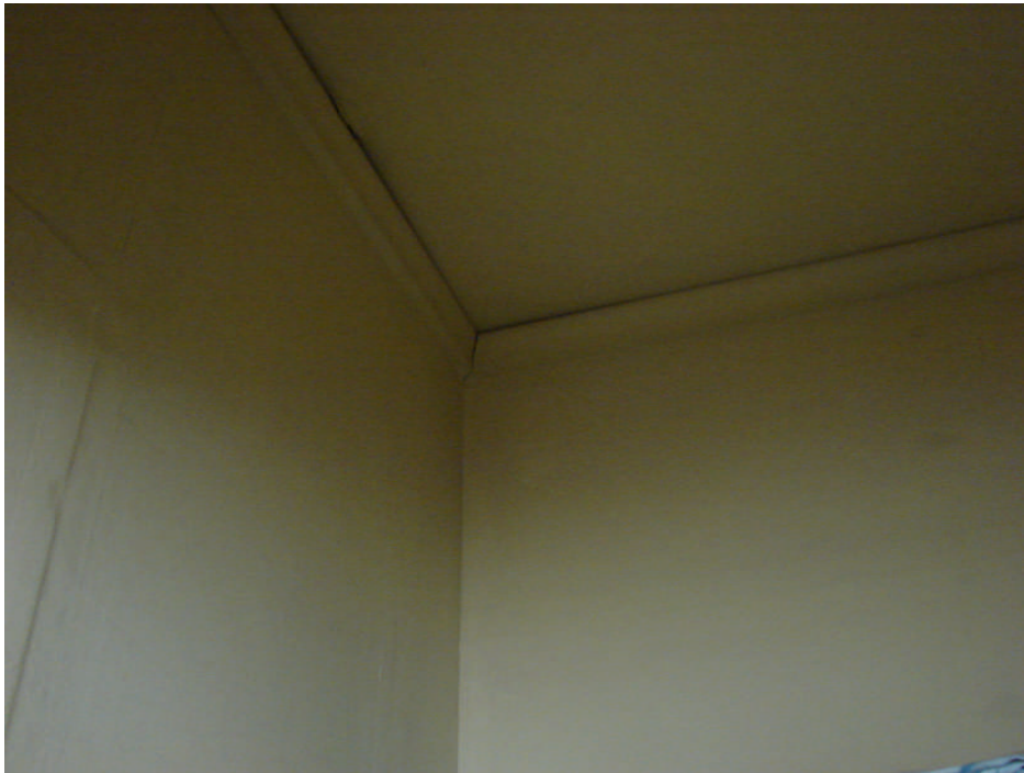
Photograph 48: Residence main floor level – moulding joint cracks at northeast corner of northwest bedroom, typical.
