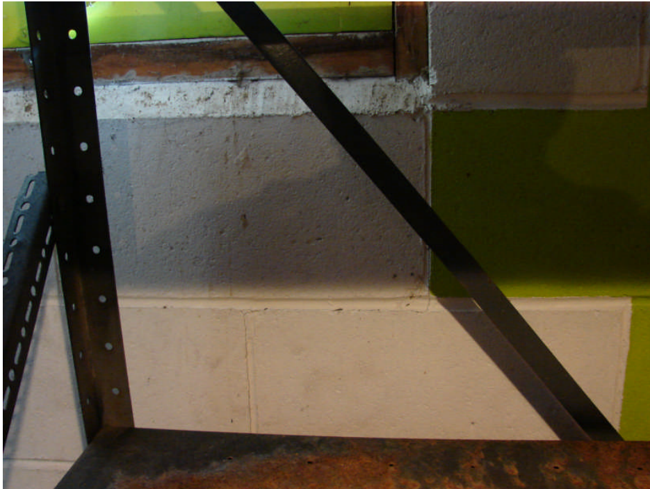
Photograph 35: Residence basement level east wall – concrete block wall step cracking under north window, typical.
