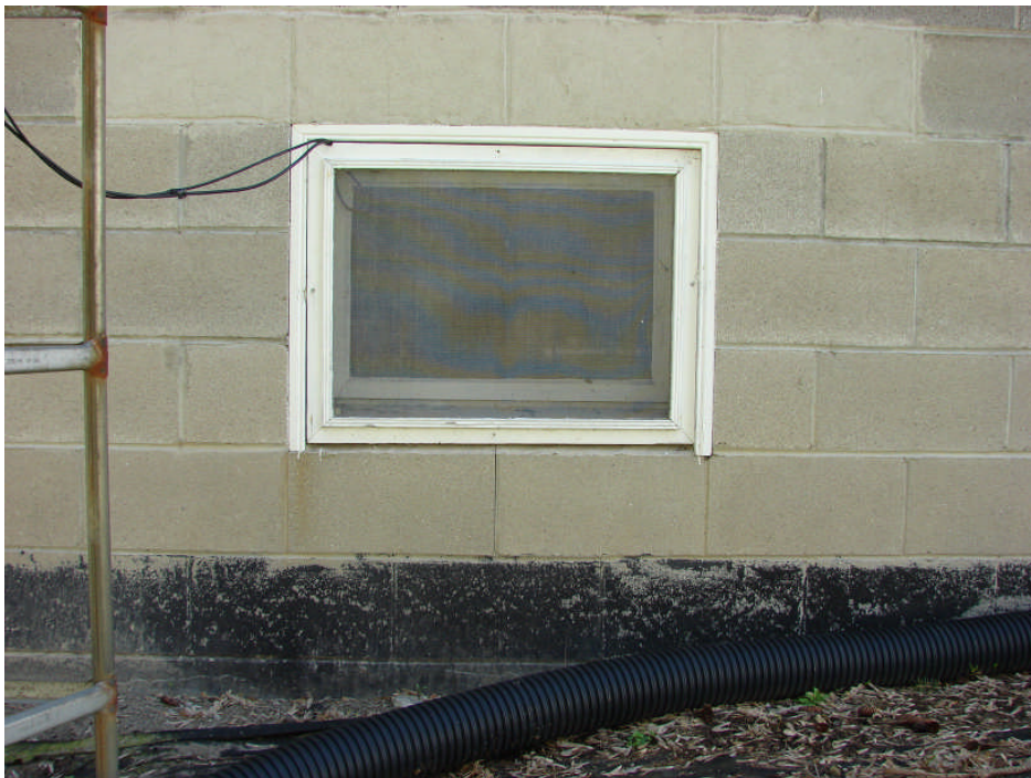
Photograph 16: Residence north elevation – Basement window paint peeling/blistering, also repaired window lintel and wall cracks near east end, typical.
