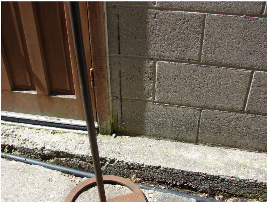
Photograph 30: Garage Building east elevation (south part) – concrete block wall step cracking near door, typical.
