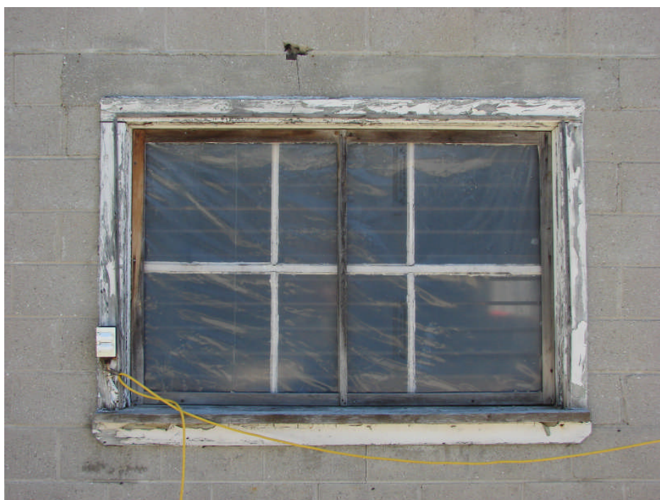
Photograph 18: Garage Building west elevation – windows paint aged and deteriorated with extensive peel/blistering, typical.
