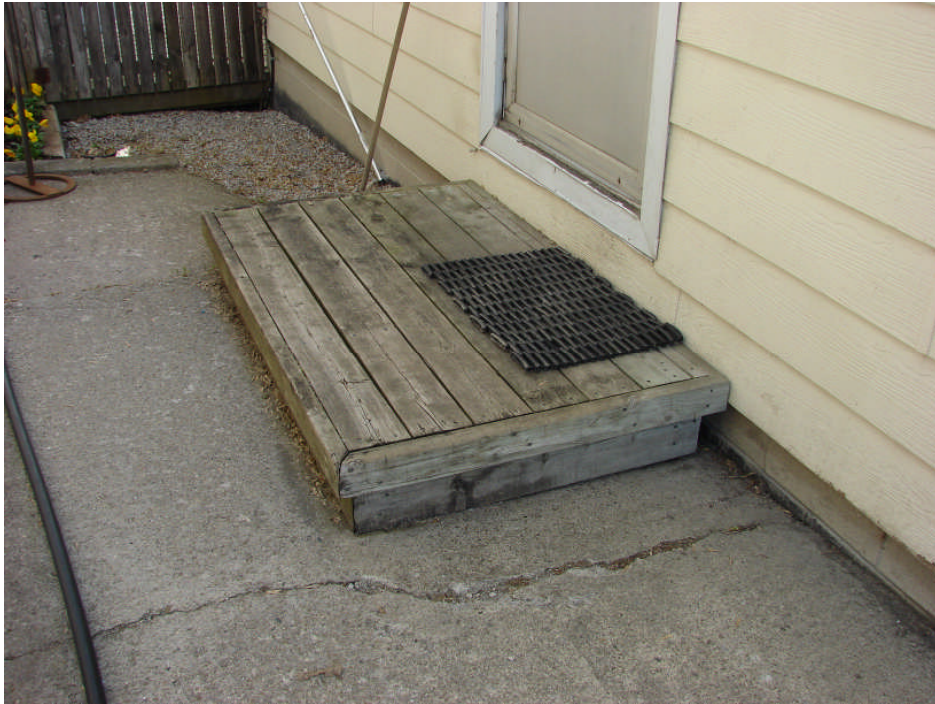
Photograph 11: Residence west elevation – Aged and weather worn wood platform & cracked slab-on-grade concrete with surface spalling, typical.
