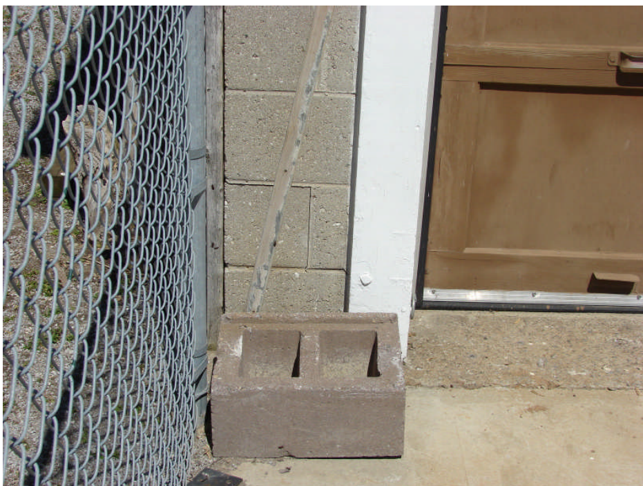
Photograph 4: Garage Building south elevation – concrete block wall step cracking at west end adjacent overhead door, typical.
