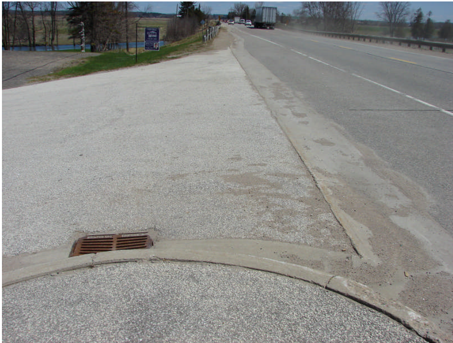
Photograph 33: Site Works – cracking of concrete curb including scuff marks and impact damage at boulevard island, typical.
