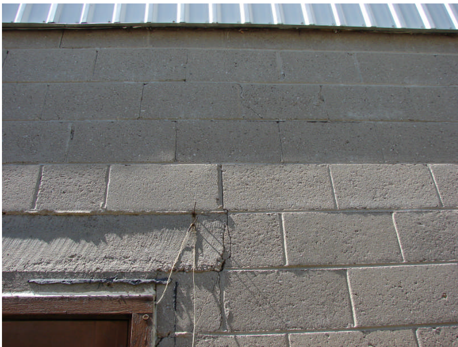
Photograph 32: Garage Building east elevation (south part) – concrete block wall step cracking at door lintel, typical.
