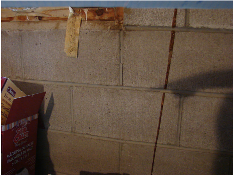
Photograph 29: Residence basement level north wall – concrete block step cracking west window, typical.
