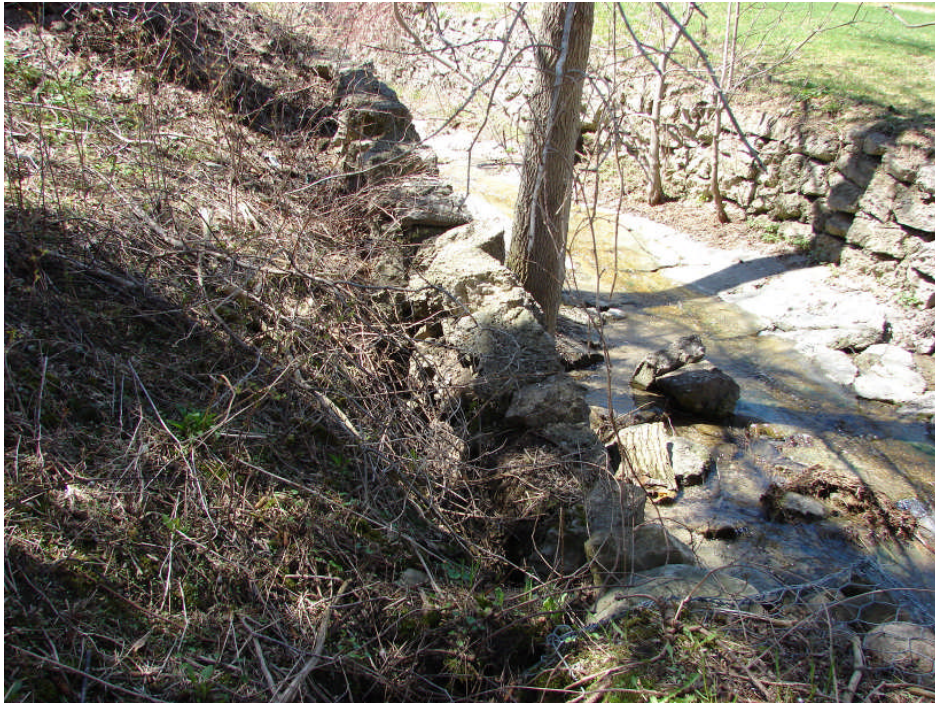
Photograph 15: Site Works – general view along south side of drainage ditch near residence looking west, with extensive soil erosion, typical.
