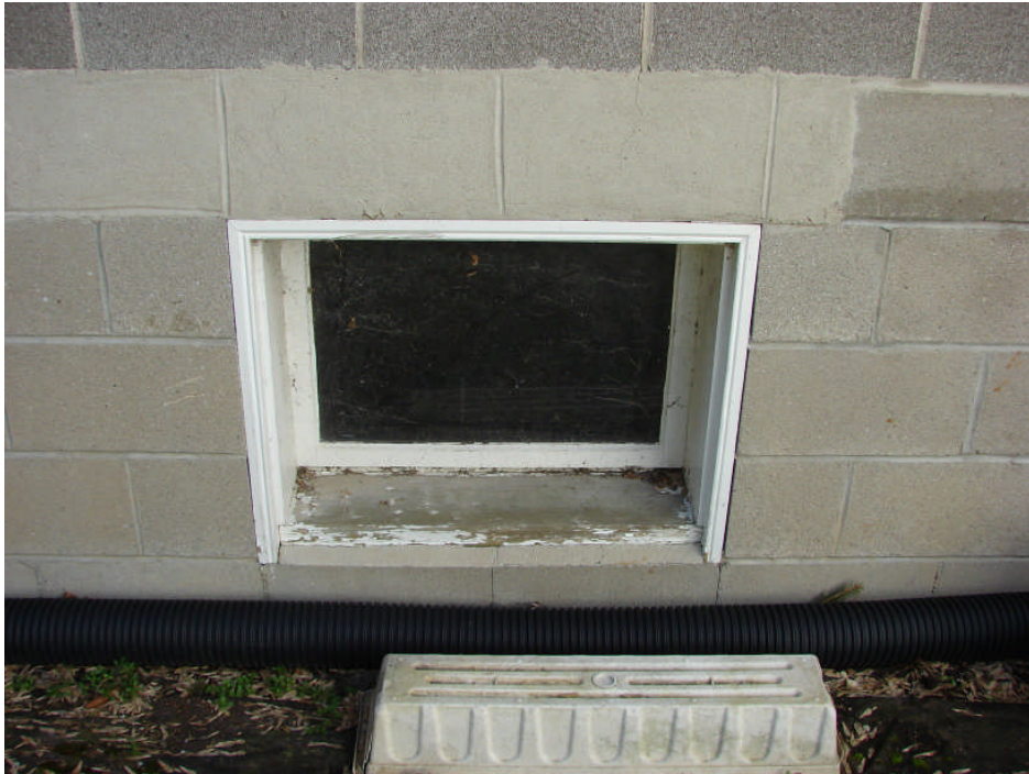
Photograph 13: Residence north elevation – Basement window paint peeling/blistering, also repaired window lintel and wall cracks near west end, typical.
