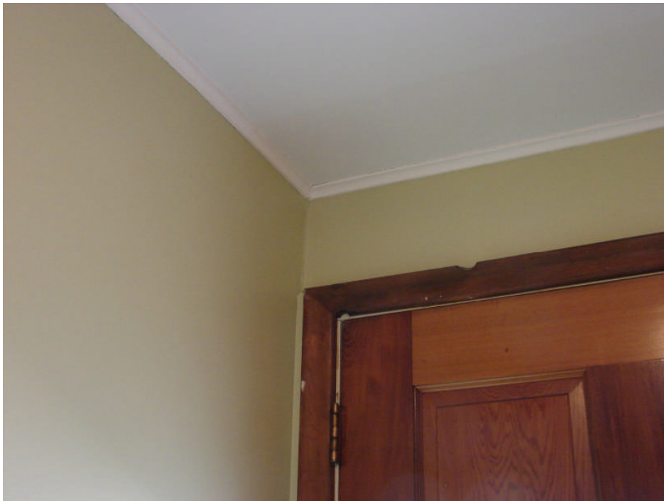
Photograph 46: Residence main floor level – drywall crack above south corner of hallway exterior door.
