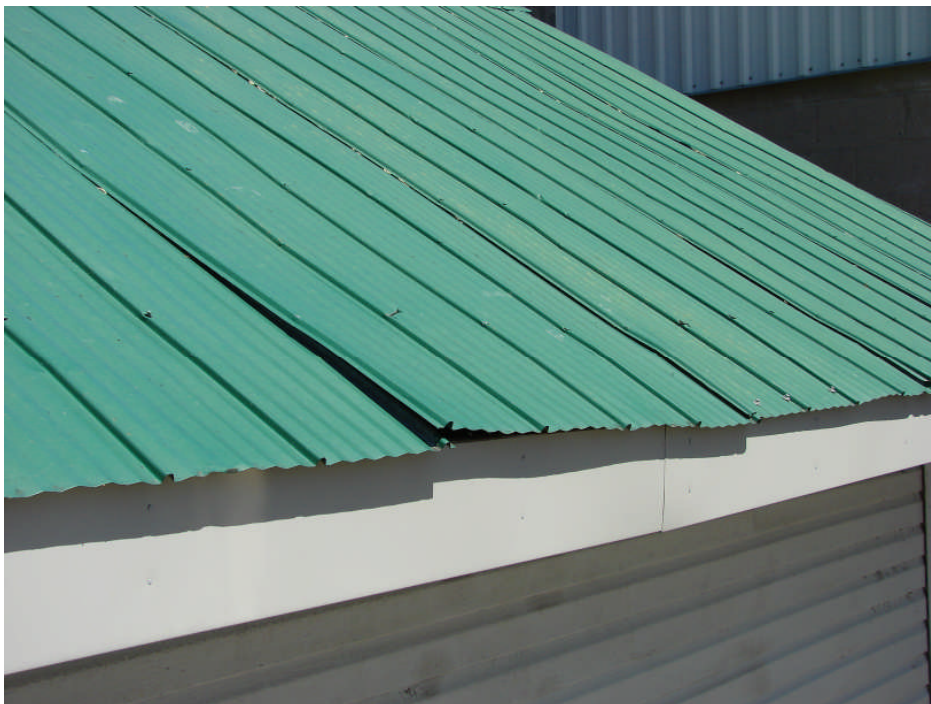
Photograph 6: Other Structures Storage Building – loose metal roof panels missing fasteners, typical.
