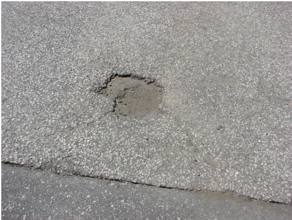
Photograph 26: Site Works – hole in the asphalt pavement and cracking near the large asphalt patch/repair.
