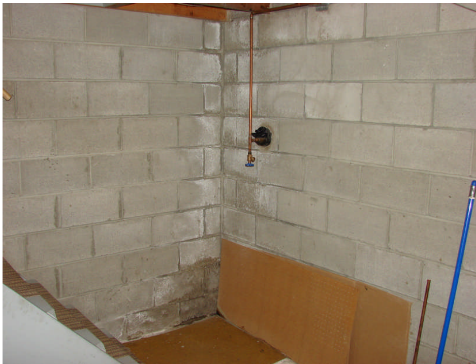
Photograph 26: Residence basement level north wall – moisture stain and efflorescence at the concrete block wall at west corner.
