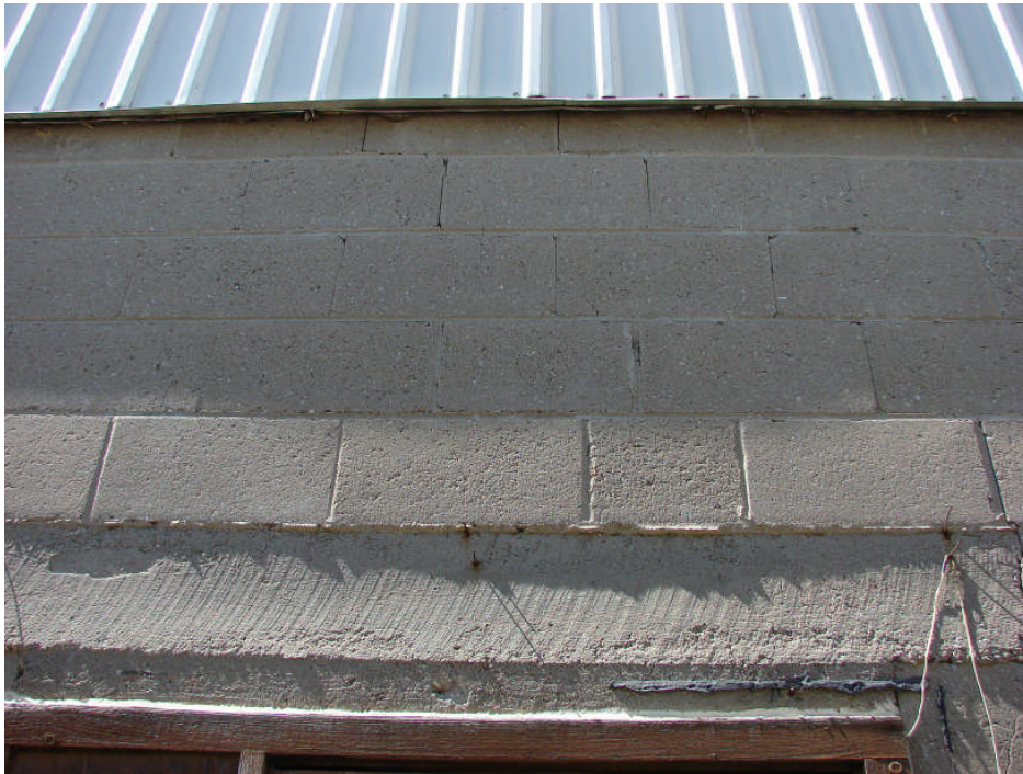
Photograph 33: Garage Building east elevation (south part) – concrete block wall step cracking above door, typical.
