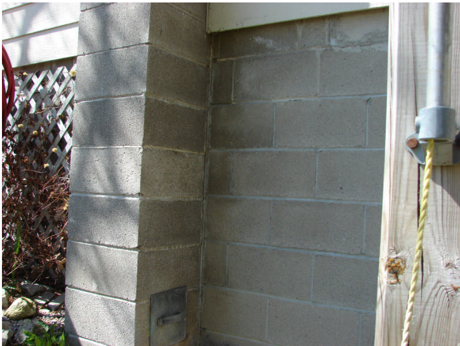
Photograph 22: Residence east elevation – concrete block wall joint cracking at chimney at basement level, typical.
