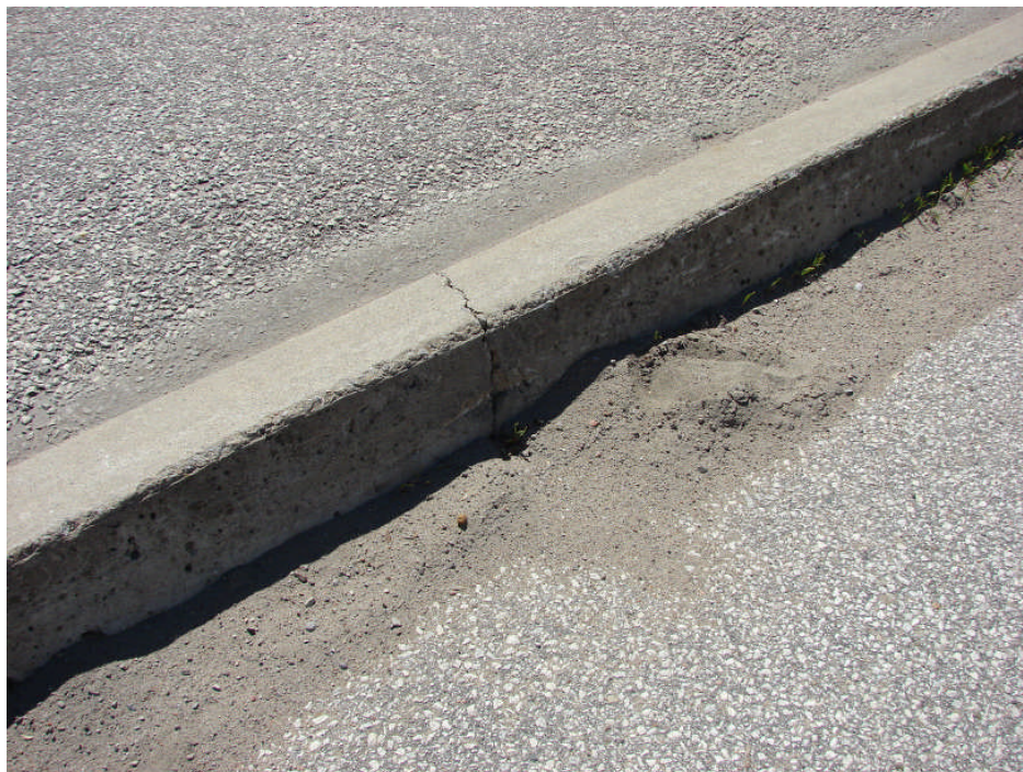
Photograph 32: Site Works – cracking of concrete curb including scuff marks and impact damage at boulevard island, typical.
