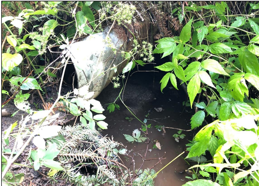
Photo 1. Void under upstream culvert inlet. [July 20, 2021]
