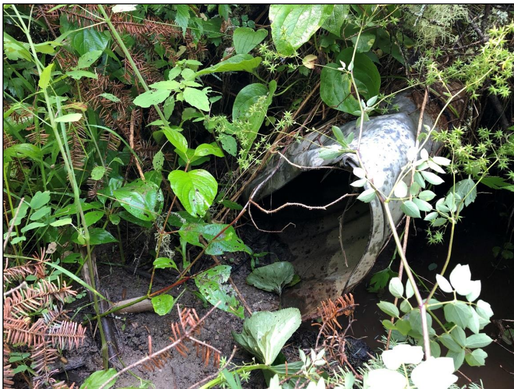
Photo 2. Culvert deformed at inlet. [July 20, 2021]
