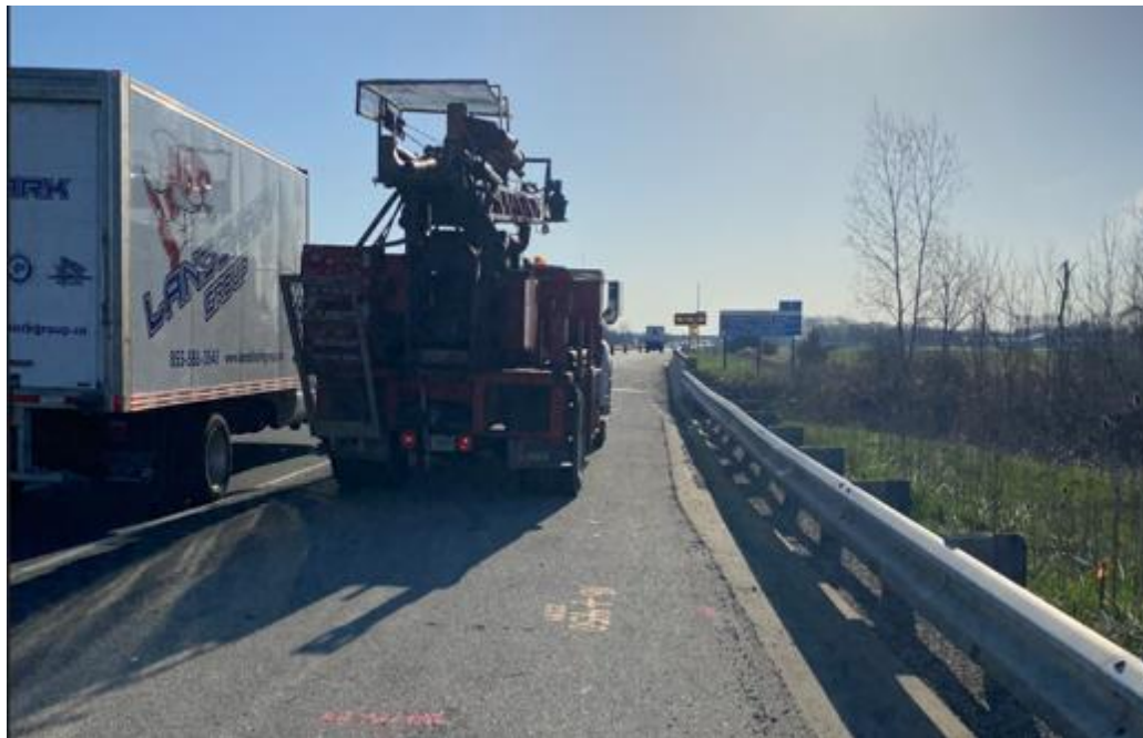
Photo 6: Drilling set up at Borehole, BH15-22 – Highway 402 Eastbound Lane (April 12 th , 2023)
