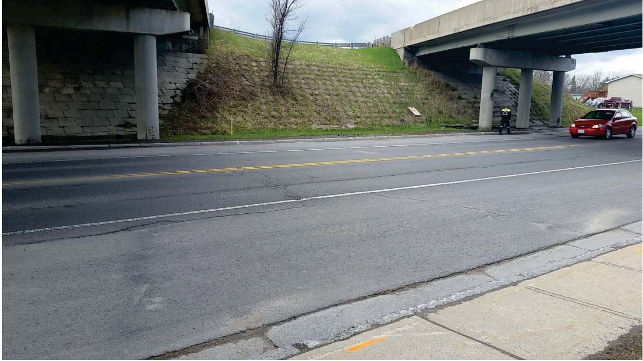
Figure 3: Looking west at existing slope paving between bridges
