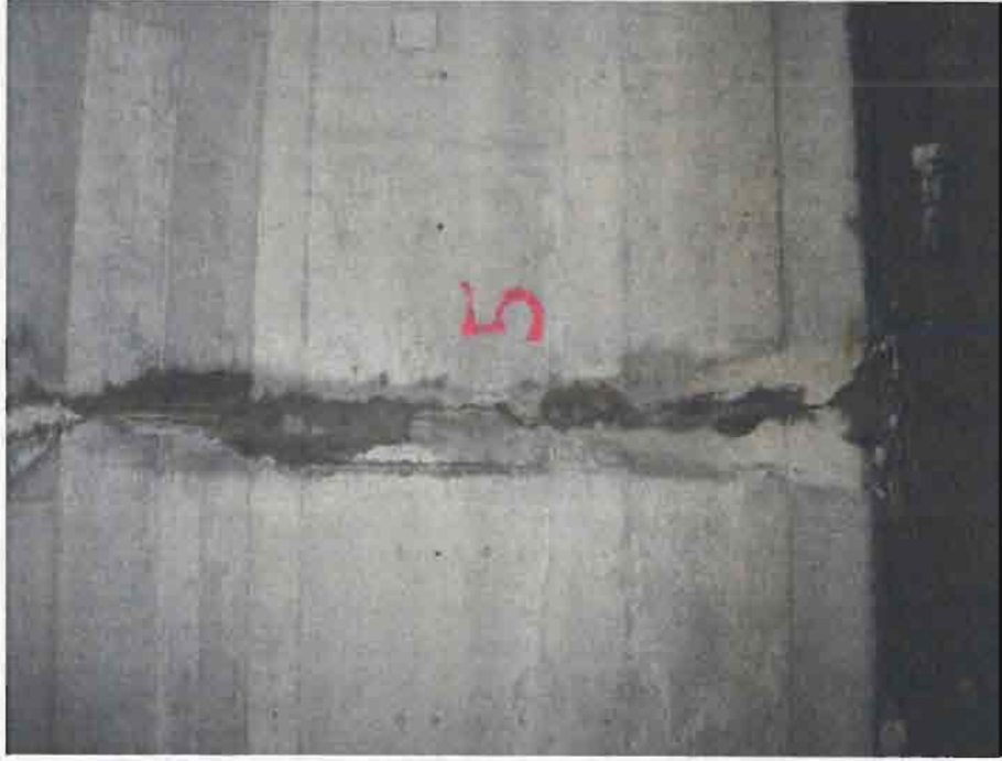
Photo 2: 2-3 millimetre wide crack on wall, 25 metres upstream/west of outlet of Ramp 'D' Chedoke Creek culvert.
