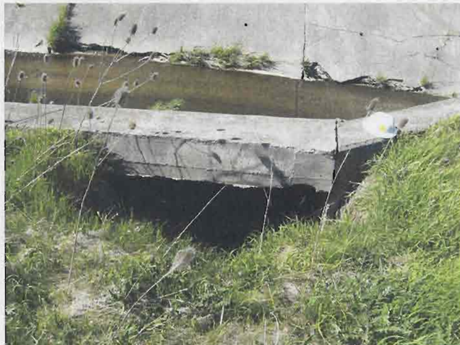
Photo 6: Sinkhole due to erosion/loss of ground just northeast of Ramp 'D' Chedoke Creek culvert.
