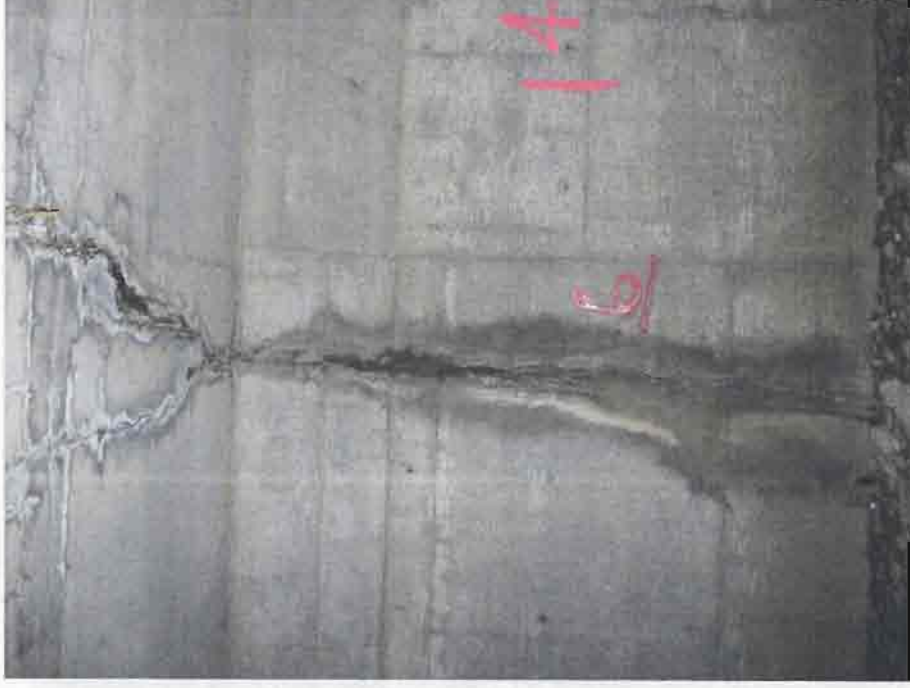
Photo 3: North wall of Ramp 'D' Chedoke Creek culvert approximately 41 metres upstream/west of outlet. Crack is about 10 millimetres wide.
