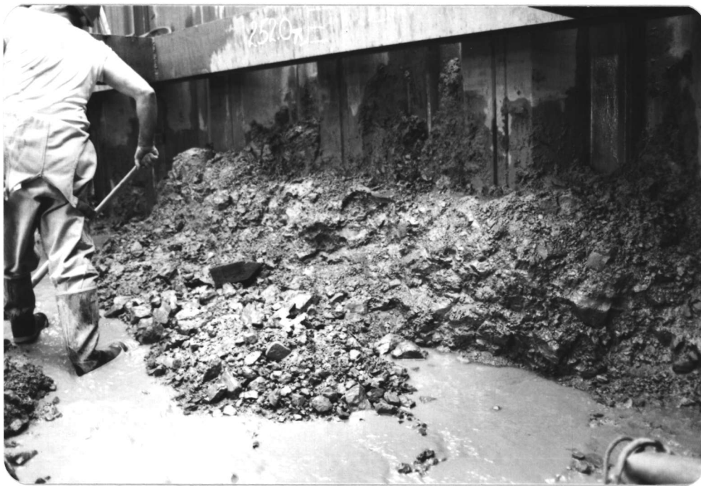
Photo No. 13 - As per Photos, Nos. 11 and 12, showing progressive disintegration after exposure to air.
