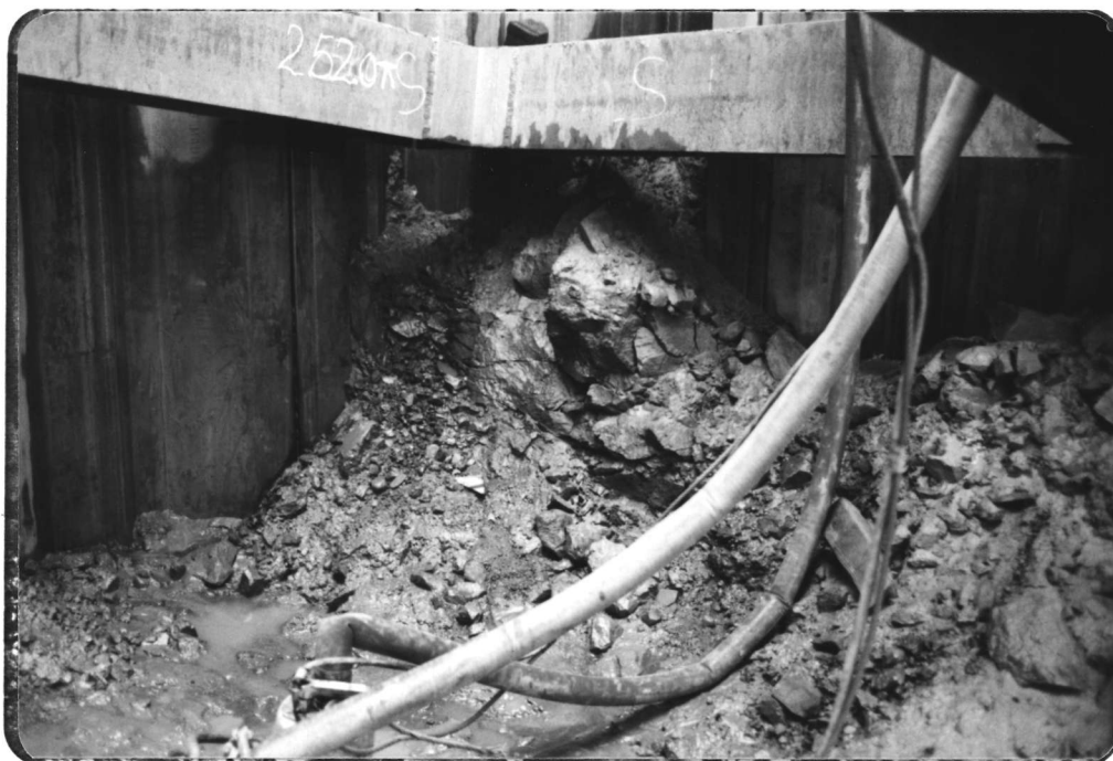
Photo No. 7 - Exposed rock at southeast corner of cell. Base at approximately elevation 248 feet.
