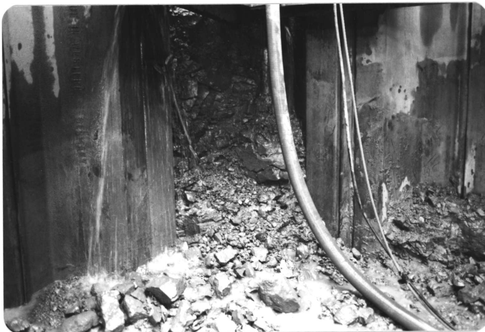
Photo No. 5 - Exposed rock at northeast corner of cell. Base at approximately 248 feet.
