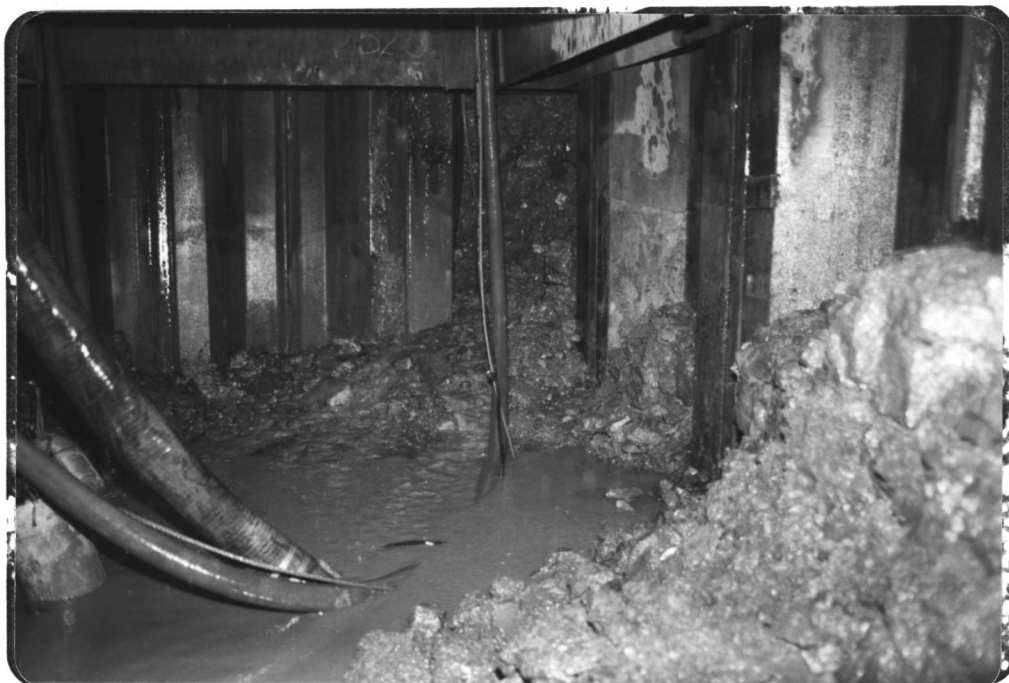
Photo No. 8 - Exposed rock at northeast corner of cell. Base at approximately elevation 248 feet. Rock bench in foreground.
