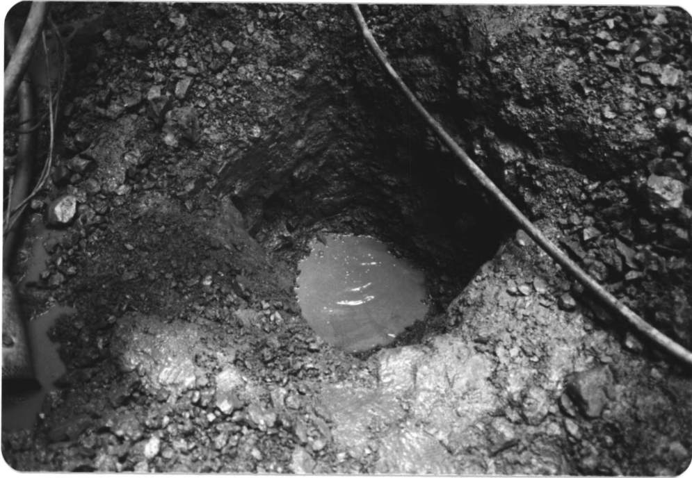
Photo No. 17 - View of test pit excavated to approximately elevation 243 feet.
