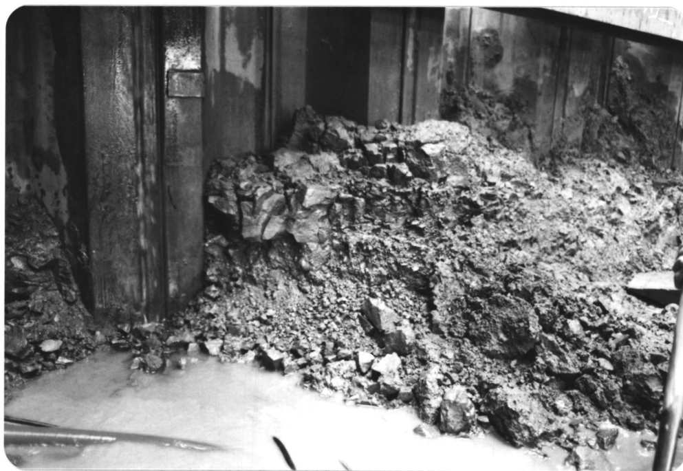
Photo No. 6 - Exposed rock at bench along east wall of cell. Top at approximately elevation 250 feet.
