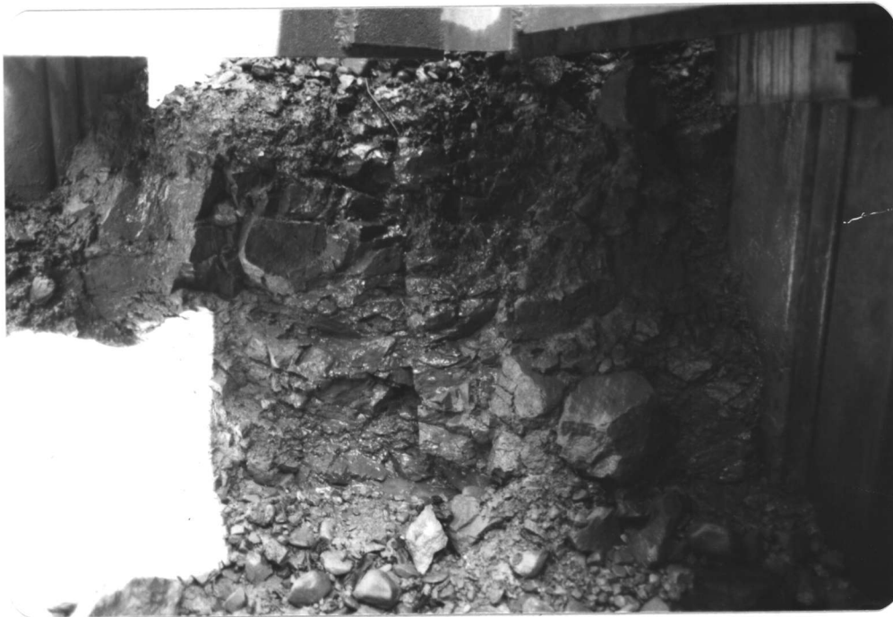
Photo No. 3 - Exposed rock northwest corner of cell. Base at approximate elevation 248 feet.
