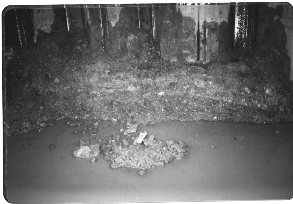
Photo No. 11 - Rock bench along east wall of cell shortly after dewatering. Top at approximately elevation 250 feet.
