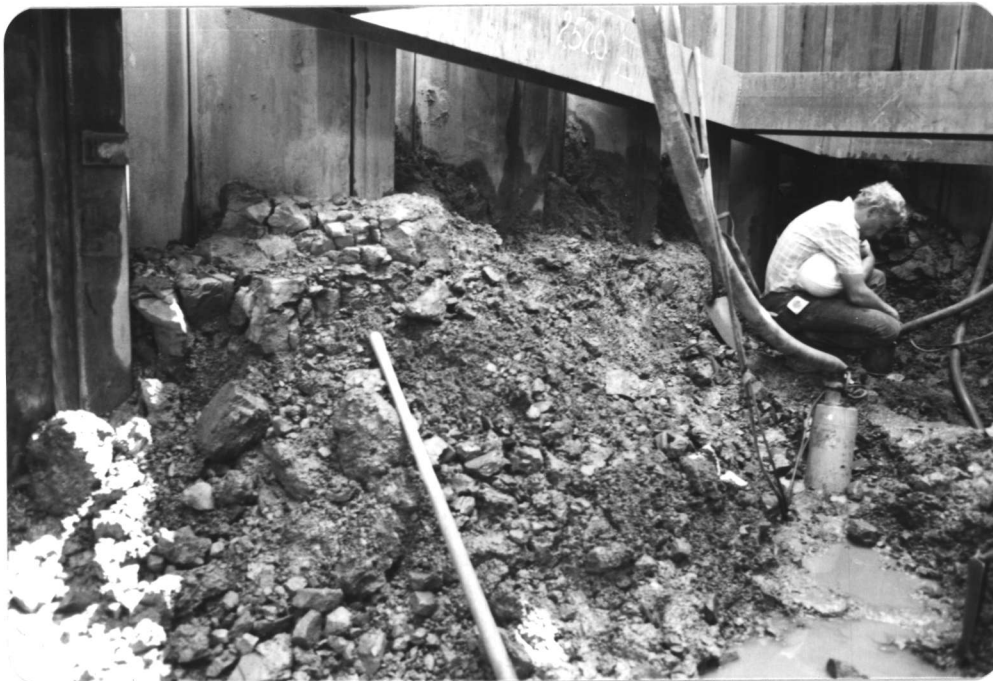
Photo No. 14 - As Photos, Nos. 11, 12 & 13, showing progressive disintegration after exposure to air.
