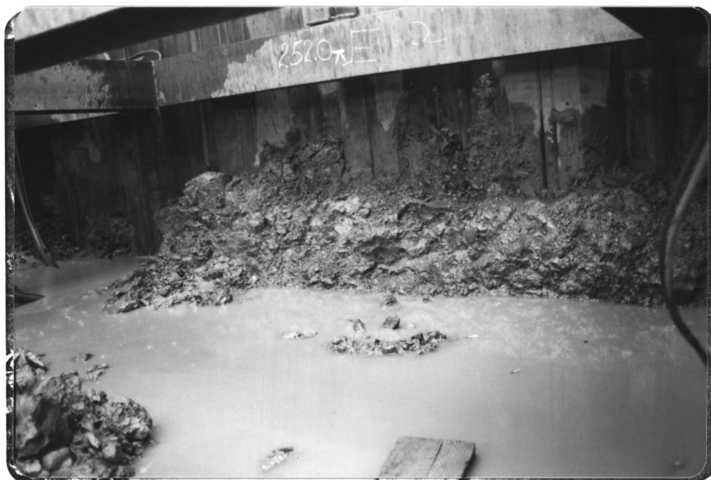
Photo No. 12 - As per Photo No. 11 showing disintegration after several hours exposure to air.
