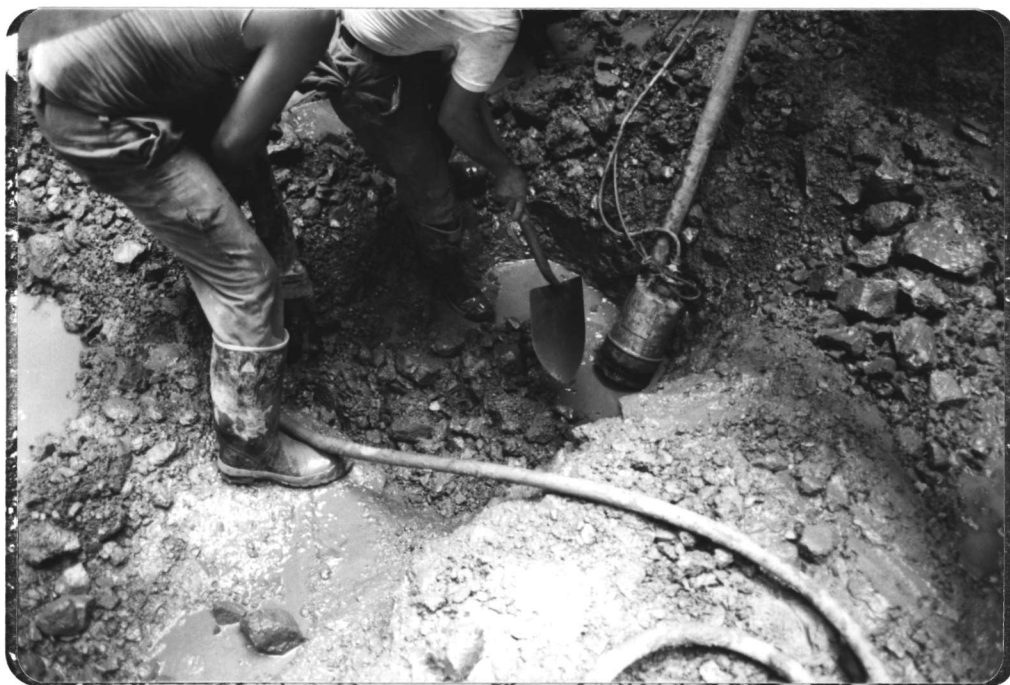
Photo No. 16 - Test pit being excavated by mechanical spade and hand shovelling.
