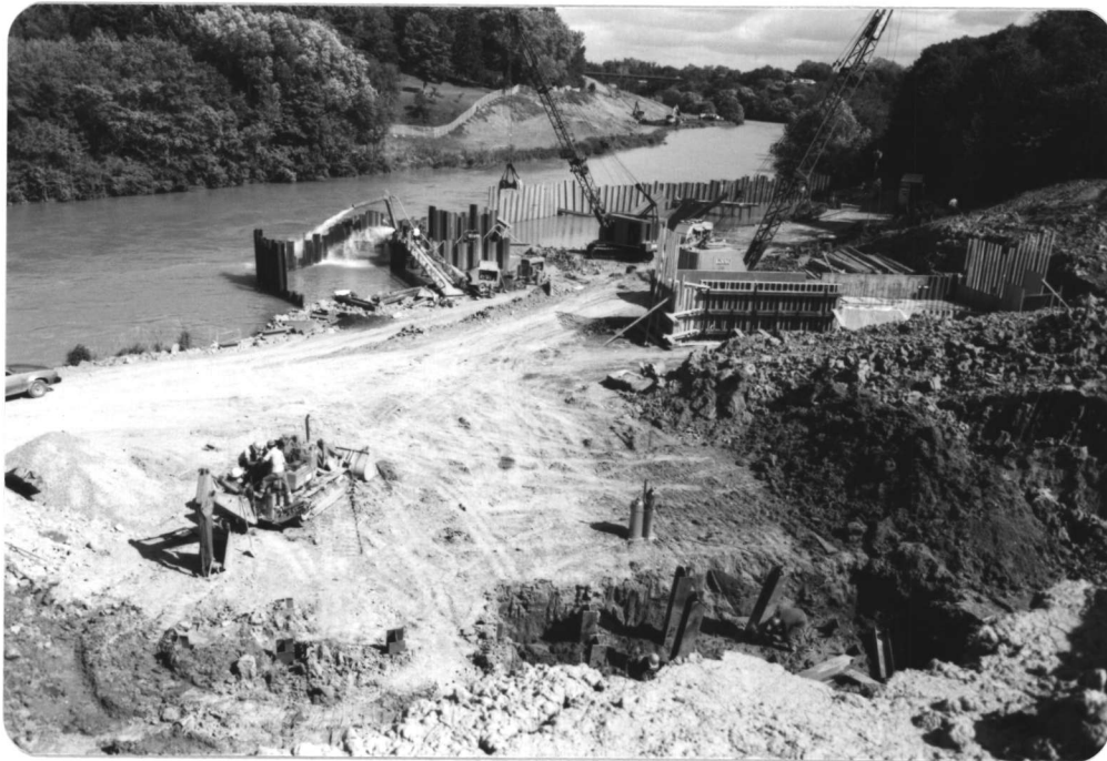
Photo No. 1 - General view of site looking upstream to the south. Cellular cofferdam (cell) inside diversion is at Pier No. 2 of northbound lane.
