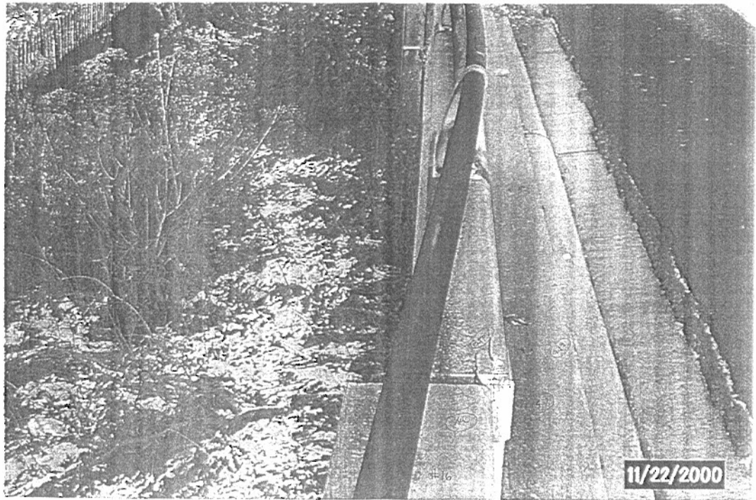
Photo 1: Displacement of Panel 16 during year 2000
